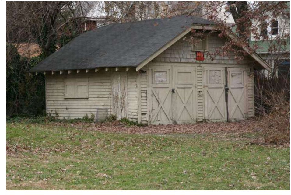
Photograph 4: Southwest (side) and southeast (front) elevations of the garage at 78 E. Centre Street. Looking north (November 2018).
