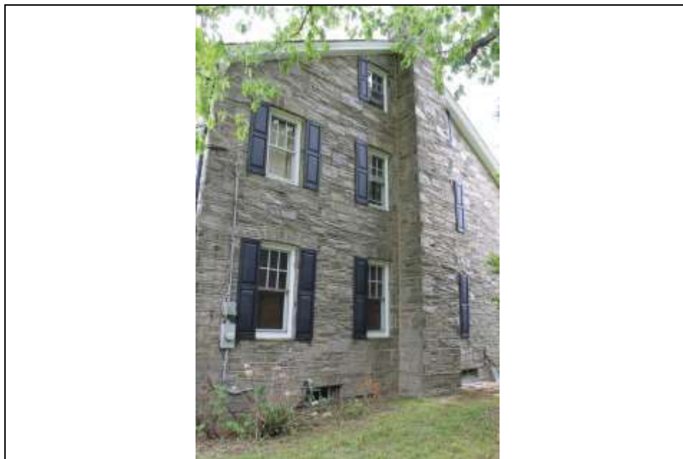
Photograph 4: Northwest (side) elevation of dwelling at 856 Main Street. Looking south (May 2014).
