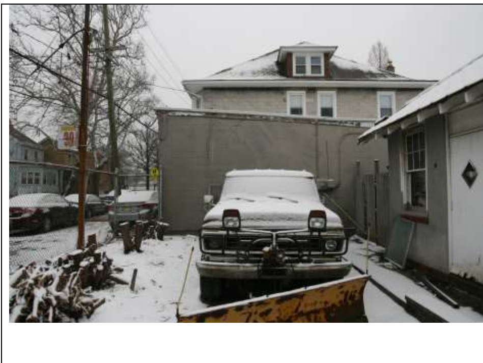
Photograph 11: North portion of northwest (side) elevation of the Garage/Workshop; note the concrete block construction. The façade of the gas station is visible on the right. Looking east (January 2019).
