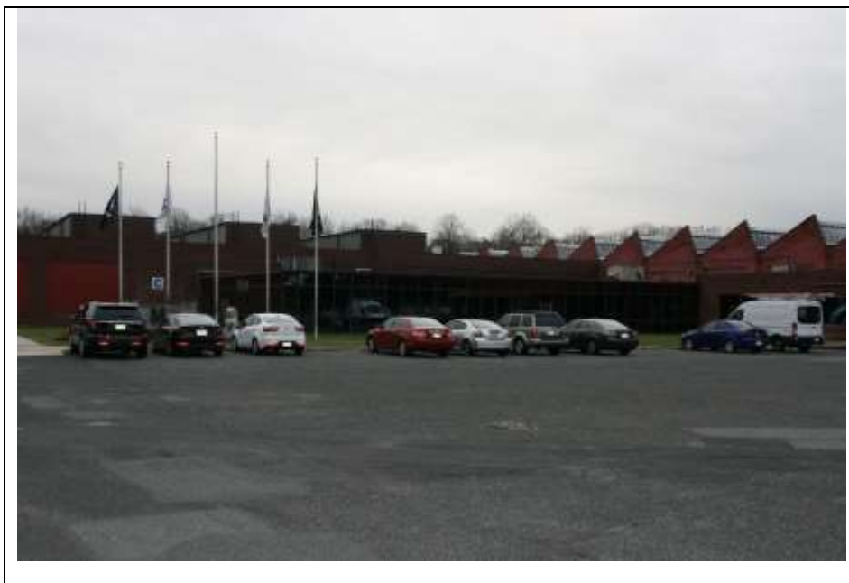
Photograph 24: Overview of the circa -1967 office (Unit C). The sawtooth roof of the 1918 manufacturing plant and storehouse is visible at right-background, and the monitor roof of Unit F is visible at left-background. Looking west (November 2018).
