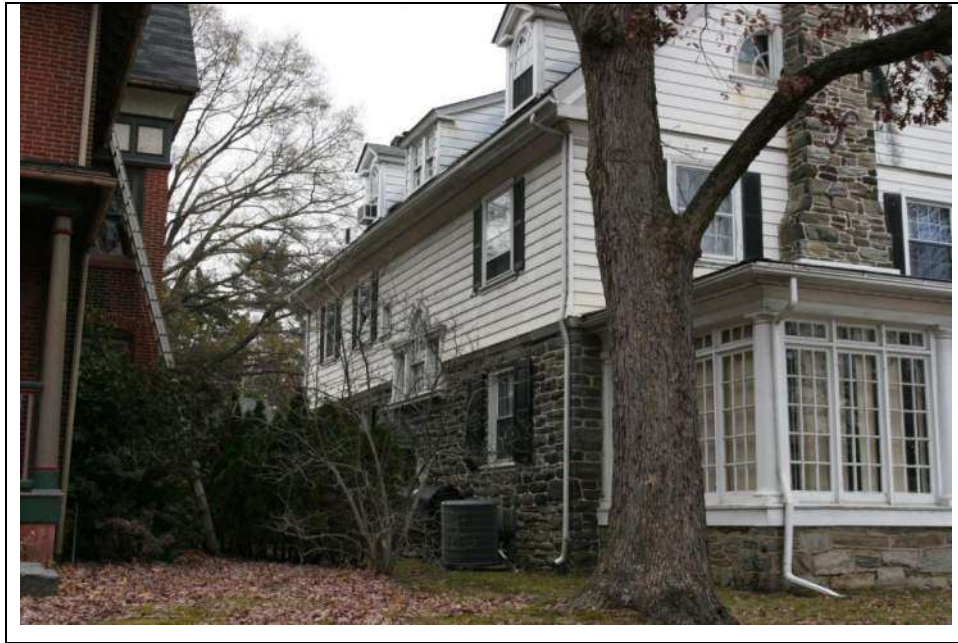
Photograph 4: South (side) and west (rear) elevations of dwelling at 7 N. Evergreen Avenue. Looking northeast (November 2018).
