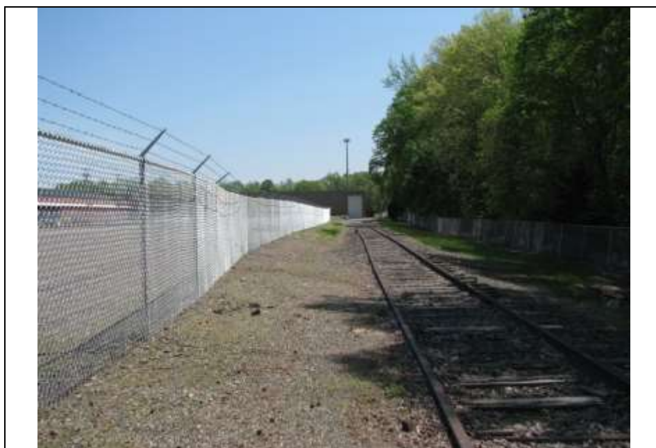
Photograph 32: Partially buried circa -1953 railroad siding located just inside the southwest property line. It appears that this line, which extended from the West Jersey Railroad's Bridgeton Branch, was installed to serve Unit K (ca. 1953), as it is aligned with an opening in the building's northwest elevation (visible at right background). Looking southeast (May 2014).
