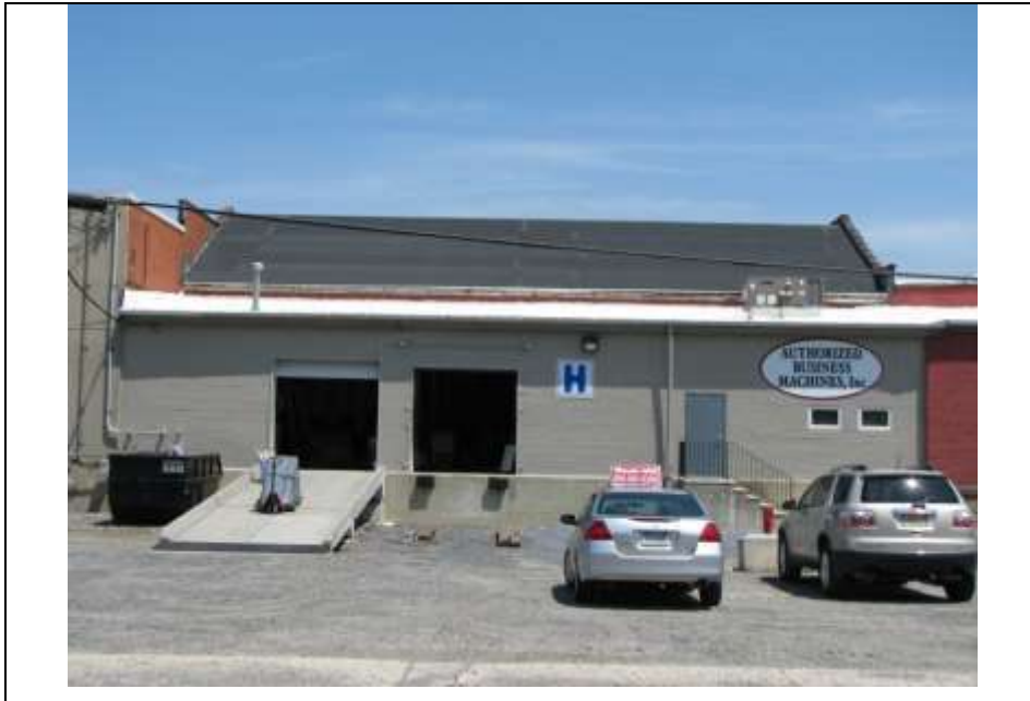
Photograph 12: Southwest elevation of the 1918 wooden box shop (Unit H). Note the modern doors and windows. Looking northeast (May 2014).
