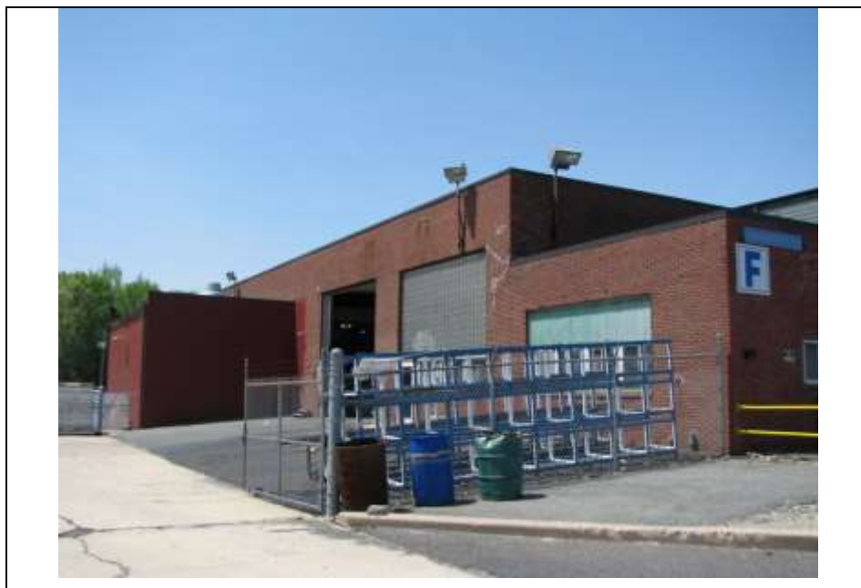
Photograph 16: Southeast elevations of the 1948 Unit F. Looking southwest (May 2014).
