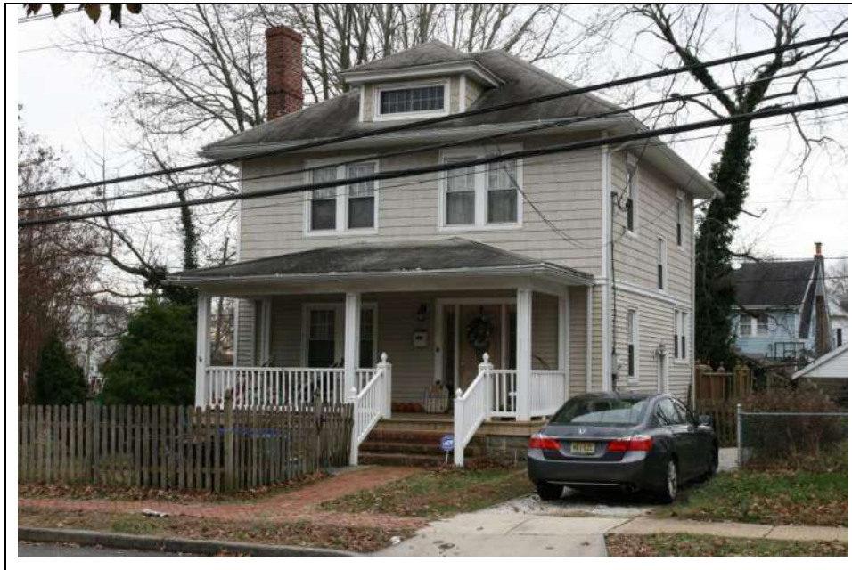
Photograph 1: Northeast (front) and northwest (side) elevations of dwelling at 77 E. Centre Street. Looking south (November 2018).
