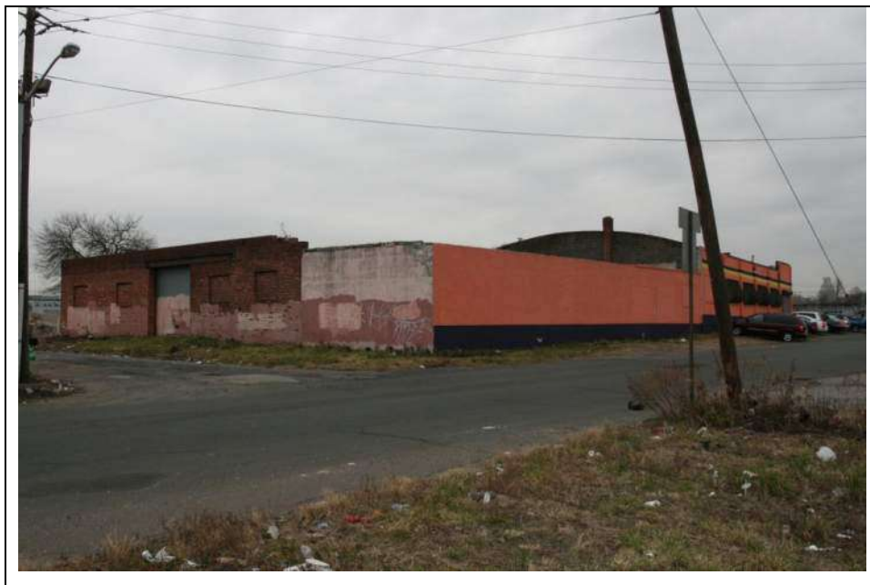
Photograph 5: South (rear) and east (side) elevations of Victory Garage (at far right) and the concrete block and brick wall surrounding the rear portion of the lot. Looking northwest (December 2018).
