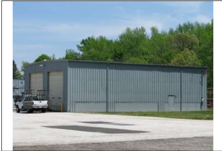
Photograph 30: Northwest (front) and southwest (side) elevations of the circa -1980 garage. Looking northeast (May 2014).
