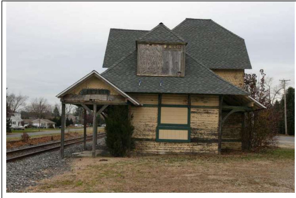
Photograph 6: Southeast (side) elevation of the Sewell Train Station, looking northwest (November 2018).
