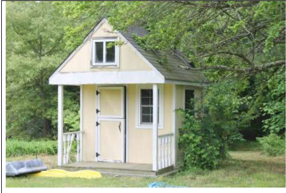
Photograph 8: North and west elevations of modern playhouse at 856 Main Street. Looking southeast (May 2014).
