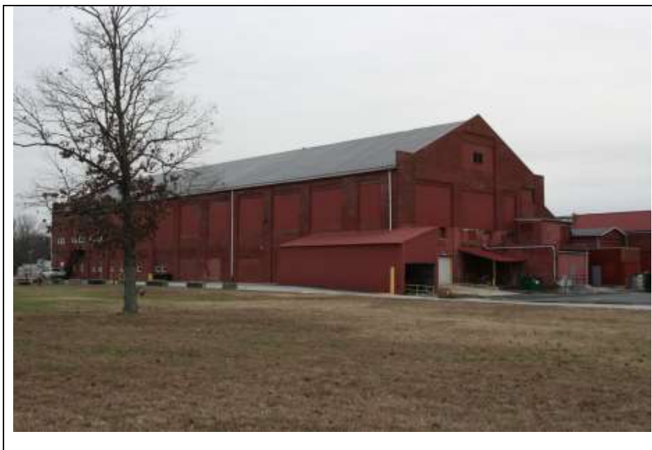
Photograph 2: Overview of the 1918 furnace room (Unit A, at left). The machine shop (Unit E) is just visible at the right. Looking south (November 2018).
