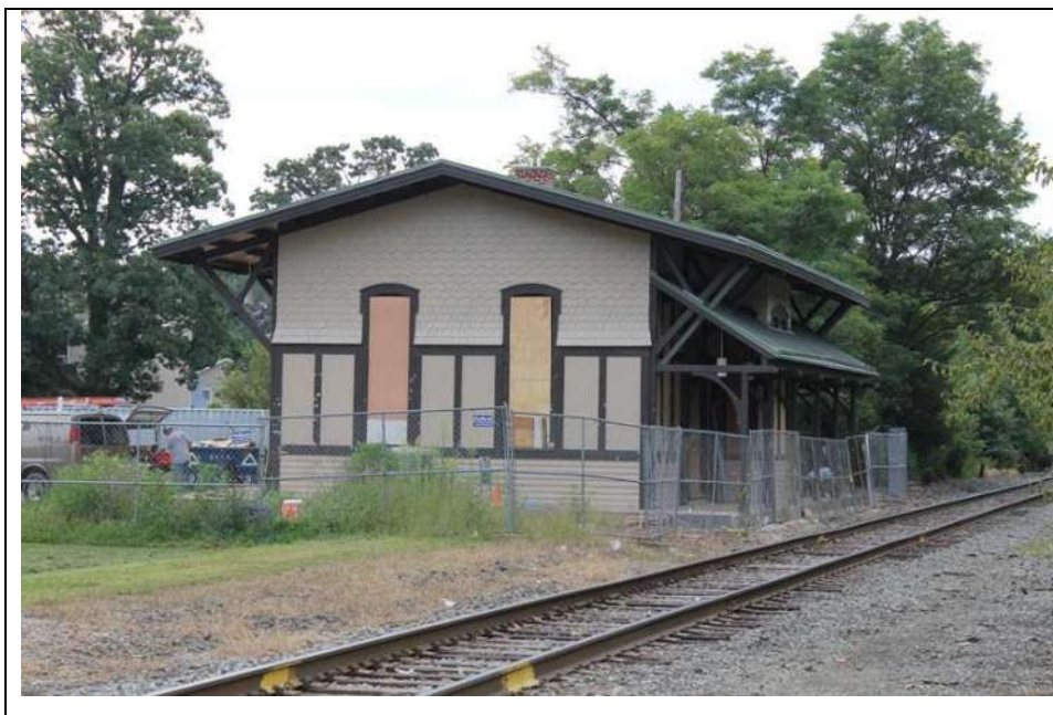
Photograph 9: Glassboro Train Station (ca. 1867, moved to its current location and renovated in 1892), located on Oakwood Avenue, Glassboro Borough, Gloucester County. This former West Jersey Railroad train station exhibits Stick and Italianate stylistic influences. The building was recently restored. Looking southeast (August 2013).
