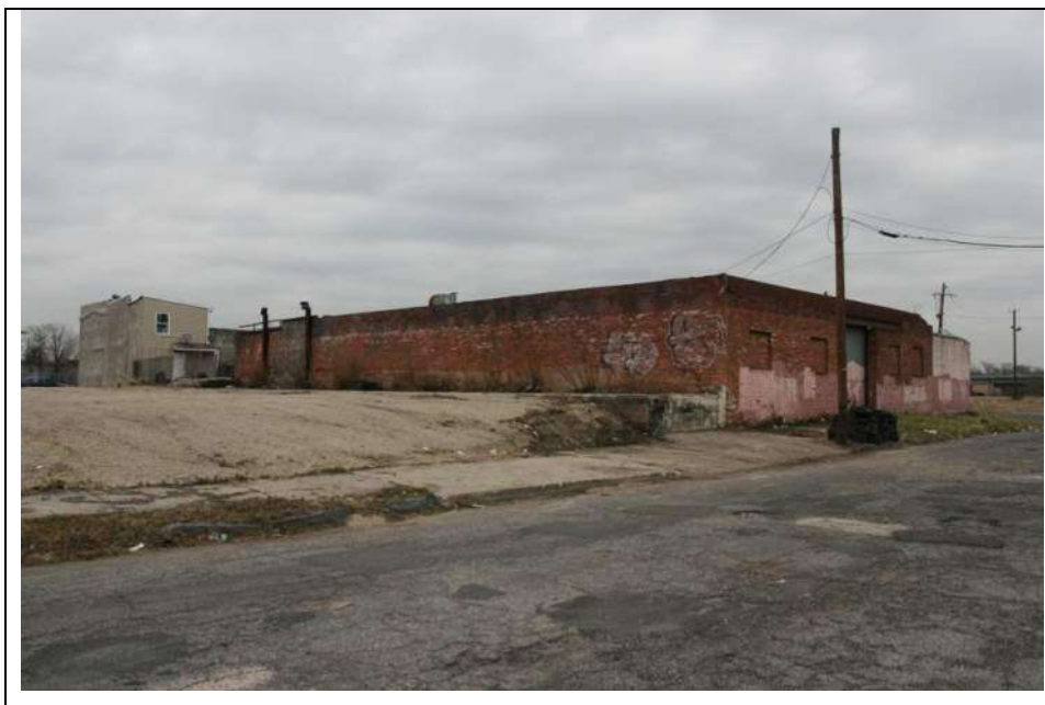
Photograph 8: West and south elevations of the brick wall enclosing the rear portion of the lot. Looking northeast (December 2018).
