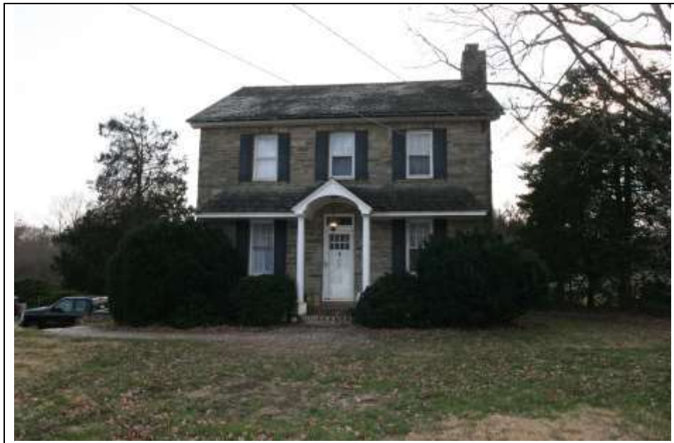
Photograph 1: Northeast elevation (façade) of dwelling at 856 Main Street. Looking southwest (December 2018).
