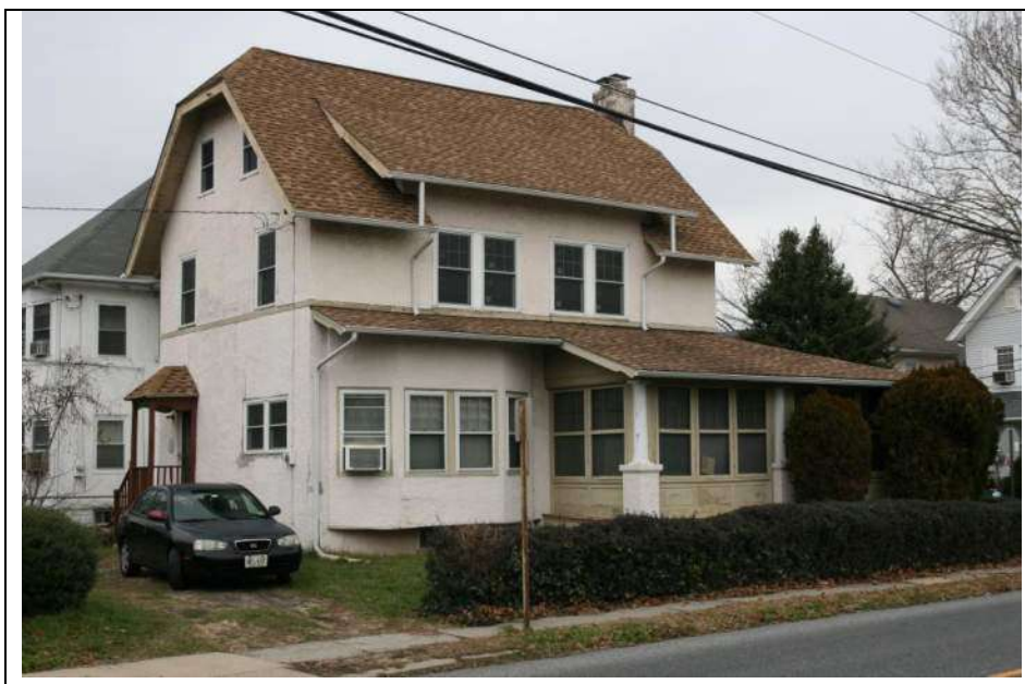
Photograph 3: Southwest (rear) and southeast (side) elevations of dwelling at 85 Aberdeen Place. Looking north (November 2018).
