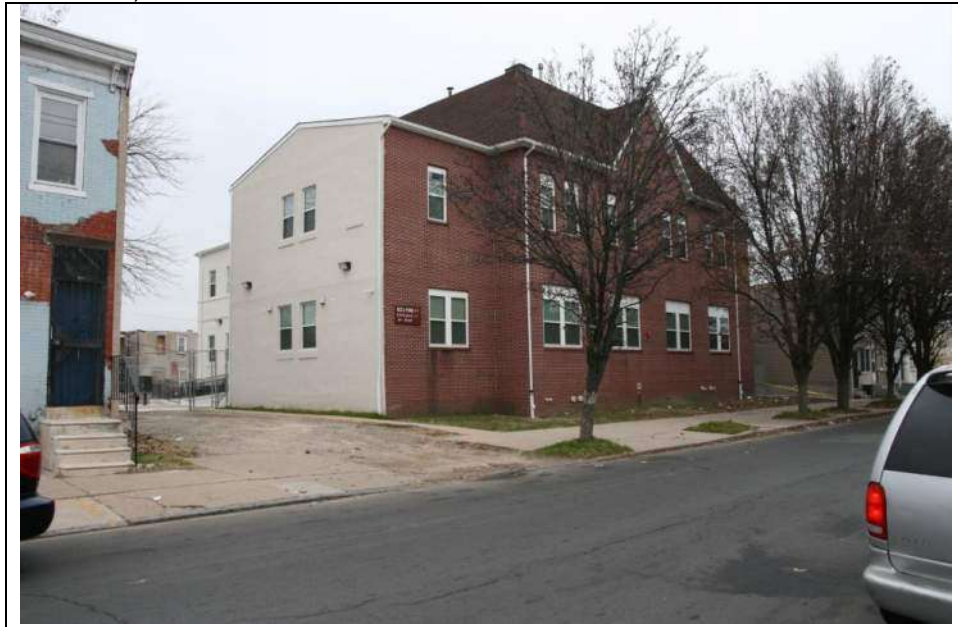
Photograph 1: West (side) and south (front) elevations of Jesse Starr School at 823 Pine Street. Looking northeast (December 2018).
