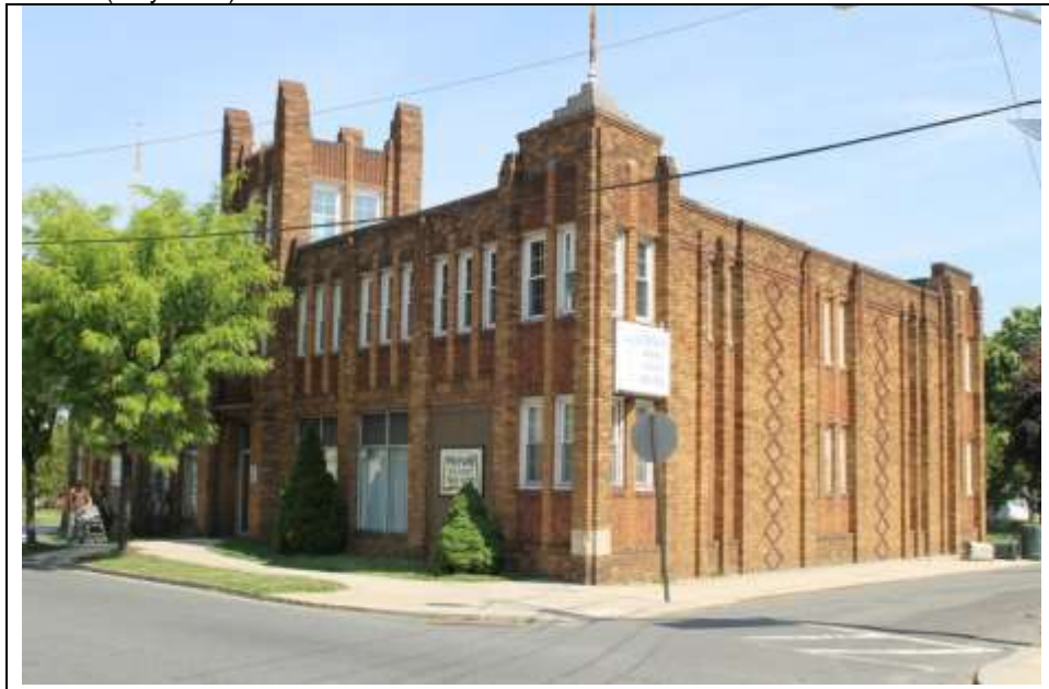
Photograph 1: South (front) and east (side) elevations of the former J.R. Quigley Company office and store at 811 Market Street. Looking northwest (May 2014).
