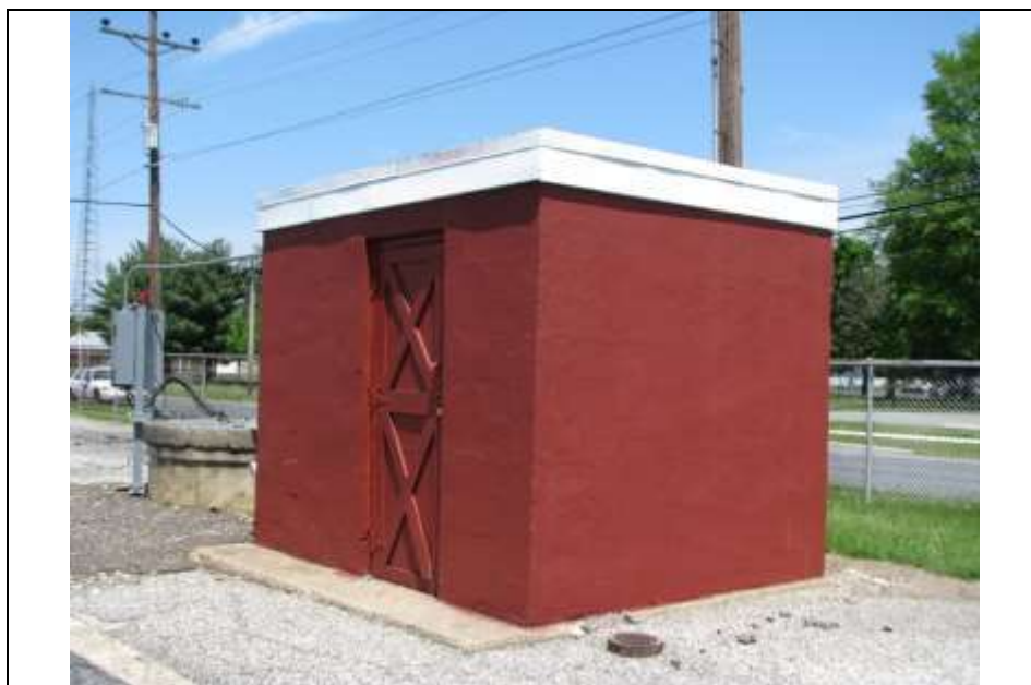
Photograph 29: Southwest (front) and southeast (side) elevations of the circa -1960 utility meter building. Looking north (May 2014).
