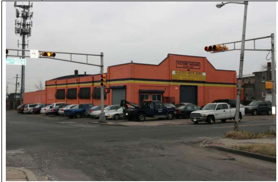
Photograph 1: East (side) and north (front) elevations of Victory Garage at 634 Kaighn Avenue. Looking southwest (December 2018).
