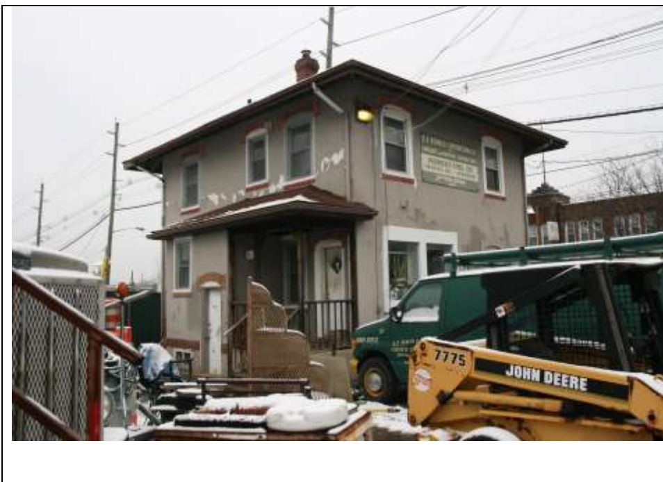
Photograph 4: Southwest (rear) and southeast (side) elevations. Looking northwest (January 2019).
