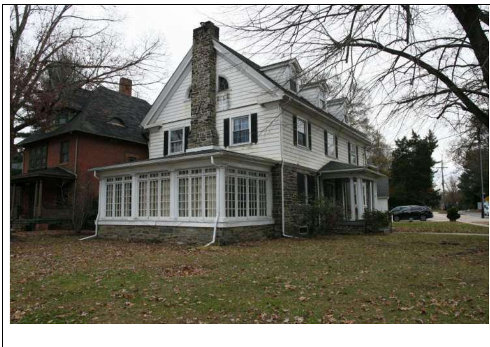
Photograph 3: South (side) and east (front) elevations of dwelling at 7 N. Evergreen Avenue. Looking north (November 2018).
