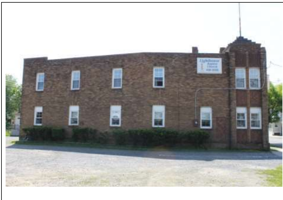
Photograph 6: West (side) elevation. Looking southeast (May 2014).
