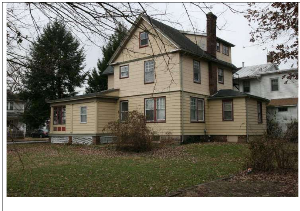
Photograph 3: Southeast (side) and northeast (rear) elevations of dwelling at 78 E. Centre Street. Looking west (November 2018).
