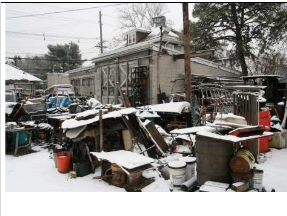
Photograph 10: Northwest (side) and southwest (rear) elevations of the Garage/Workshop. Looking northeast (January 2019).
