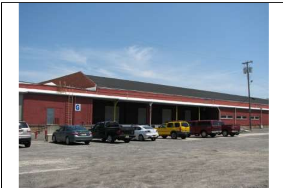
Photograph 11: Southwest elevation of the 1918 storehouse (Unit G). Note the modern doors and windows. Looking east (May 2014).
