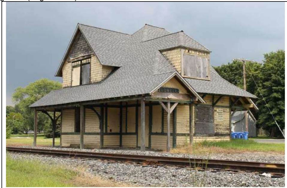
Photograph 1: Southwest (front) and southeast (side) elevations of the Sewell Train Station at 782 Atlantic Avenue. Looking north (August 2013).
