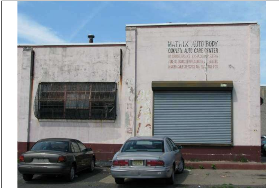
Photograph 6: Detail of east (side) elevation of Victory Garage, showing bays five and six, prior to repainting. Looking west (May 2014).
