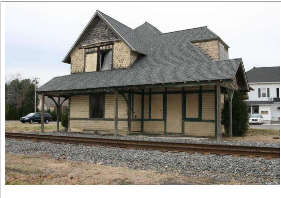
Photograph 3: Southwest (front) elevation of the Sewell Train Station, looking northeast (November 2018).
