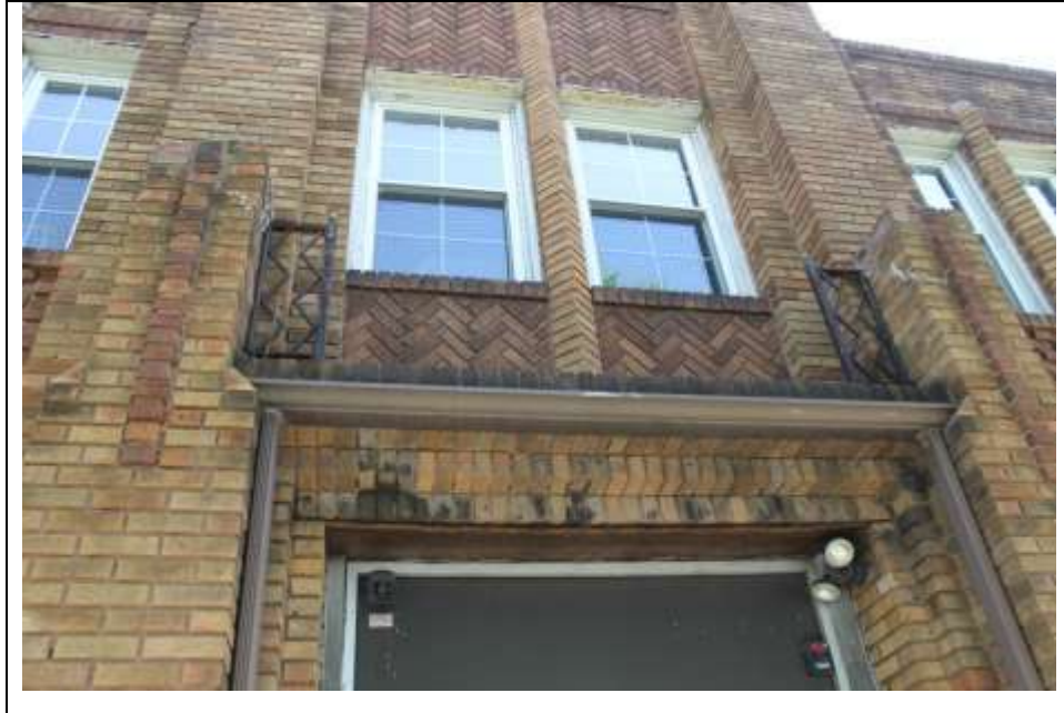
Photograph 4: Detail of brickwork and ironwork in the second story of the façade's central tower. Looking northeast (May 2014).
