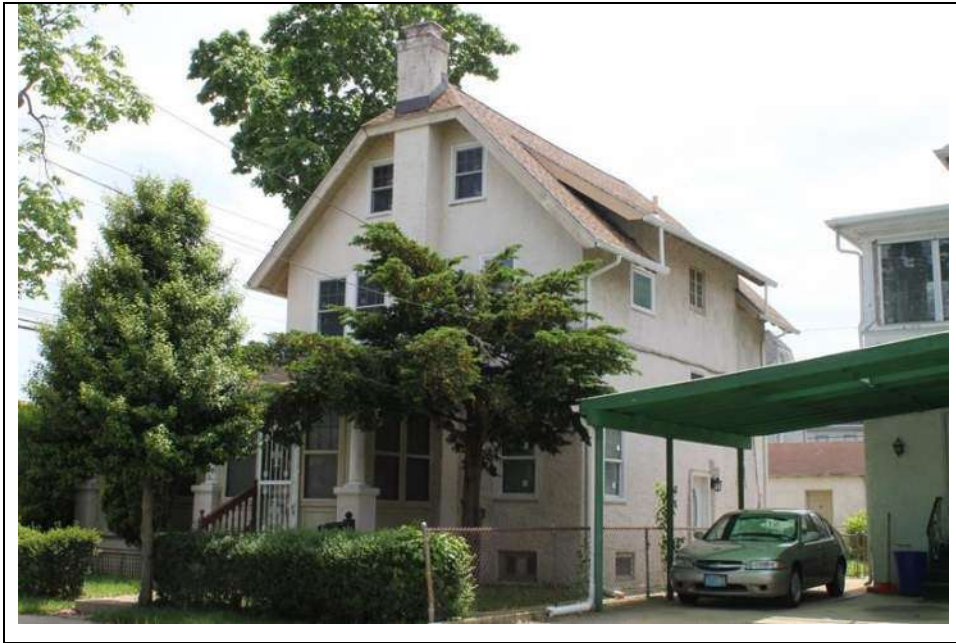
Photograph 4: Northeast (front) and northwest (side) elevations of dwelling at 85 Aberdeen Place. Looking south (May 2014).
