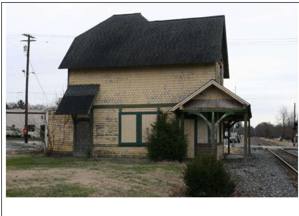
Photograph 4: Northwest (side) elevation of the Sewell Train Station, looking southeast (November 2018).
