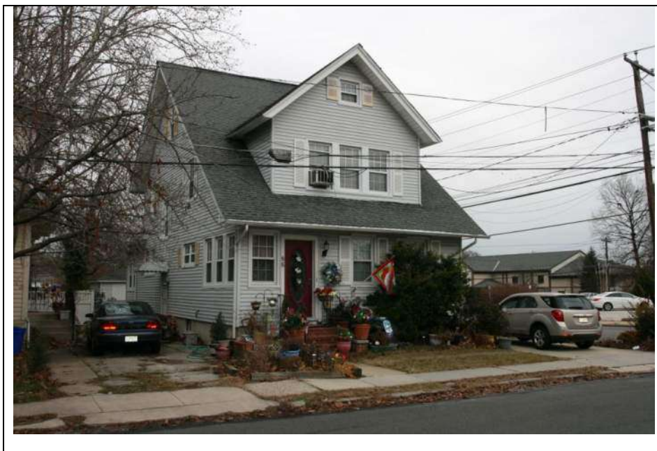
Photograph 2: Northwest (side) and southwest (front) elevations of dwelling at 86 Aberdeen Place. Looking northeast (November 2018).
