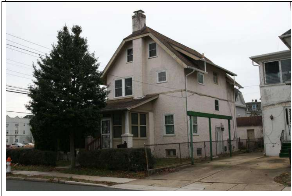
Photograph 1: Northeast (front) and northwest (side) elevations of dwelling at 85 Aberdeen Place. Looking south (November 2018).
