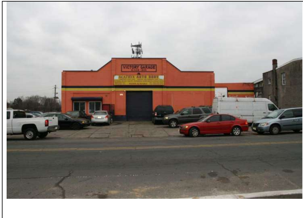
Photograph 2: North elevation (façade) of Victory Garage at 634 Kaighn Avenue. Looking south (December 2018).
