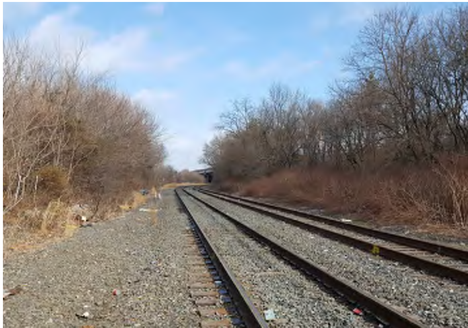
Photograph 62: View of the proposed GCL corridor along Railroad Avenue in Camden, facing north (February 2018).
