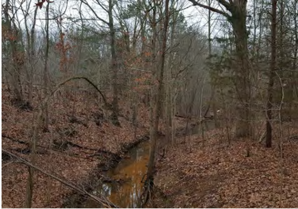
Photograph 63: View of a channelized creek at the base of the steep berm carrying the Conrail Line through Deptford Township, facing south (February 2018).
