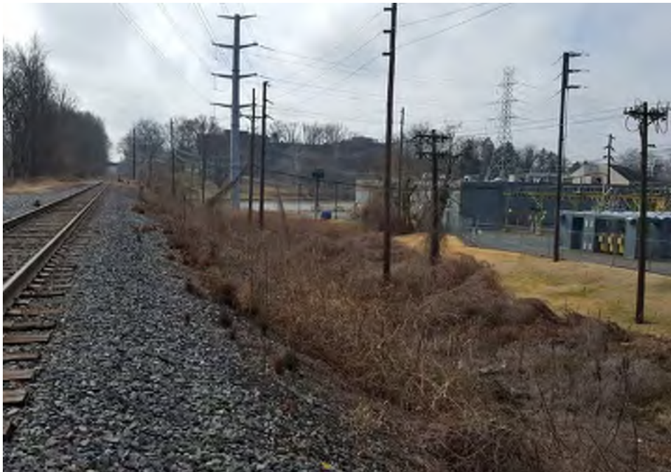
Photograph 38: View of the steep berm on the west side of the Conrail Line at the proposed Red Bank Avenue Station, facing southeast (February 2018).
