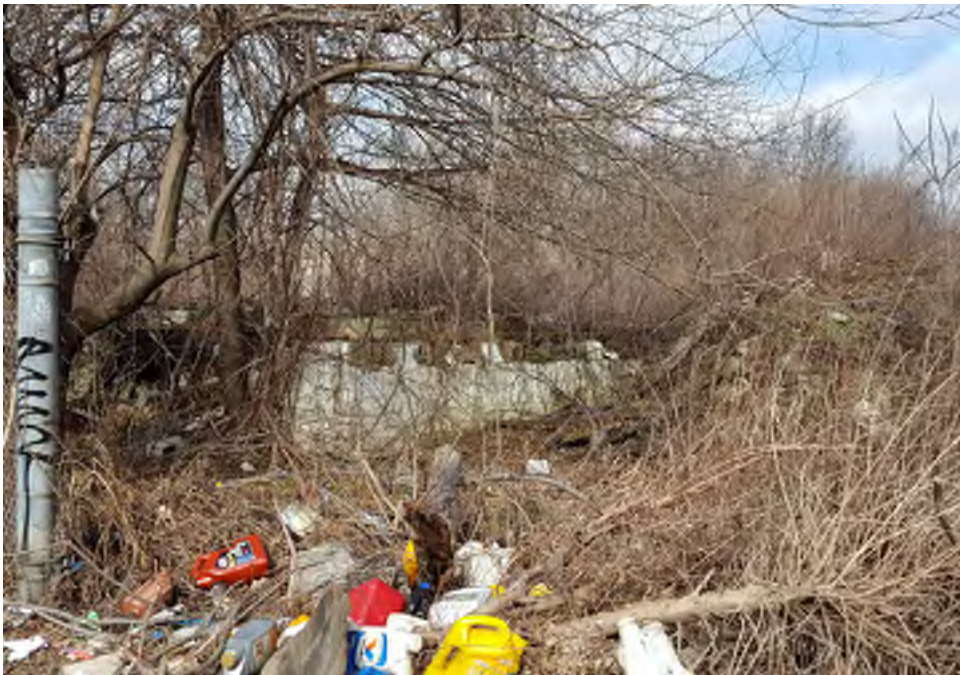
Photograph 11: View of the southern edge of Test Area 3 showing partially demolished buildings, spoil piles, and recent garbage piles, facing north (February 2018).
