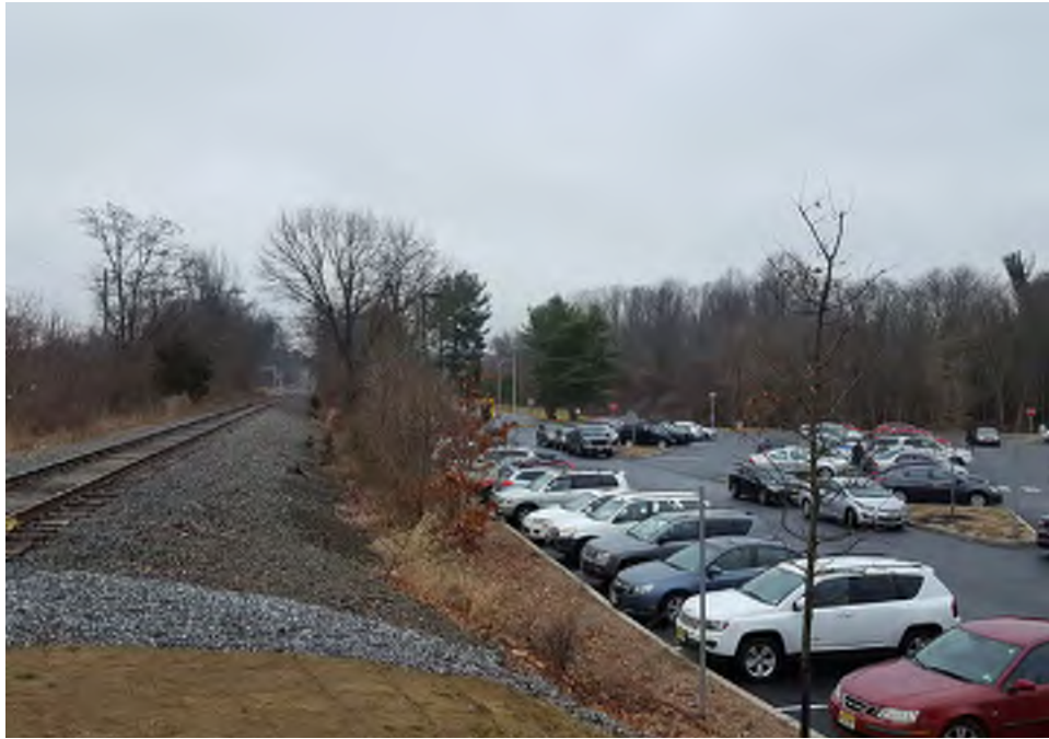
Photograph 43: View of the proposed Rowan University West Station showing the prepared railroad berm and parking lot on the east side, facing north (February 2018).
