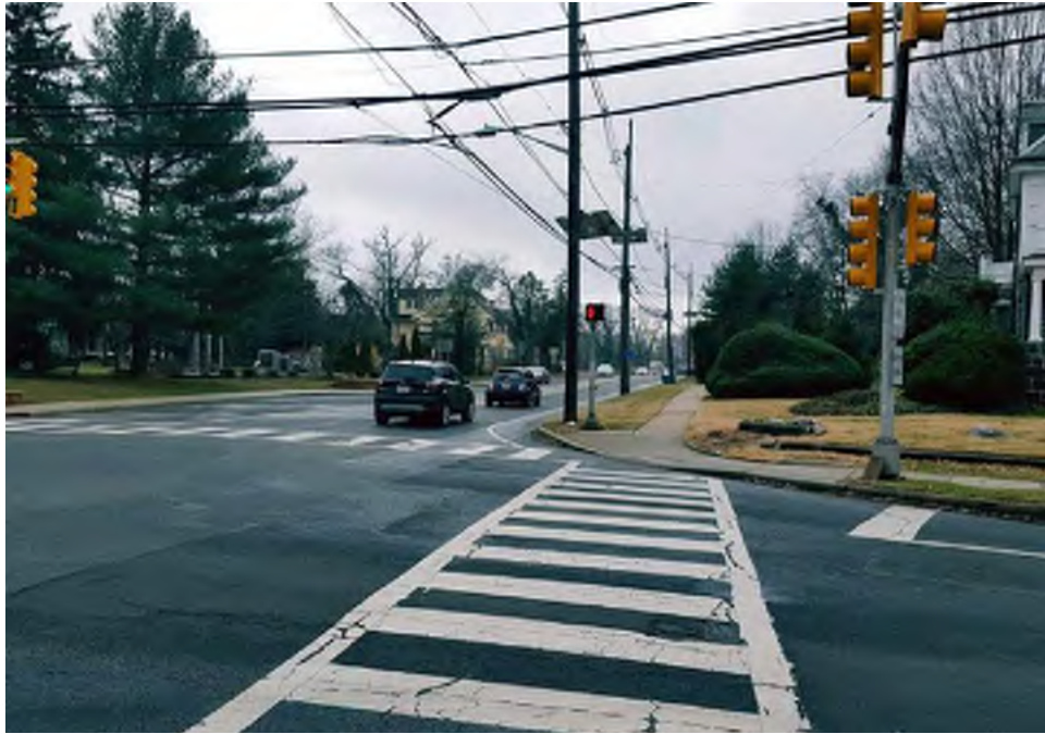
Photograph 54: View of the northwest quadrant of the Cooper Street intersection improvement area showing the road, sidewalk, and landscaped yard, facing northwest (February 2018).
