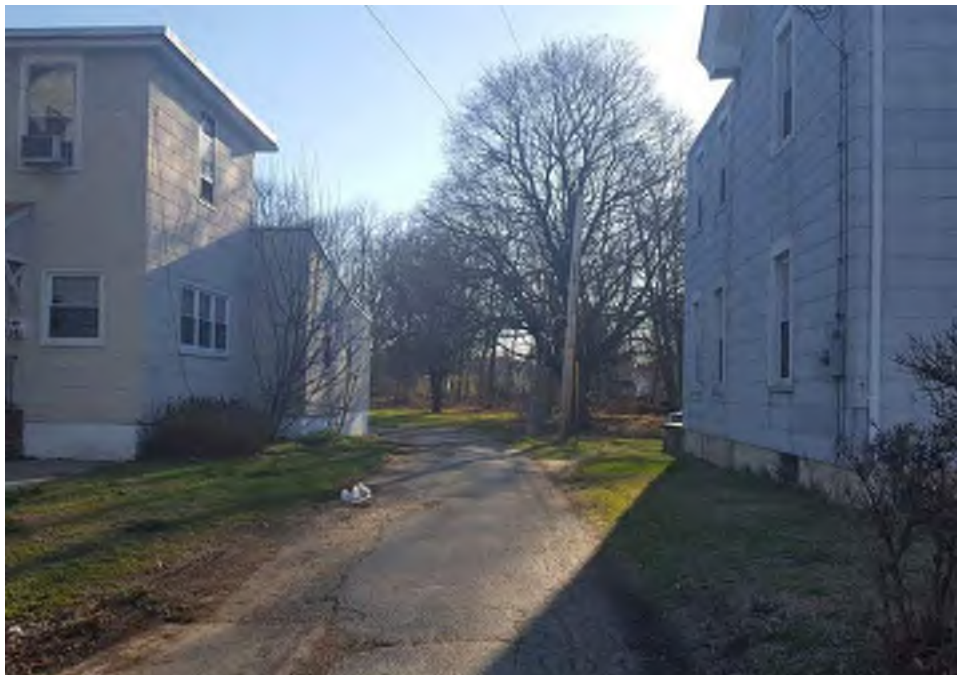
Photograph 28: View of the western end of Test Area 13 showing some of the nineteenth-century buildings at this location, facing east (February 2018).
