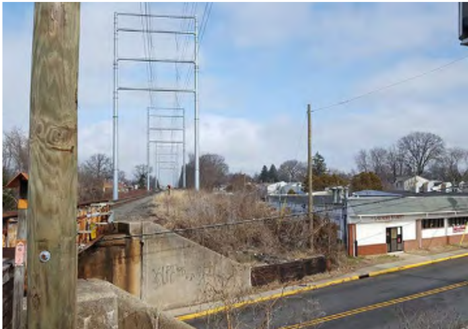
Photograph 42: View of the steep berm on the east side of the Conrail Line at the proposed Red Bank Avenue Station, facing northeast (February 2018).
