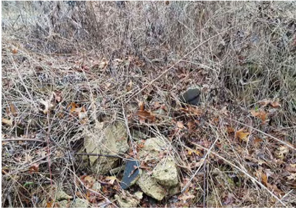
Photograph 47: View of concrete rubble in the north woods at the New Glassboro Yard Site, facing northwest (February 2018).
