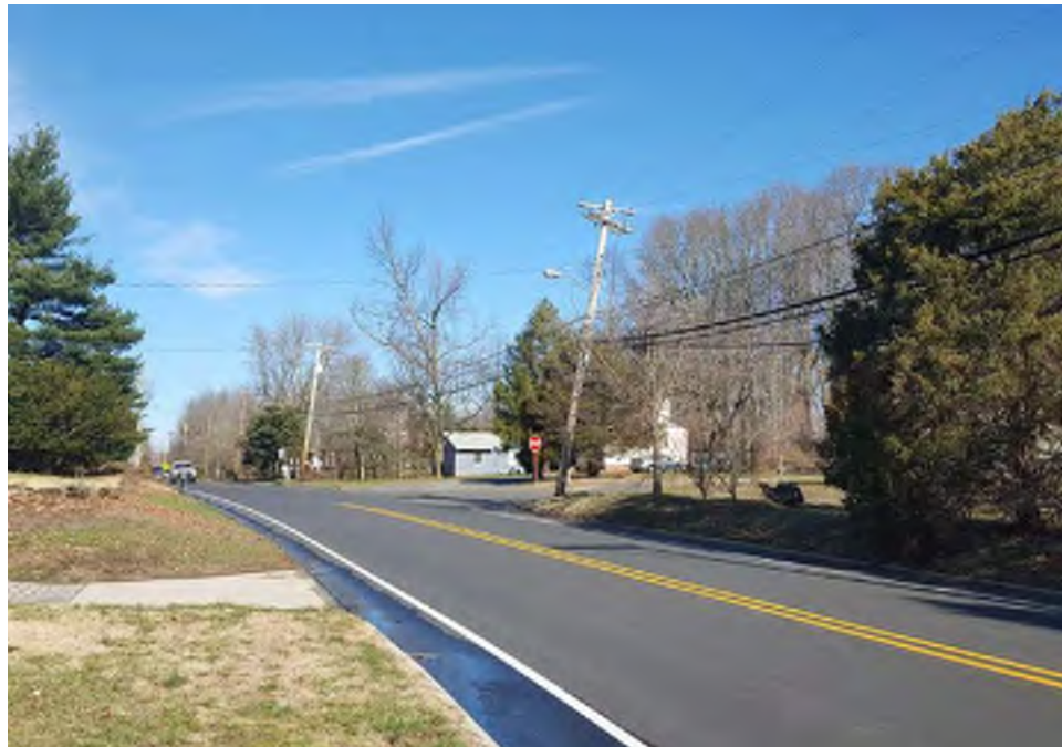
Photograph 55: View of the intersection at Tylers Mill Road and Main Street in Mantua Township showing the road, road berms, and underground utility corridors, facing northwest (February 2018).
