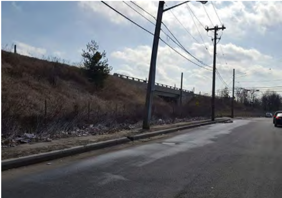
Photograph 3: View of the sloped berm of Test Area 2 from Pine Street in Camden, facing southeast (February 2018).
