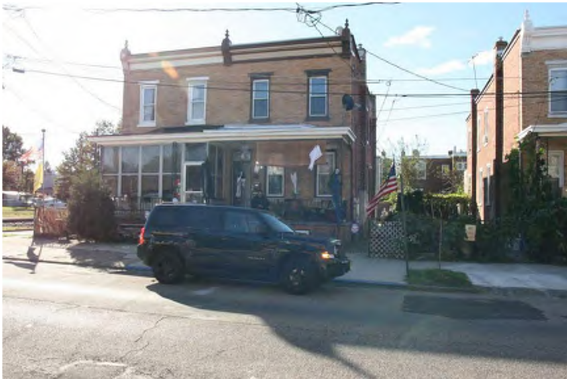
Photograph 16: 510-512 Chambers Avenue, Gloucester City (October 2018).
