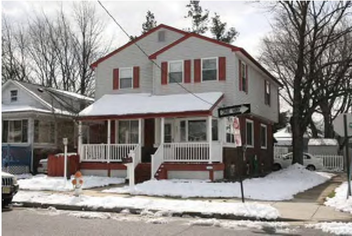
Photograph 3: 800 Mercer Street, Gloucester City (March 2018).
