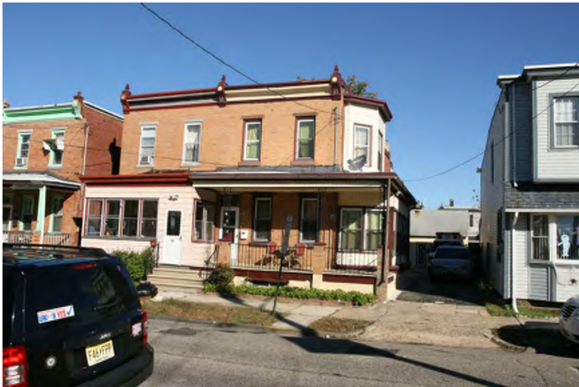
Photograph 14: 509-511 Chambers Avenue, Gloucester City (October 2018).
