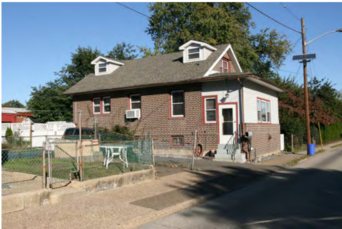
Photograph 6: 211 Railroad Avenue, Gloucester City (October 2018).
