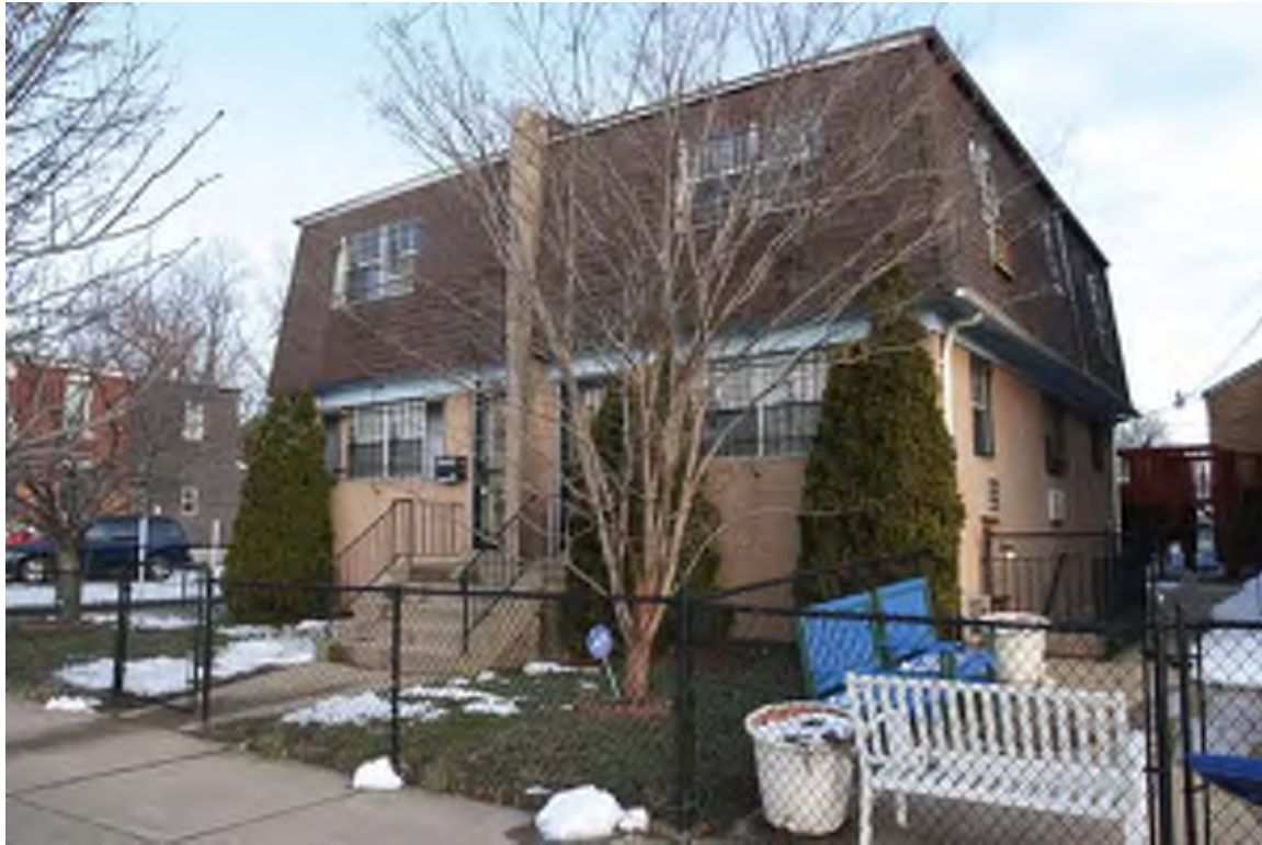
Photograph 1: 749-751 Kaighn Avenue, Camden City (March 2018).
