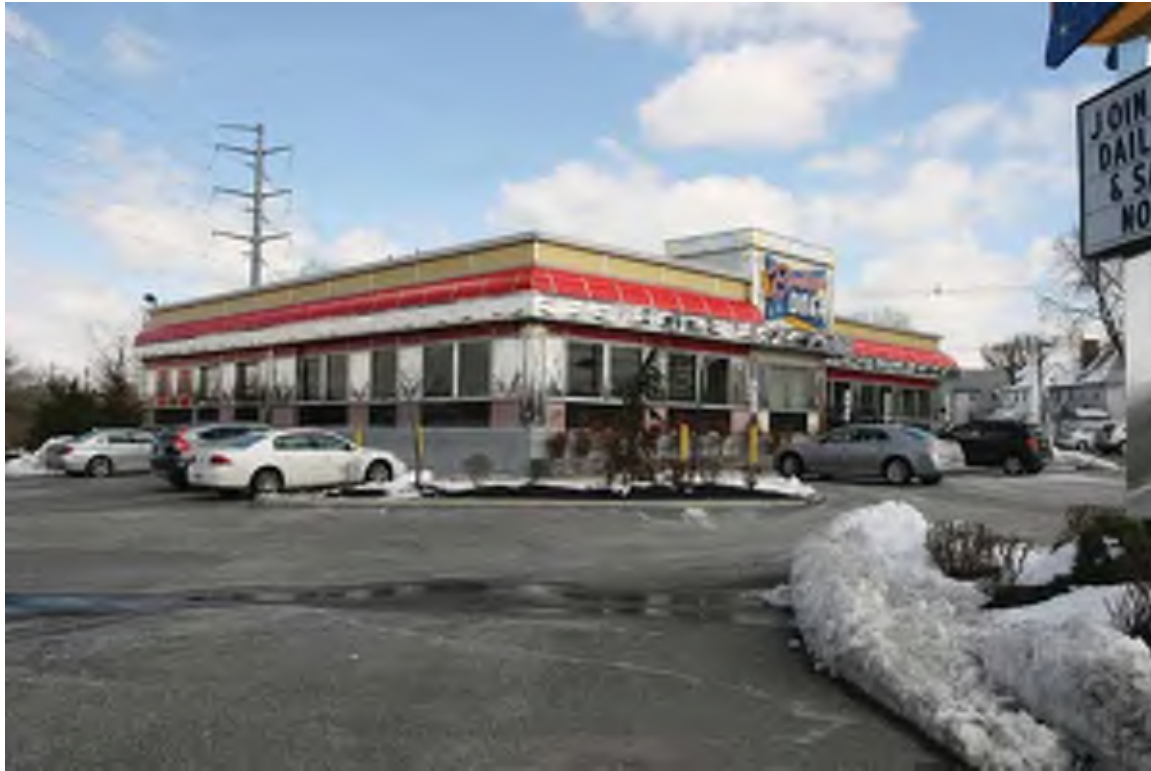
Photograph 5: 297 Crescent Boulevard, Brooklawn Borough (March 2018).
