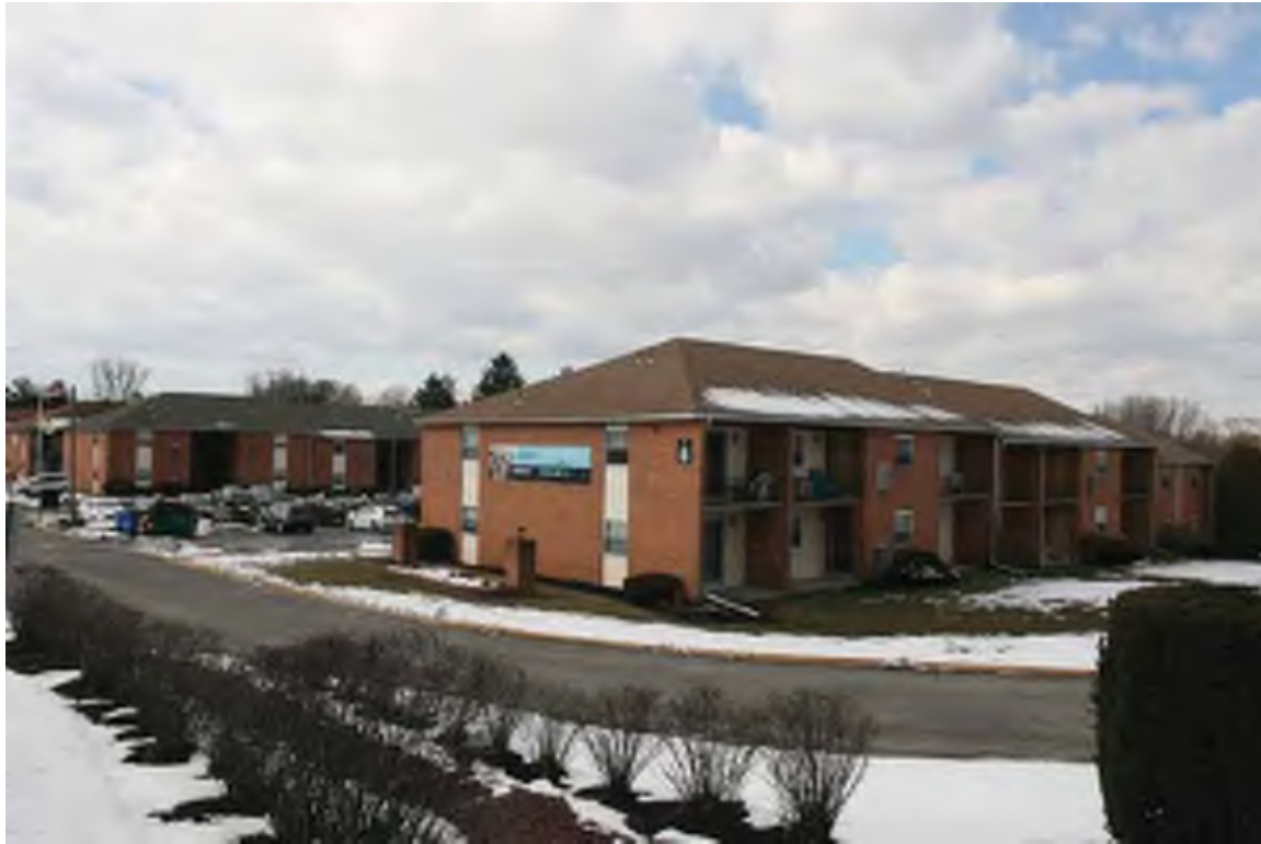
Photograph 25: Crossing at Glassboro, 515 Mullica Hill Road, Glassboro Borough (March 2018).
