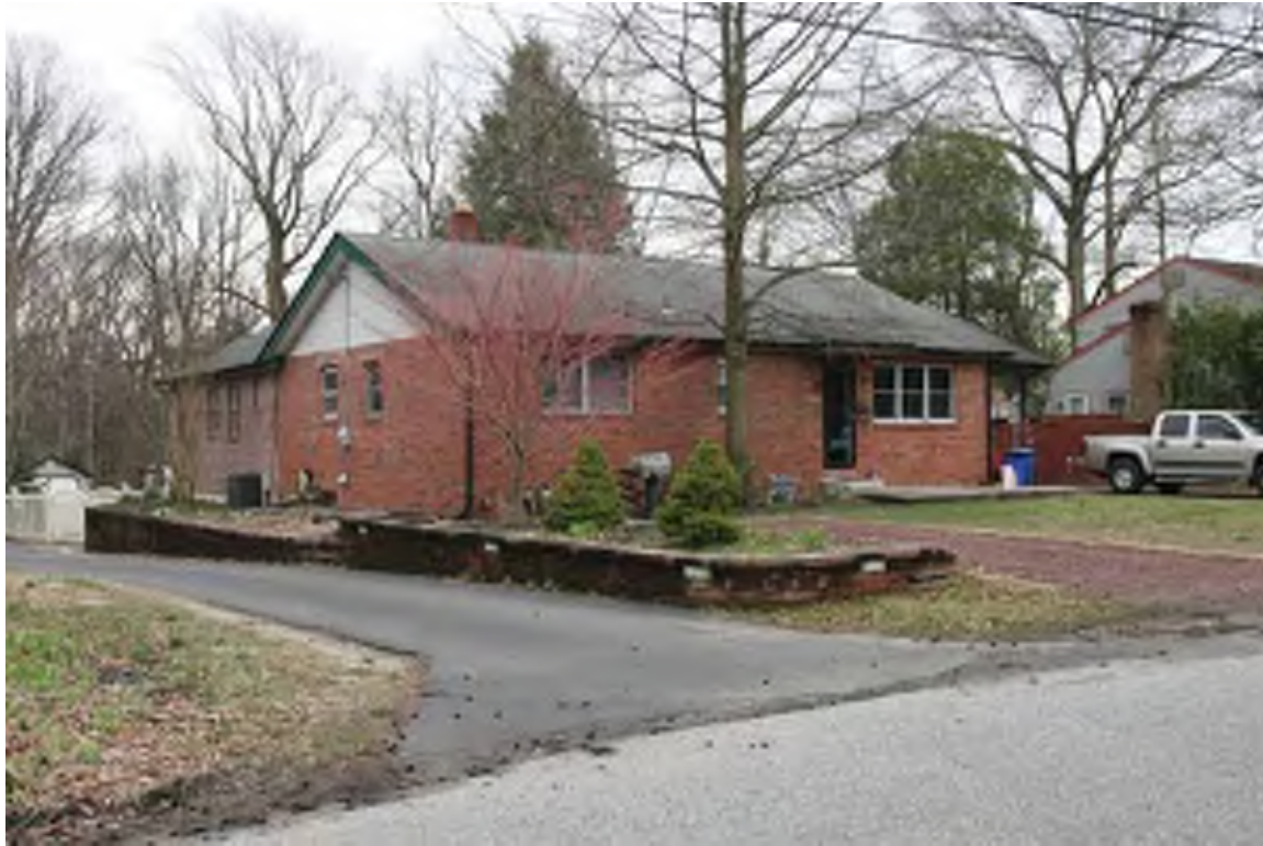
Photograph 7: 560 Barlow Avenue, Woodbury Heights Borough (April 2018).
