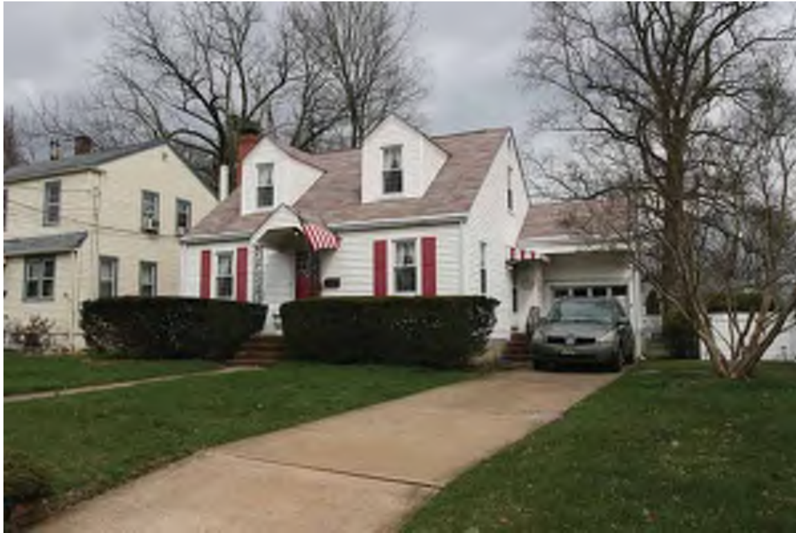
Photograph 17: 459 Oak Avenue, Woodbury Heights Borough (April 2018).
