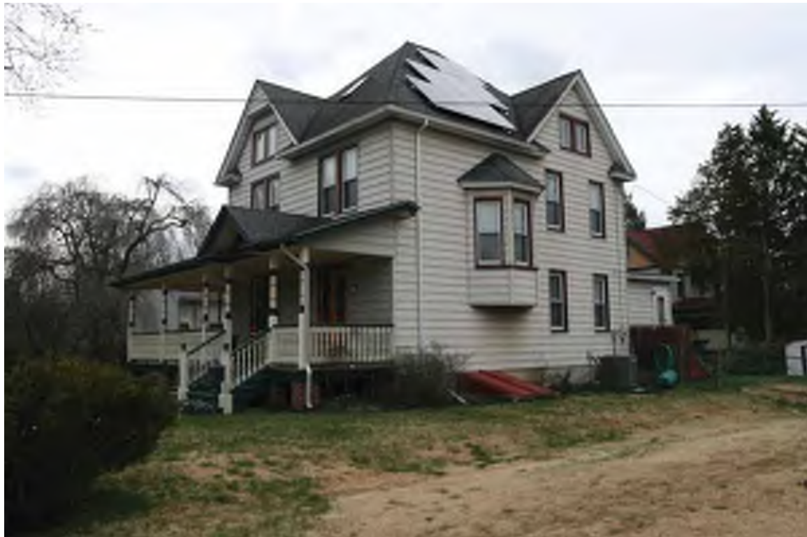
Photograph 18: 452 Oak Avenue, Woodbury Heights Borough (April 2018).
