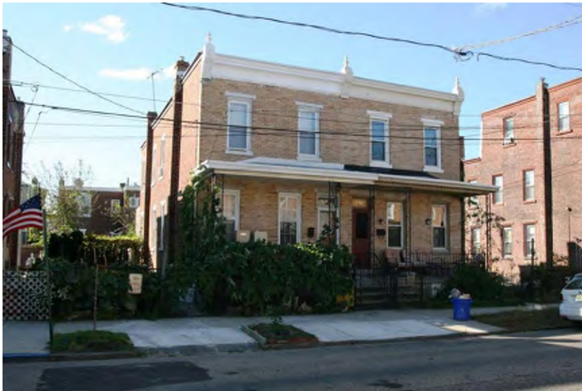
Photograph 17: 506-508 Chambers Avenue, Gloucester City (October 2018).
