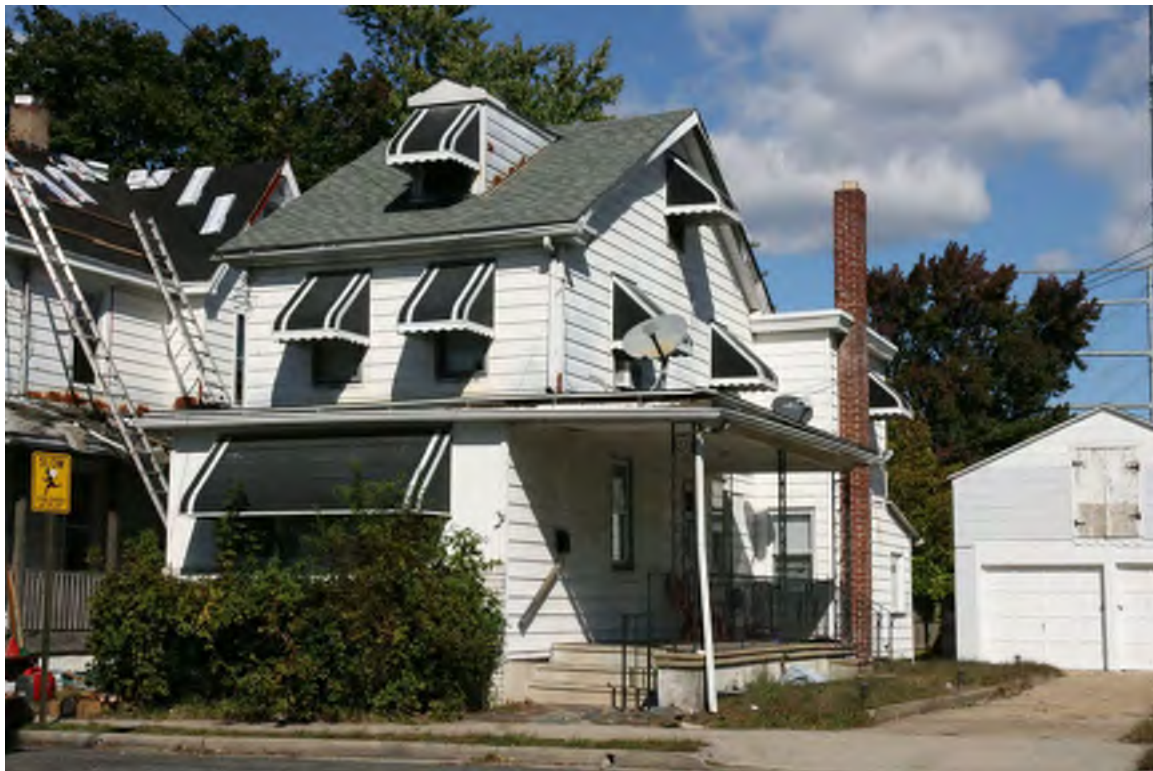
Photograph 40: 30 Dare Street, Woodbury City (October 2018).
