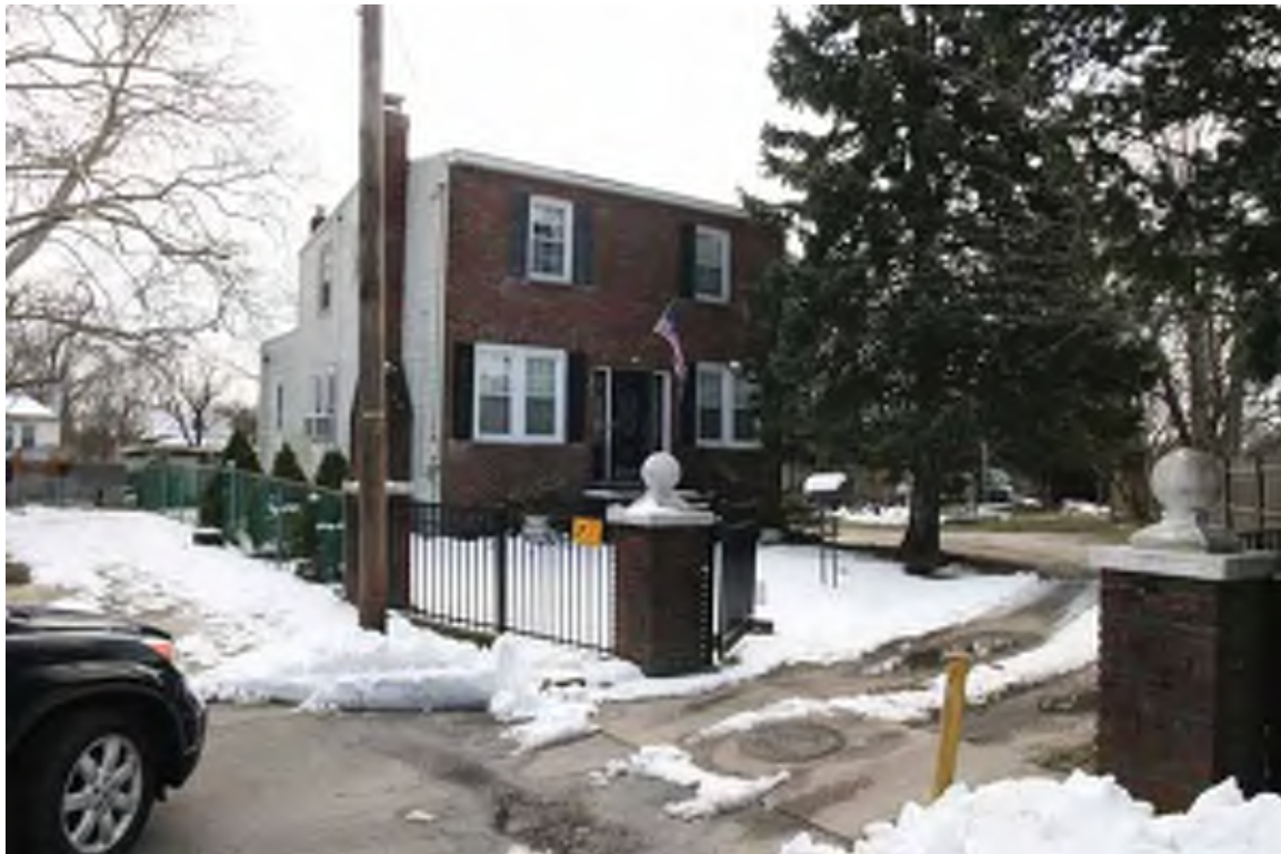
Photograph 4: 27 S. Stinson Avenue, Gloucester City (March 2018).
