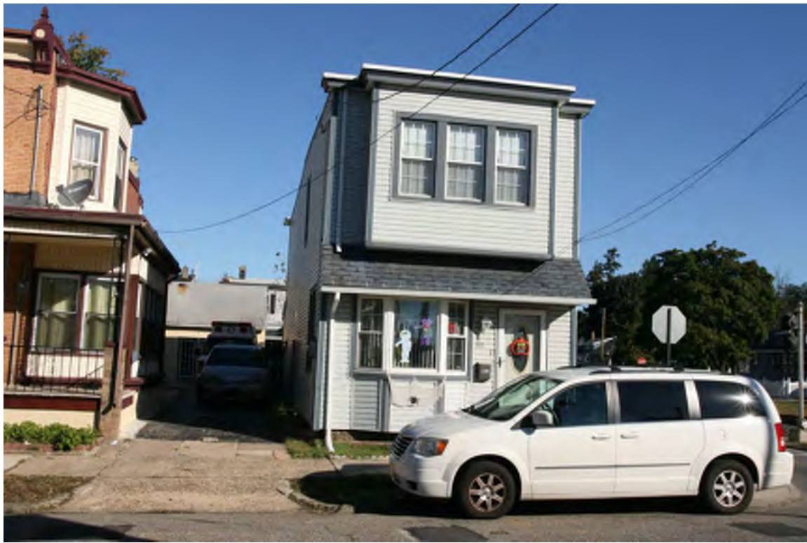
Photograph 15: 513 Chambers Avenue, Gloucester City (October 2018).
