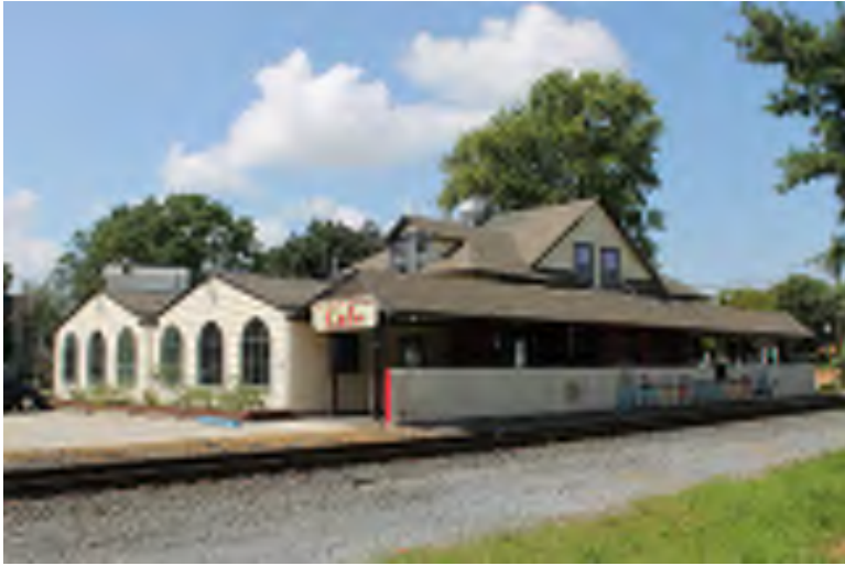
Photograph 137: 701 Monmouth Street (Gloucester City Train Station), Gloucester City. View of south (side) and east (front) elevations.
