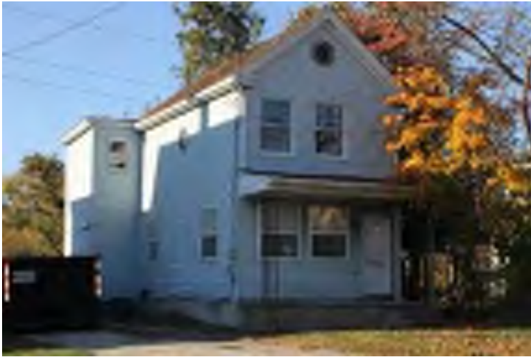
Photograph 81: 1190 Broadway, Deptford Township.
