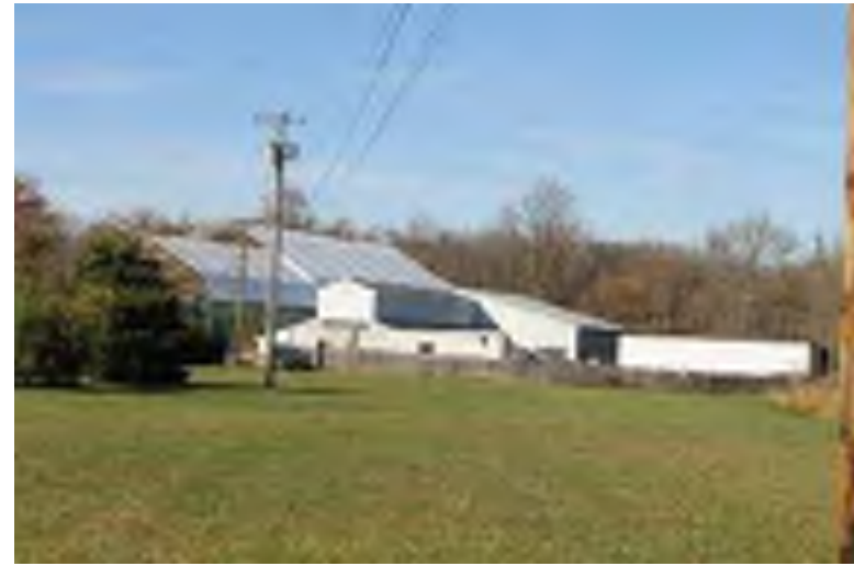
Photograph 166: 408 Lambs Road, Mantua Township.
