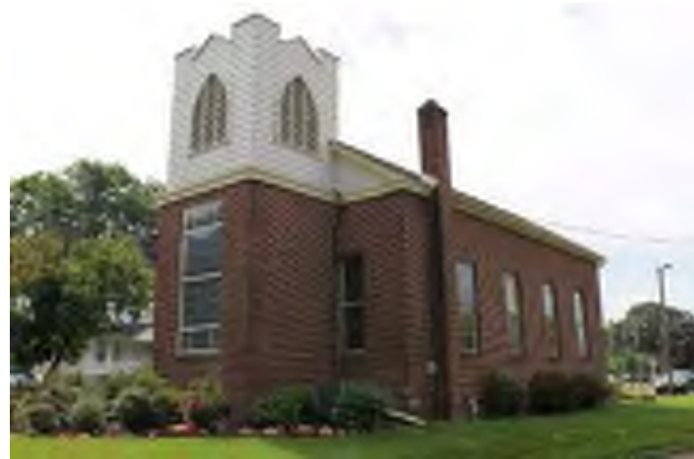
Photograph 100: Glassworks Residential District/South Glassboro, Glassboro Borough. View looking south toward Bethlehem United Church of Christ within the potential district.
