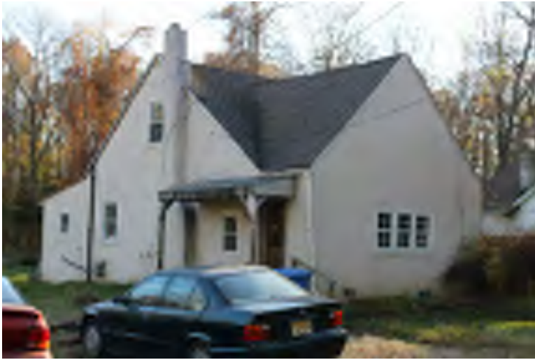
Photograph 89: Arthur Avenue (east of 566 Arthur Avenue and west of West Boulevard), Elk Township.
