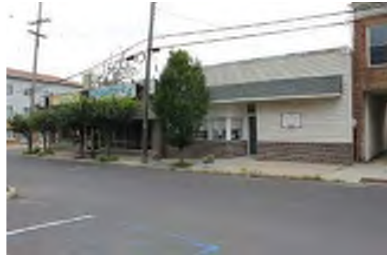
Photograph 192: W. Jersey Avenue Commercial Streetscape, Pitman Borough. View looking northeast toward 107 W. Jersey Avenue.
