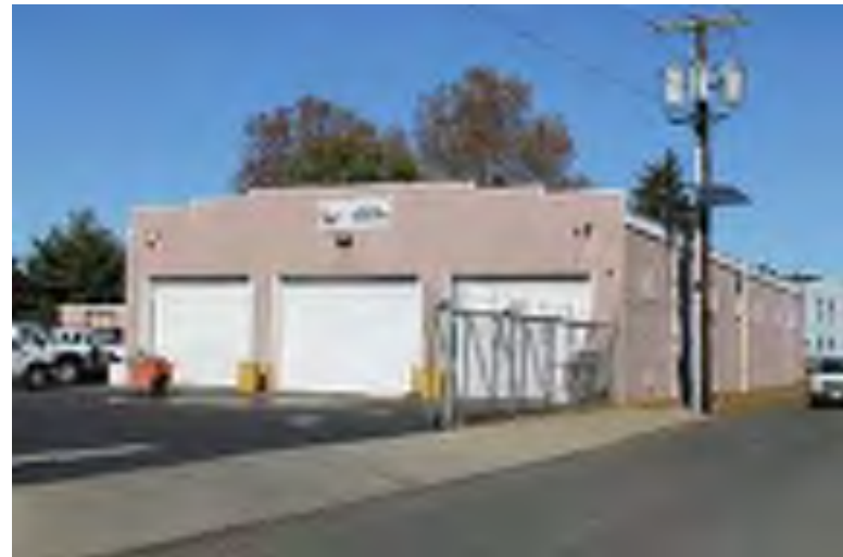
Photograph 152: 101 Washington Avenue, Gloucester City.
