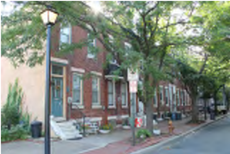
Photograph 75: Trenton Avenue Rowhouses (west of S. 9th Street), Camden City.
