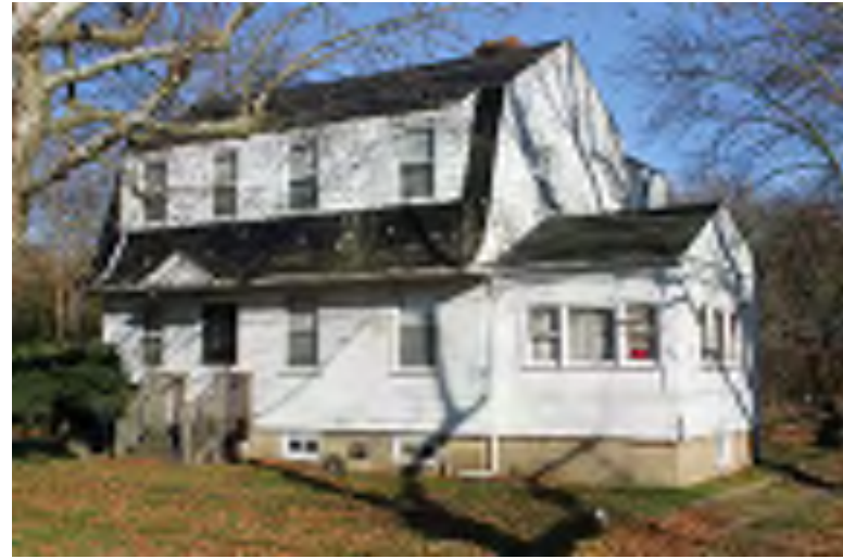
Photograph 94: 129 Buck Road, Elk Township.
