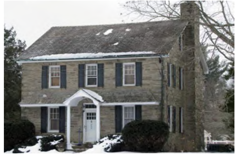
Photograph 54: 856 Main Street, Mantua Township.
