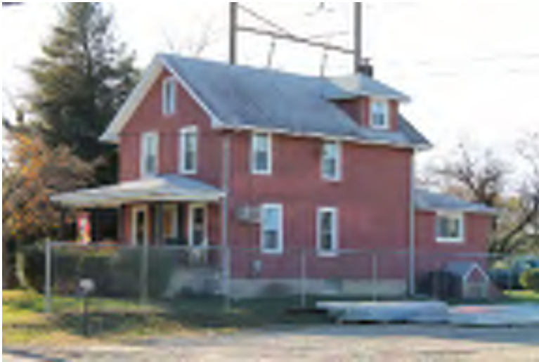
Photograph 79: 1180 Broadway, Deptford Township.
