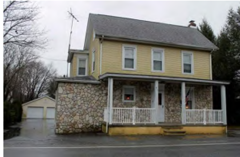
Photograph 14: 410 Ellis Street, Glassboro Borough.
