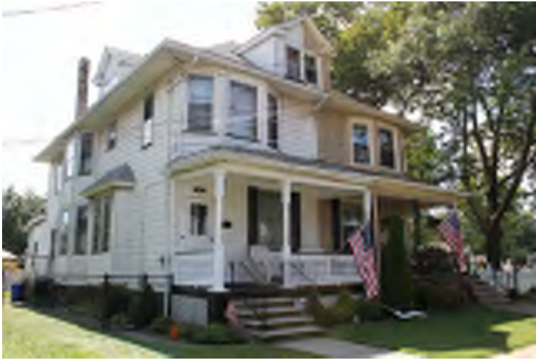
Photograph 141: Monmouth Street Streetscape (Railroad Avenue to Johnson Boulevard), Gloucester City. View looking southwest to 806-808 Monmouth Street within the potential district.
