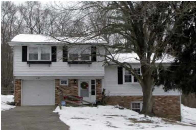
Photograph 63: 493 Tylers Mill Road, Mantua Township.
