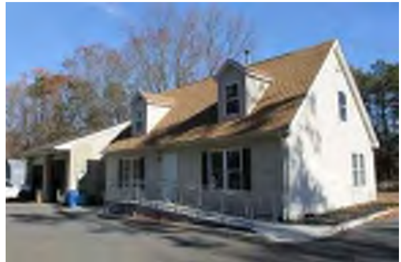
Photograph 200: W. Maple Street (Wenonah Public Works), Wenonah Borough.
