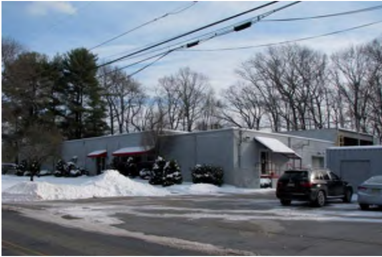
Photograph 57: 328 Tylers Mill Road, Mantua Township.
