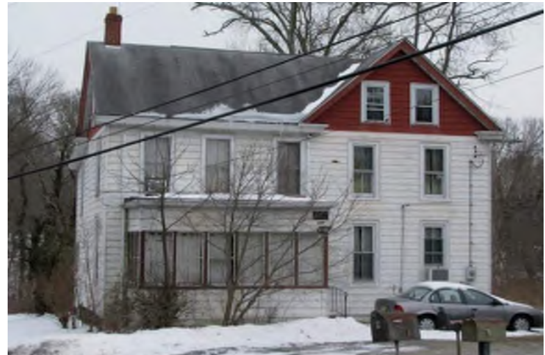
Photograph 64: 494 Tylers Mill Road, Mantua Township.
