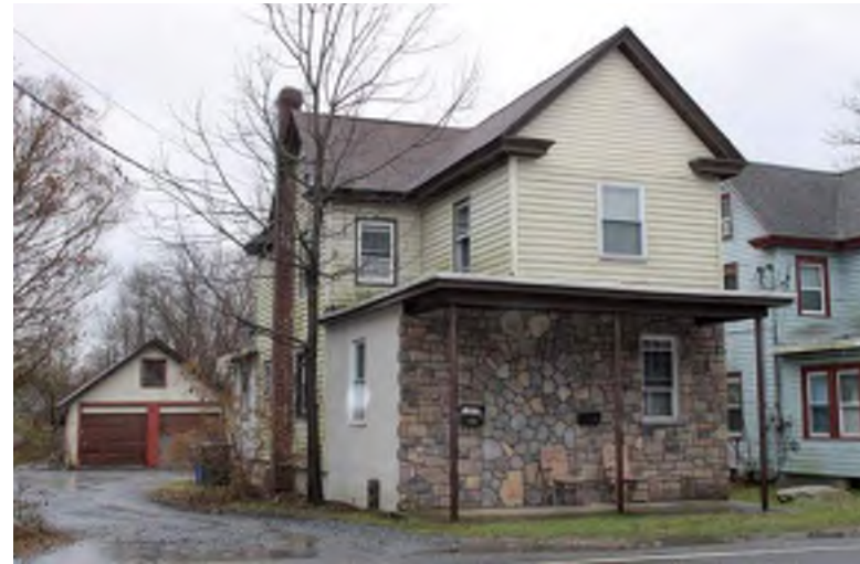
Photograph 12: 406 Ellis Street, Glassboro Borough.
