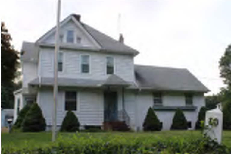
Photograph 281: W. Jersey Avenue (between 791 and 871), Woodbury Heights Borough.
