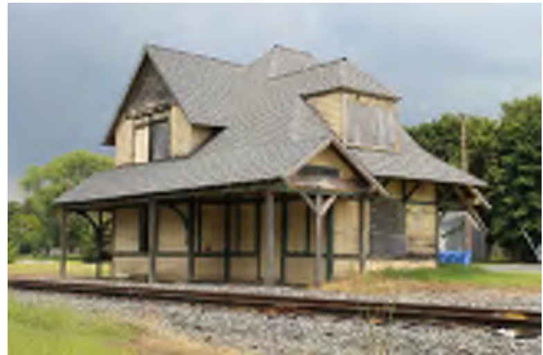
Photograph 160: W. Atlantic Avenue (Sewell Train Station), Sewell, Mantua Township.
