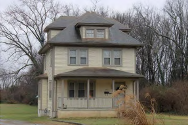
Photograph 17: 420 Ellis Street, Glassboro Borough.
