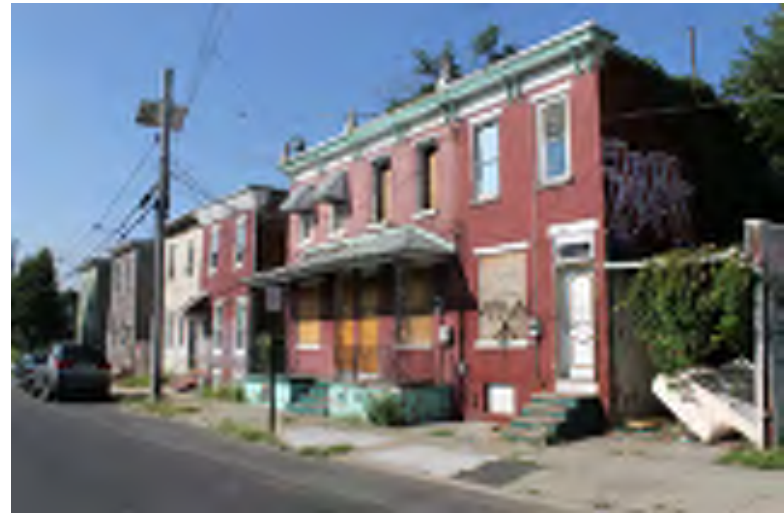
Photograph 36: S. 9th Street Streetscape (Ramona Gonzalez Street to Pine Street), Camden City.
