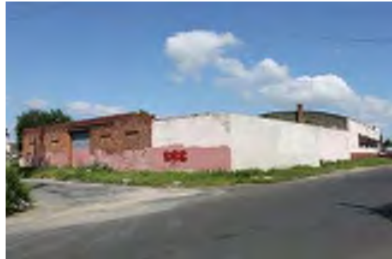
Photograph 52: 628-634 Kaighns Avenue (Victory Garage), Camden City. View of south (rear) and east (side) elevations.
