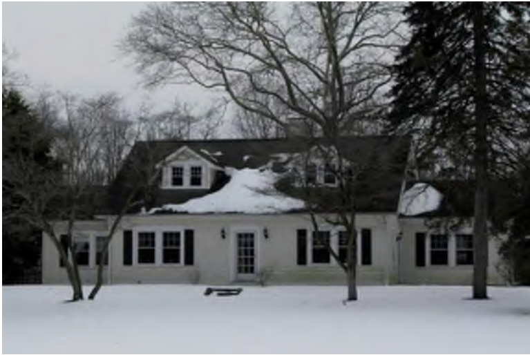
Photograph 49: 816 Main Street, Mantua Township.
