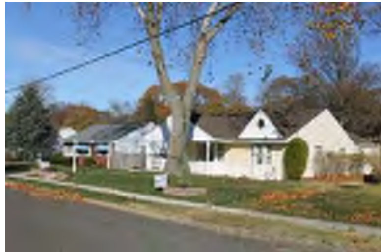
Photograph 176: Brookfield and Cedar Avenues Grouping, Pitman Borough. View looking northeast along Brookfield Avenue within the grouping.
