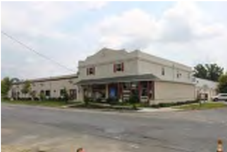
Photograph 163: 195 Center Street, Sewell, Mantua Township.
