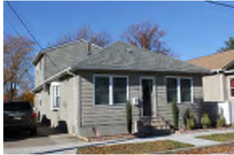
Photograph 150: 5 S. Stites Avenue, Gloucester City.
