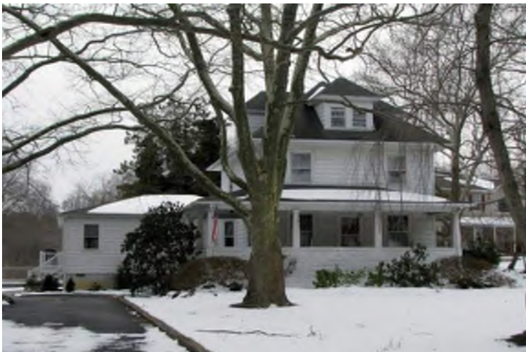
Photograph 51: 832 Main Street, Mantua Township.
