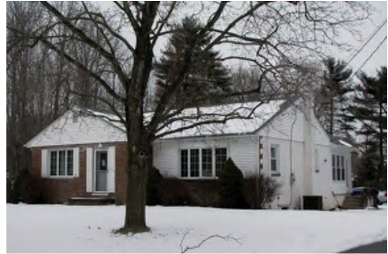
Photograph 50: 825 Main Street, Mantua Township.
