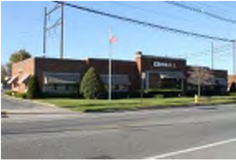
Photograph 85: Cornell & Co., Inc. building on Broadway (west-side, south of Gilbert Avenue), Deptford Township.
