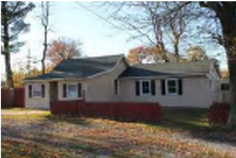
Photograph 83: 1240 Broadway, Deptford Township.
