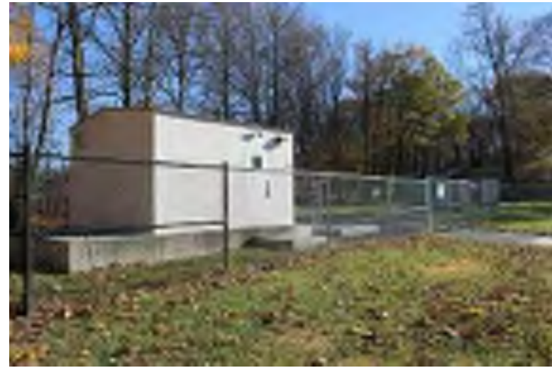
Photograph 86: Municipal Pumping Station No. 1 on Princeton Boulevard, Deptford Township.
