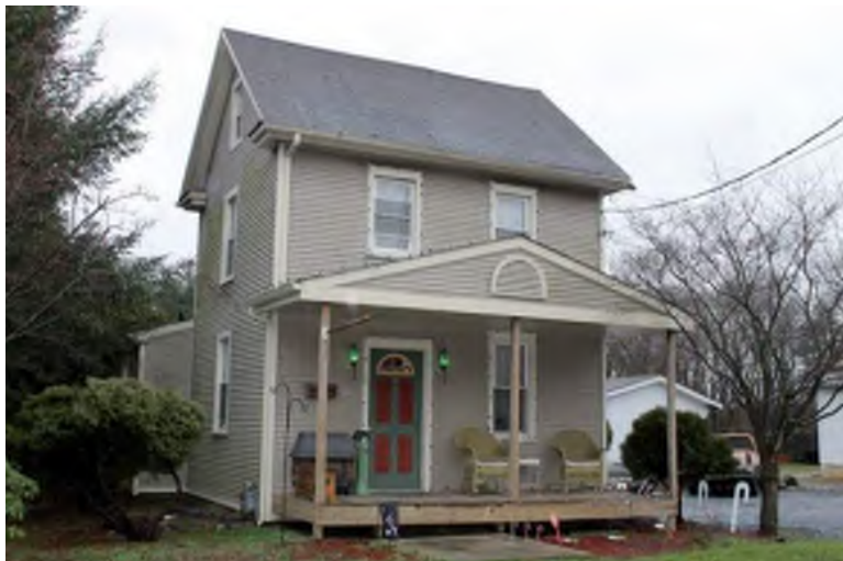
Photograph 15: 412 Ellis Street, Glassboro Borough.
