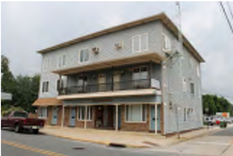
Photograph 195: 42-46 Pitman Avenue, Pitman Borough.
