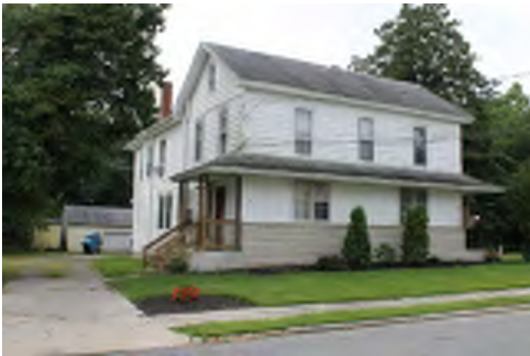
Photograph 115: 34 Zane Street, Glassboro Borough.
