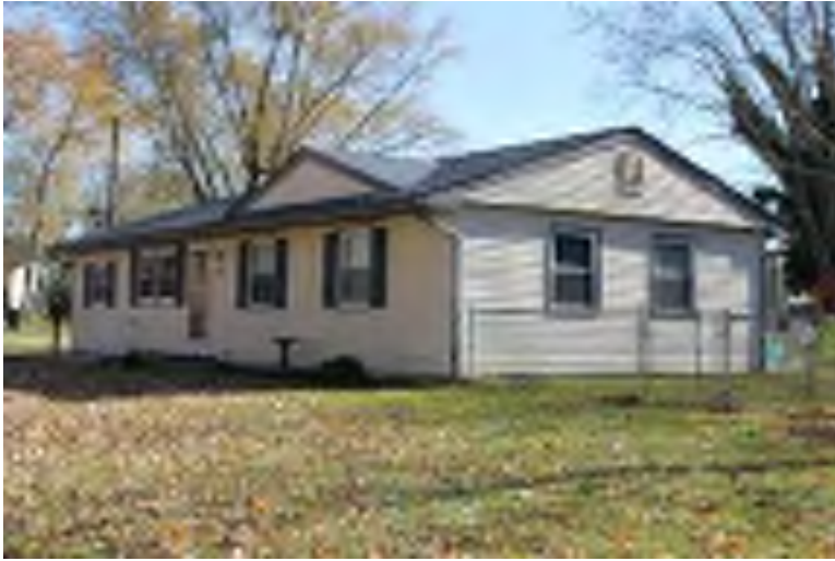
Photograph 161: Buckingham Village residential development, Sewell, Mantua Township. View looking southeast toward a representative dwelling at 500 Atlantic Avenue within the development.
