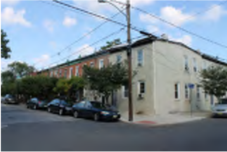
Photograph 77: Walnut Street Rowhouses (north-side, west of S. 9th Street), Camden City.
