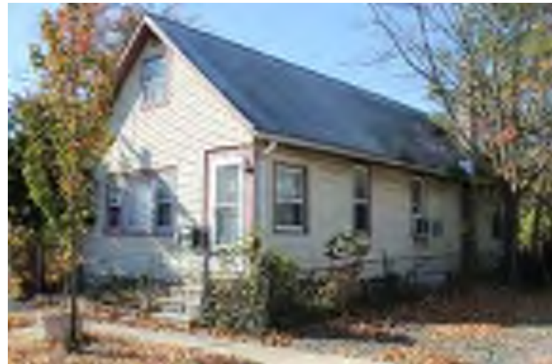
Photograph 148: 1 S. Stites Avenue, Gloucester City.
