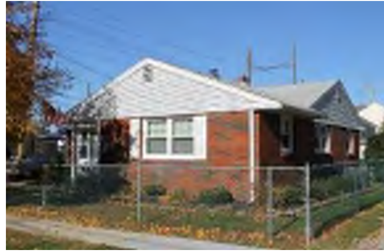
Photograph 26: 111 Browning Lane, Brooklawn Borough.
