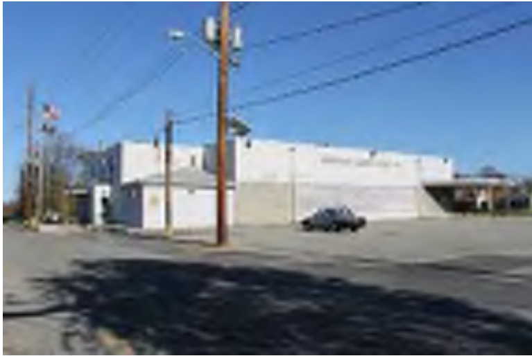
Photograph 29: 11 Railroad Lane (American Legion Post 72), Brooklawn Borough.
