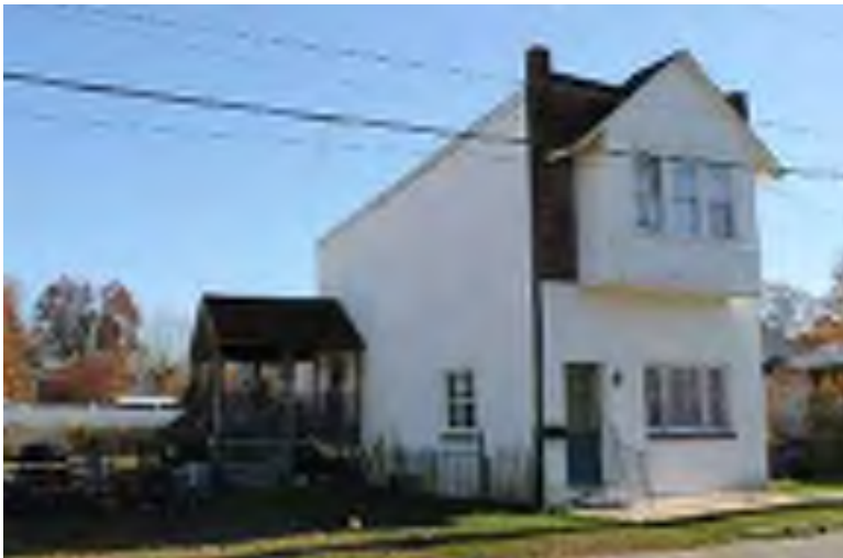
Photograph 27: 1 Railroad Lane, Brooklawn Borough.
