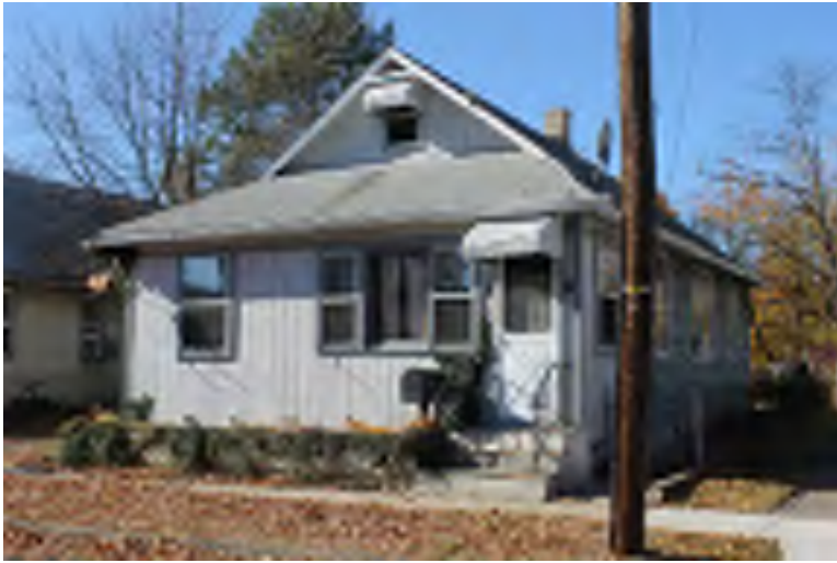
Photograph 149: 3 S. Stites Avenue, Gloucester City.
