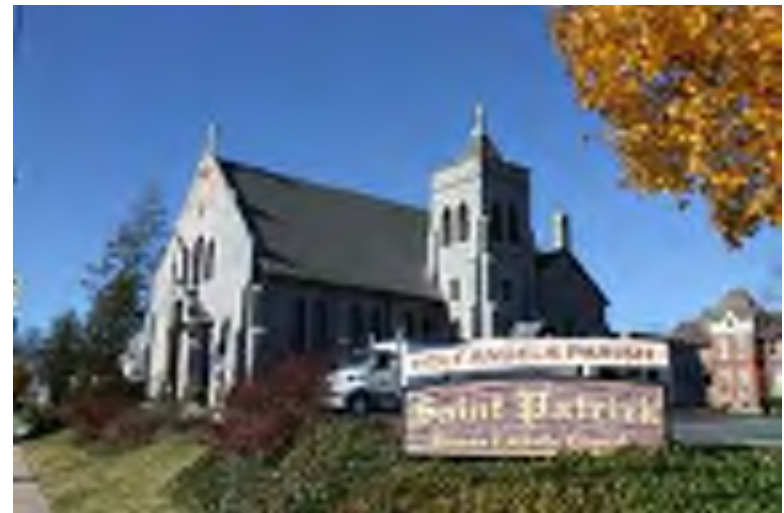
Photograph 20: St. Patrick Church at Cooper and Euclid Streets, a contributing resource to the Newton Historic District (NR eligible; SR Listed), Woodbury City. This building is also within the Woodbury Historic District (NR eligible; local certified district).
