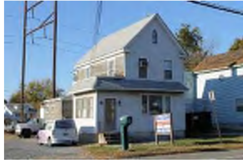
Photograph 82: 1198 Broadway, Deptford Township.
