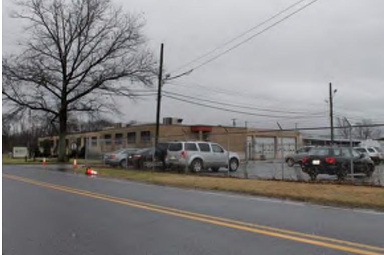
Photograph 19: 428 Ellis Street (Atlantic City Electric), Glassboro Borough.
