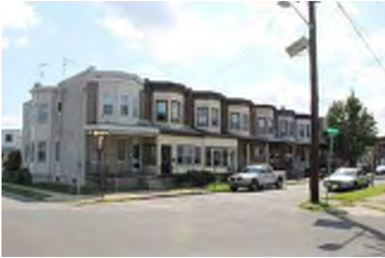
Photograph 145: Paul Street Rowhouses (south-side, west of Railroad Avenue), Gloucester City.
