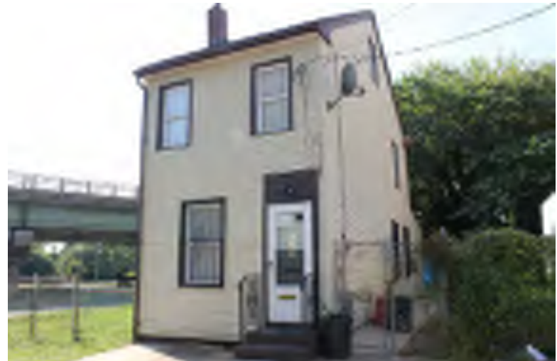
Photograph 64: 828 Mt. Vernon Street, at the east end of the Mt. Vernon St. Streetscape (south-side, 8th Street to 9th Street), Camden City.
