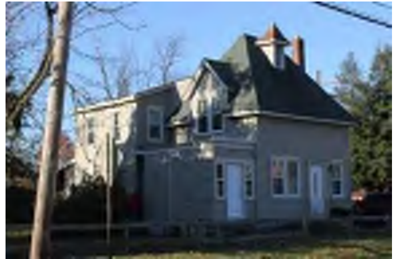
Photograph 80: 1184 Broadway, Deptford Township.
