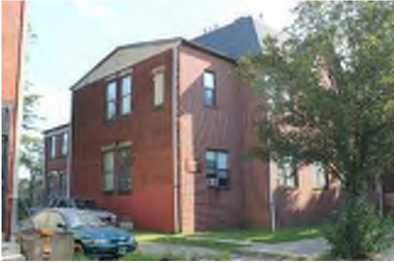
Photograph 5: Jesse Starr School (NR eligible), 823 Pine Street, Camden City. View of façade and west (side) elevation. The building has lost integrity as a result of extensive alterations since the previous evaluation and appears to be no longer eligible for listing in the NR.
