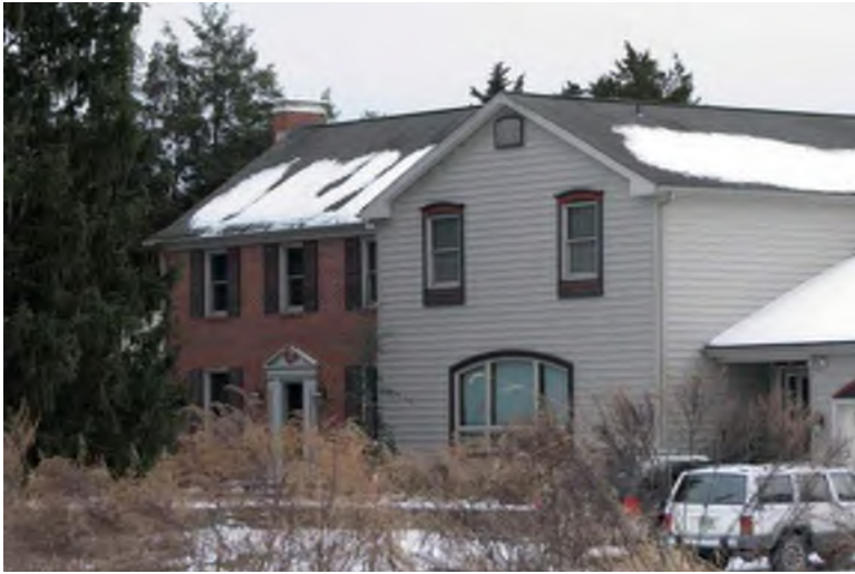
Photograph 53: 844 Main Street, Mantua Township. Detail of original dwelling facade (left) and circa -2000 addition.
