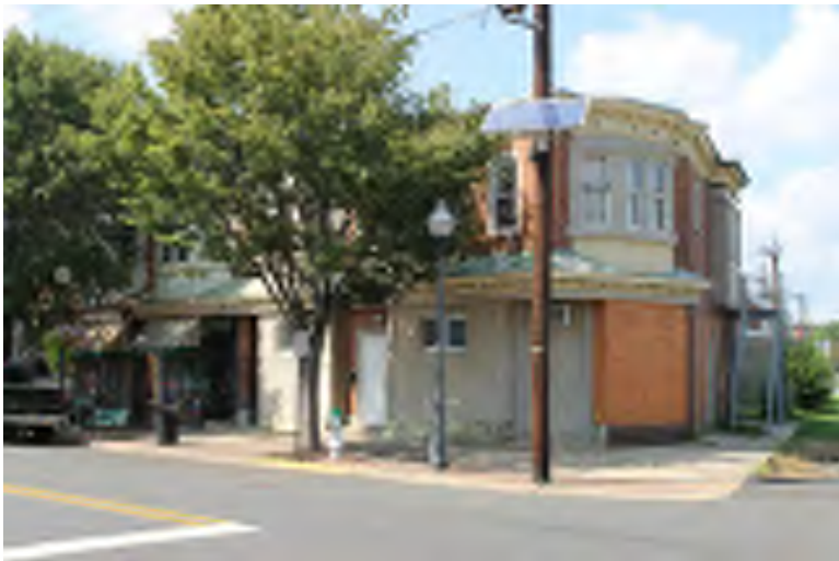
Photograph 139: Monmouth Street Commercial Row, Gloucester City.
