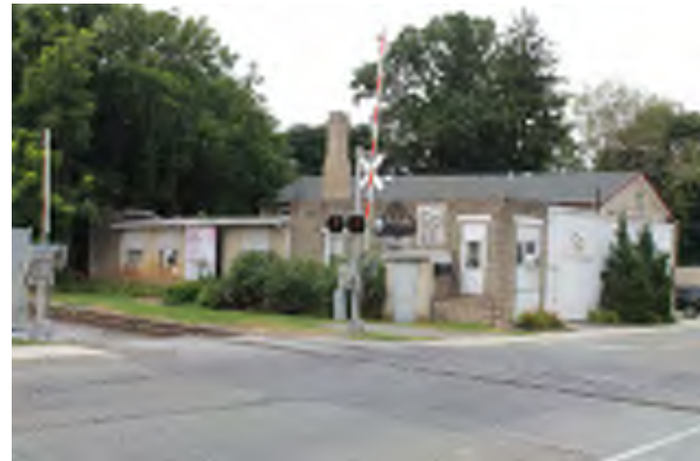
Photograph 180: 51-53 E, Holly Avenue (Pitman Grove Review Printing), Pitman Borough.
