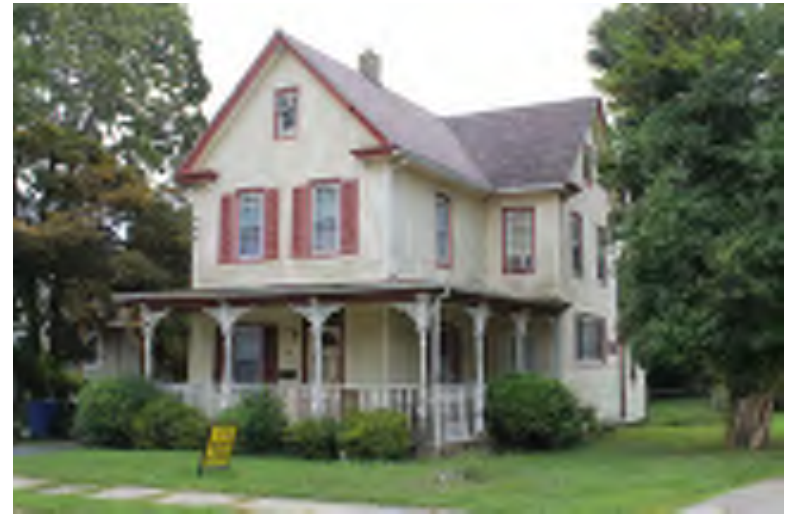
Photograph 114: 32 Zane Street, Glassboro Borough.
