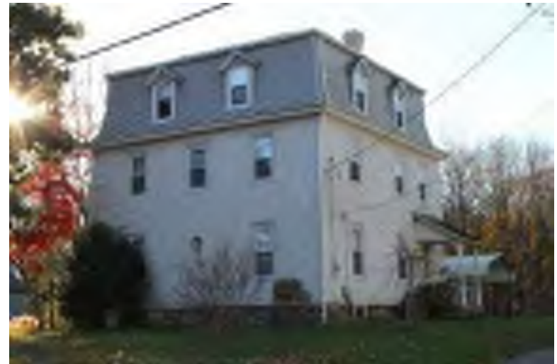
Photograph 92: 120 Buck Road, Elk Township.
