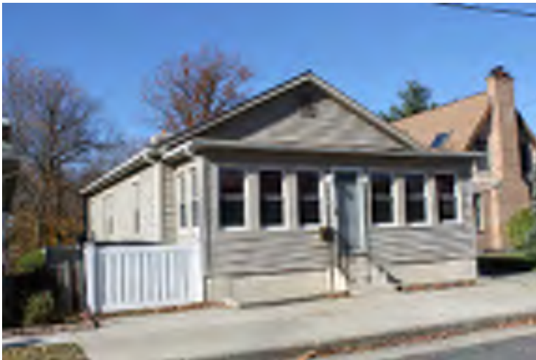
Photograph 151: 7 S. Stites Avenue, Gloucester City.
