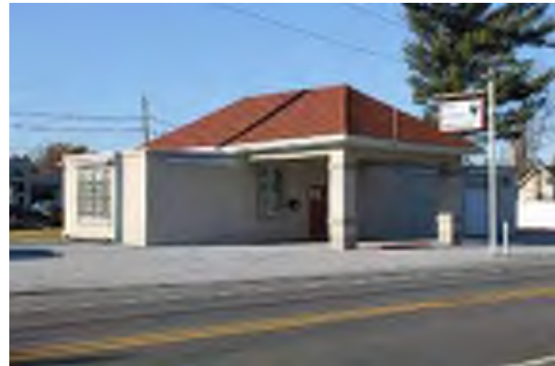
Photograph 84: 1250 Broadway, Deptford Township.
