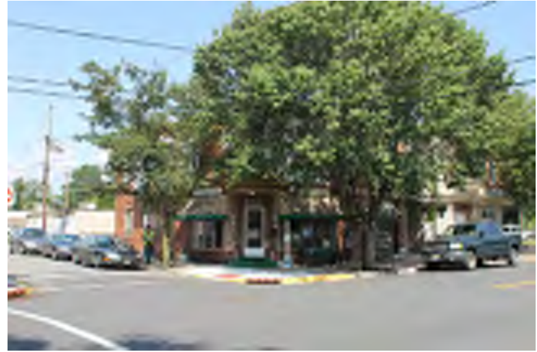
Photograph 138: Monmouth Street Commercial Row, Gloucester City.
