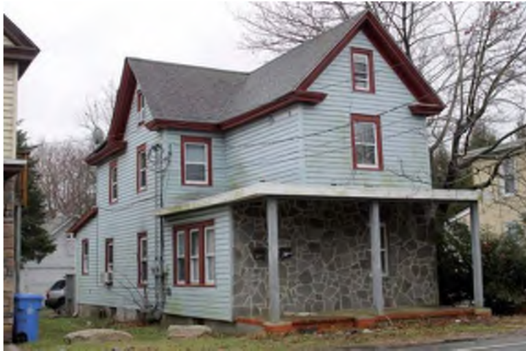
Photograph 13: 408 Ellis Street, Glassboro Borough.
