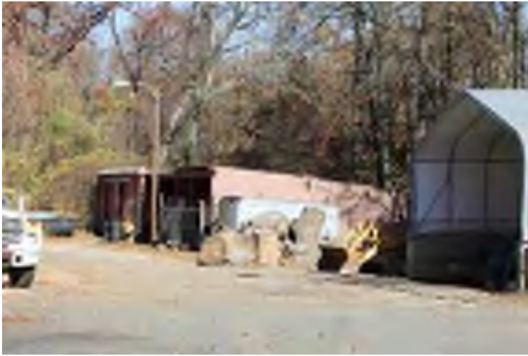
Photograph 201: W. Maple Street (Wenonah Public Works), Wenonah Borough.
