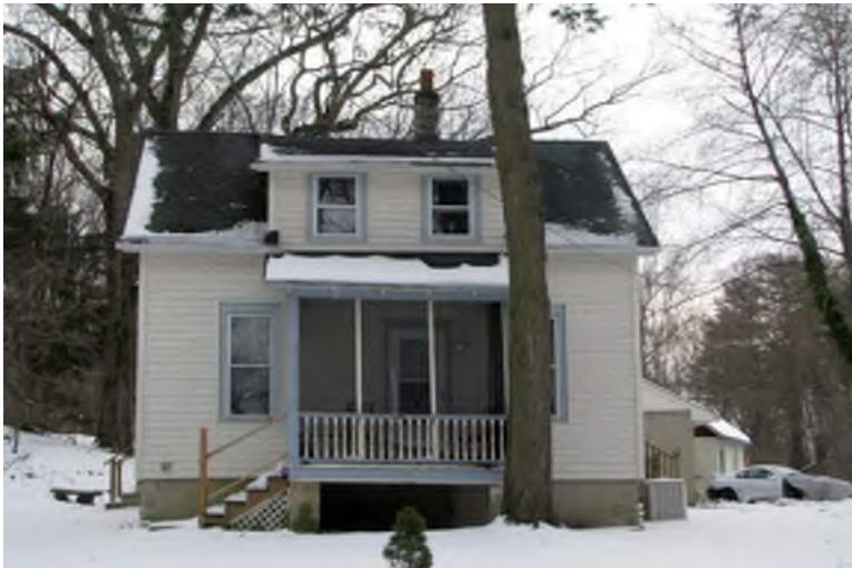
Photograph 11: 205 Bark Bridge Road, Deptford Township. View showing the primary dwelling.
