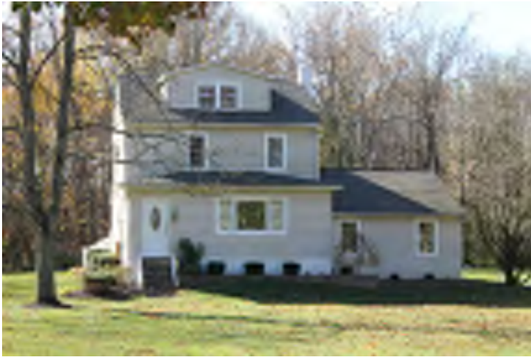
Photograph 273: 562 Chestnut Avenue, Woodbury Heights Borough.
