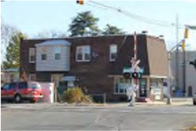
Photograph 245: 25 Olive Street, Westville Borough.
