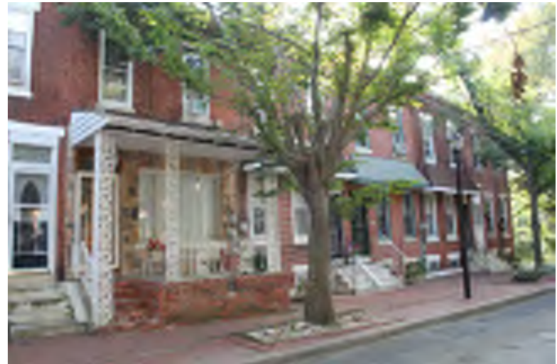
Photograph 76: Trenton Avenue Rowhouses (west of S. 9th Street), Camden City.
