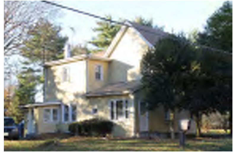
Photograph 90: 116 Buck Road, Elk Township.
