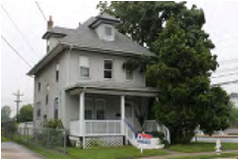
Photograph 265: 92 Wallace Street, Woodbury City.
