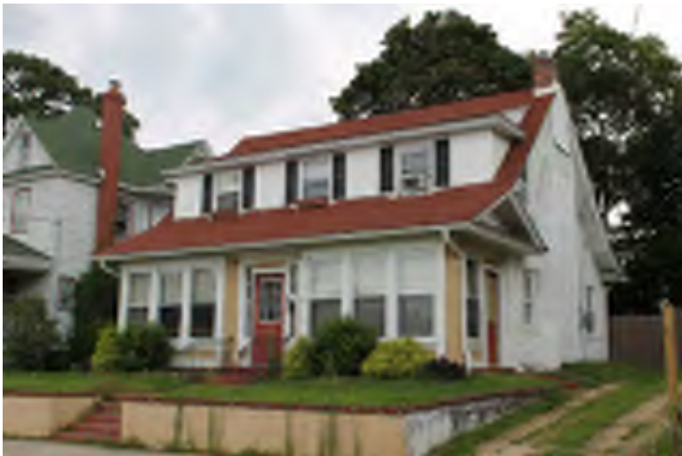
Photograph 199: Simpson Avenue Residential Streetscape, Pitman Borough. View looking northeast to 51 Simpson Avenue.
