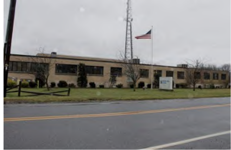
Photograph 18: 428 Ellis Street (Atlantic City Electric), Glassboro Borough.
