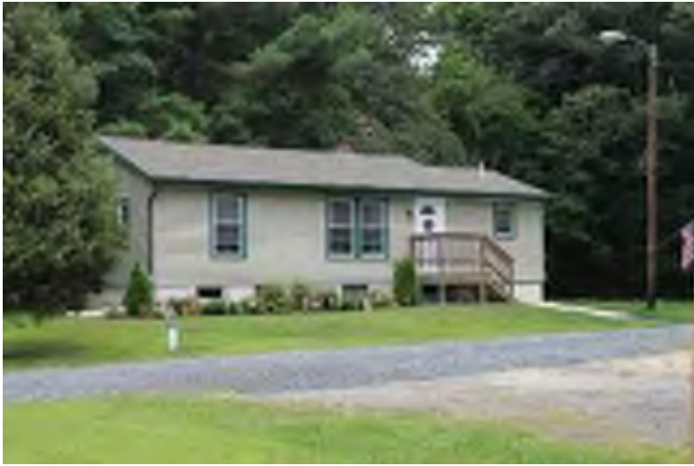
Photograph 93: 121 Buck Road, Elk Township.
