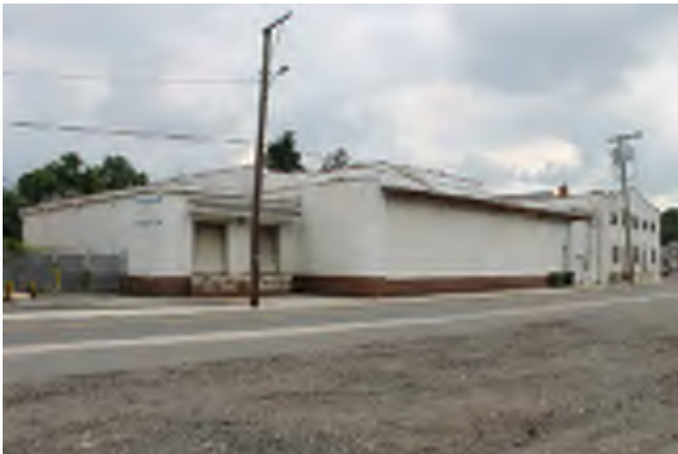
Photograph 179: 55 Commerce Avenue (Riley/Fay Sales Company Milk, Ice, and Cold Storage), Pitman Borough. View of west (front) and north (side) elevations.
