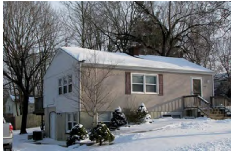
Photograph 42: 402 Yale Road N., Glassboro Borough.
