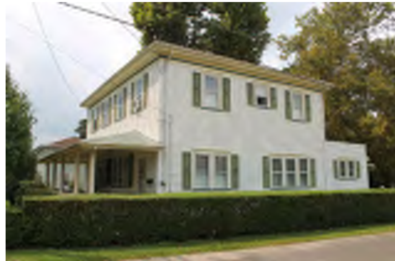
Photograph 164: 200-202 Center Street, Sewell, Mantua Township.
