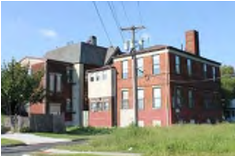
Photograph 7: Jesse Starr School (NR eligible), 823 Pine Street, Camden City. View of north (rear) and east (side) elevations, showing alterations.
