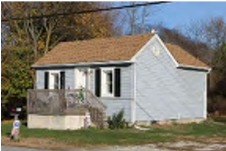
Photograph 95: 151 Buck Road, Elk Township.
