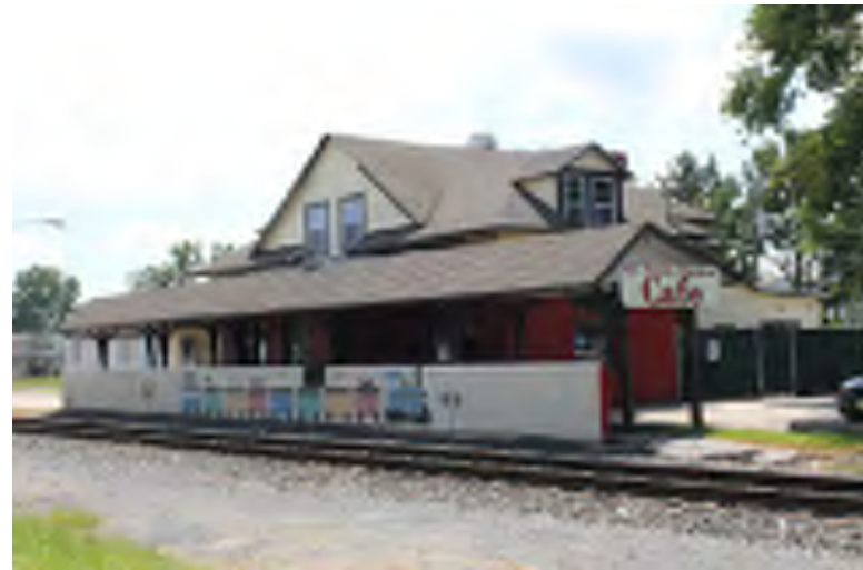
Photograph 136: 701 Monmouth Street (Gloucester City Train Station), Gloucester City. View of north (side) and east (front) elevations.
