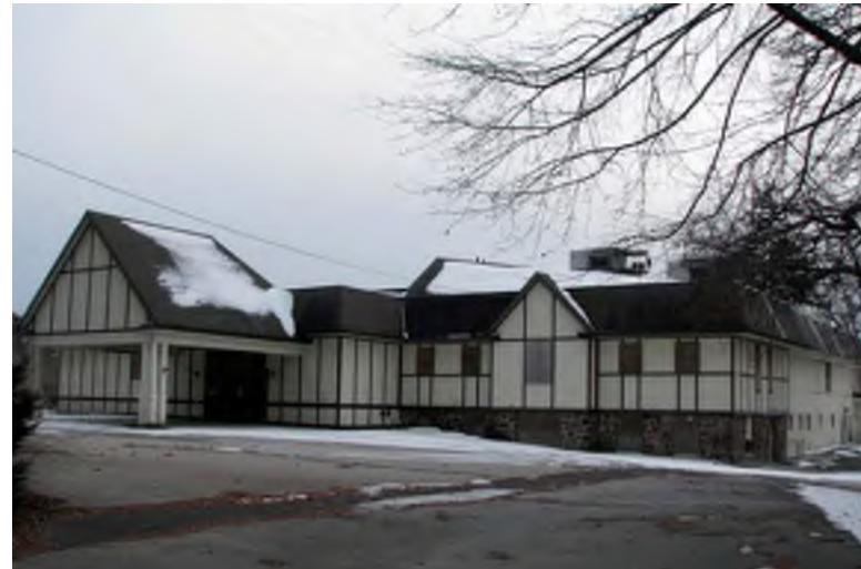
Photograph 72: 467 Cooper Street (former Woodbury Country Club), Woodbury City. The Woodbury Country Club was founded in 1897, using an 18th-century farmhouse as the clubhouse. The clubhouse has been completely engulfed with additions and there are no other extant buildings from the late 19th to mid-20th centuries.
