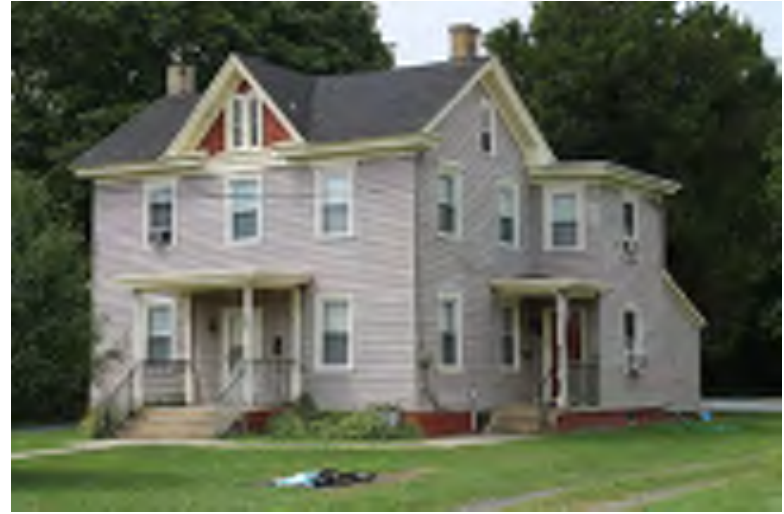
Photograph 102: Glassworks Residential District/South Glassboro, Glassboro Borough. View looking southwest toward 29 Academy Street within the potential district.
