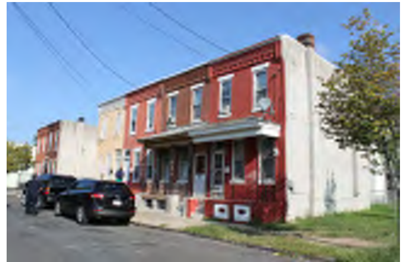
Photograph 60: Line Street Rowhouses (north-side, west of S. 9th Street), Camden City.
