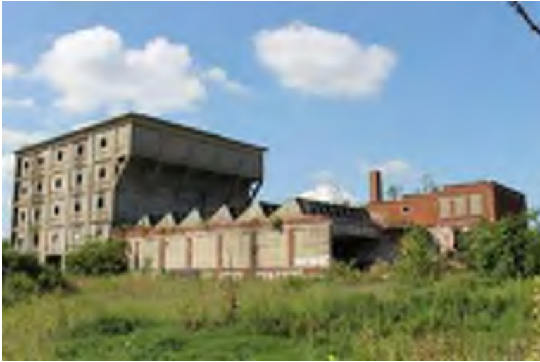
Photograph 69: Railroad Avenue/S. 7th Street at Kaighns Avenue (Farr & Bailey Manufacturing Company/Congoleum Nairn Company) Linoleum Plant, Camden City. View looking south from Kaighns Avenue.
