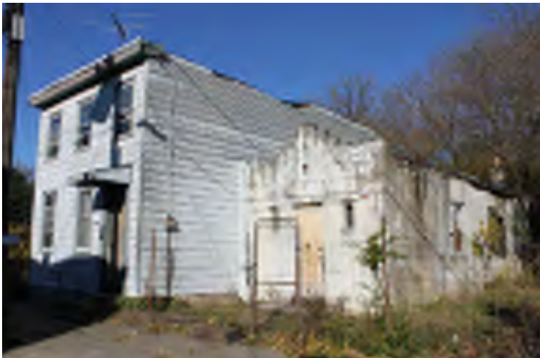
Photograph 63: 817 Mt. Vernon Street, Camden City.
