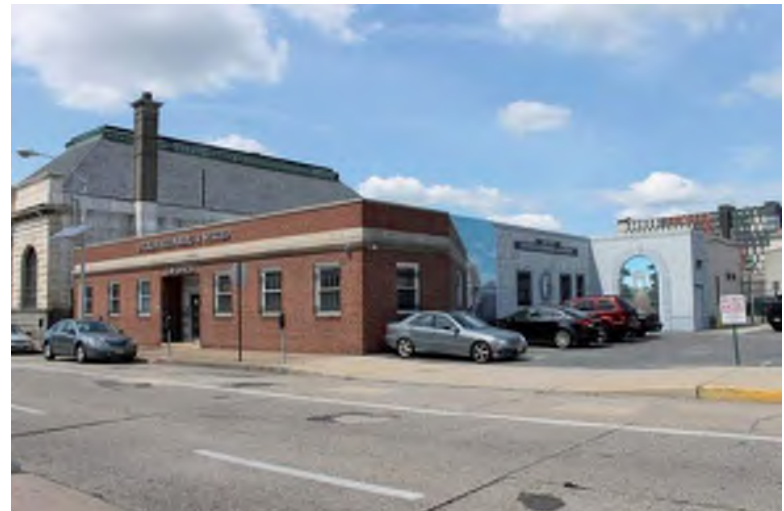
Photograph 4: 415 Federal Street, Camden City.
