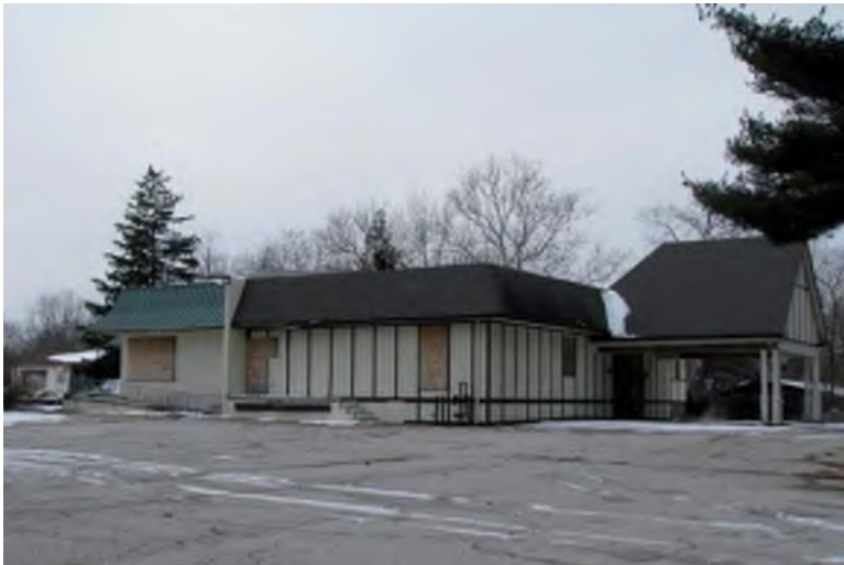
Photograph 71: 467 Cooper Street (former Woodbury Country Club), Woodbury City. The Woodbury Country Club was founded in 1897, using an 18th-century farmhouse as the clubhouse. The clubhouse has been completely engulfed with additions and there are no other extant buildings from the late 19th to mid-20th centuries.
