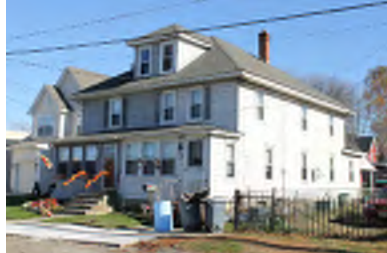
Photograph 28: 3-5 Railroad Lane, Brooklawn Borough.
