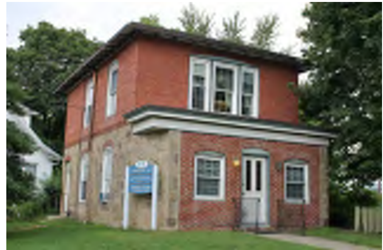
Photograph 196: 55 Simpson Avenue (Fire Company No. 1), Pitman Borough.
