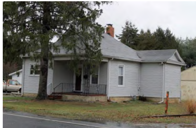
Photograph 16: 418 Ellis Street, Glassboro Borough.
