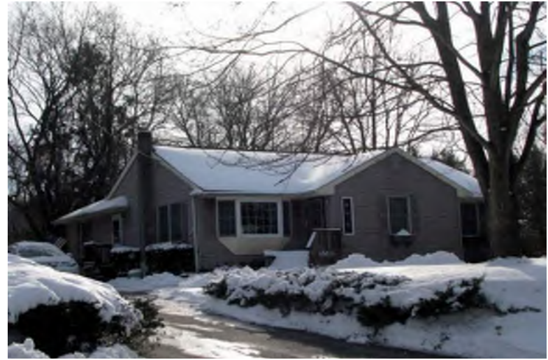
Photograph 62: 360 Tylers Mill Road, Mantua Township.
