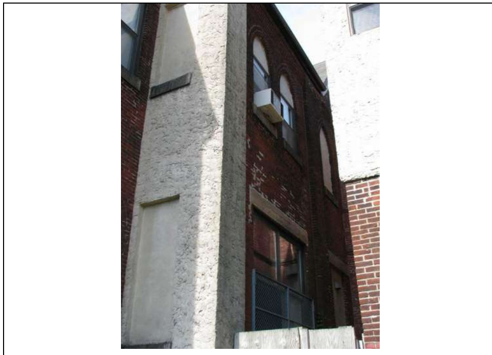
Photograph 5: Partial view of the east (side) and north (rear) elevations of the original 1888 to 1889 building. Looking southwest (May 2014).
