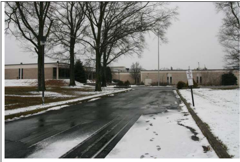
Photograph 8: Northeast elevation (side) of Blocks A on the right and B on the left. Looking southwest (January 2019).
