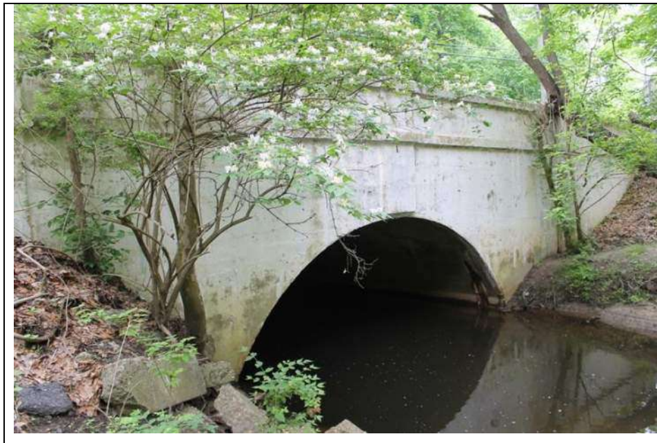
Photograph 5: North (downstream) elevation prior to the rehabilitation. Looking southwest. Note the barrel arch (May 2014).
