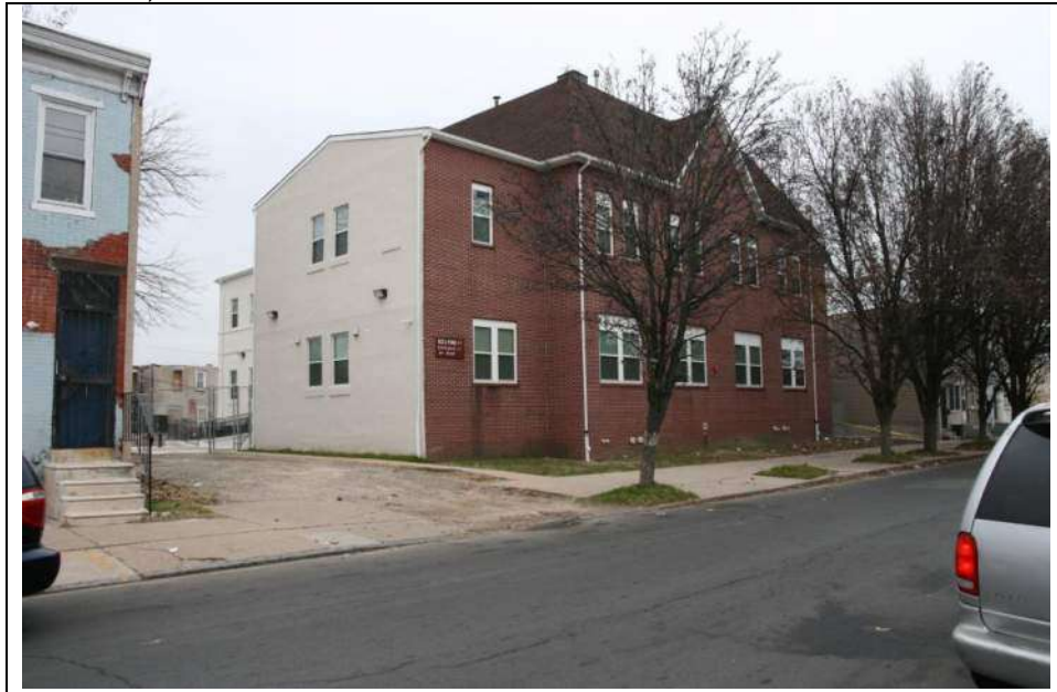
Photograph 1: West (side) and south (front) elevations of Jesse Starr School at 823 Pine Street. Looking northeast (December 2018).
