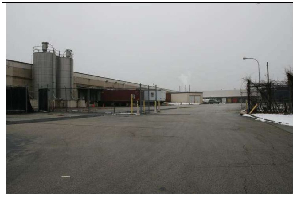
Photograph 15: Southwest elevation of Block C and north elevation of Block E. Looking southeast (January 2019).
