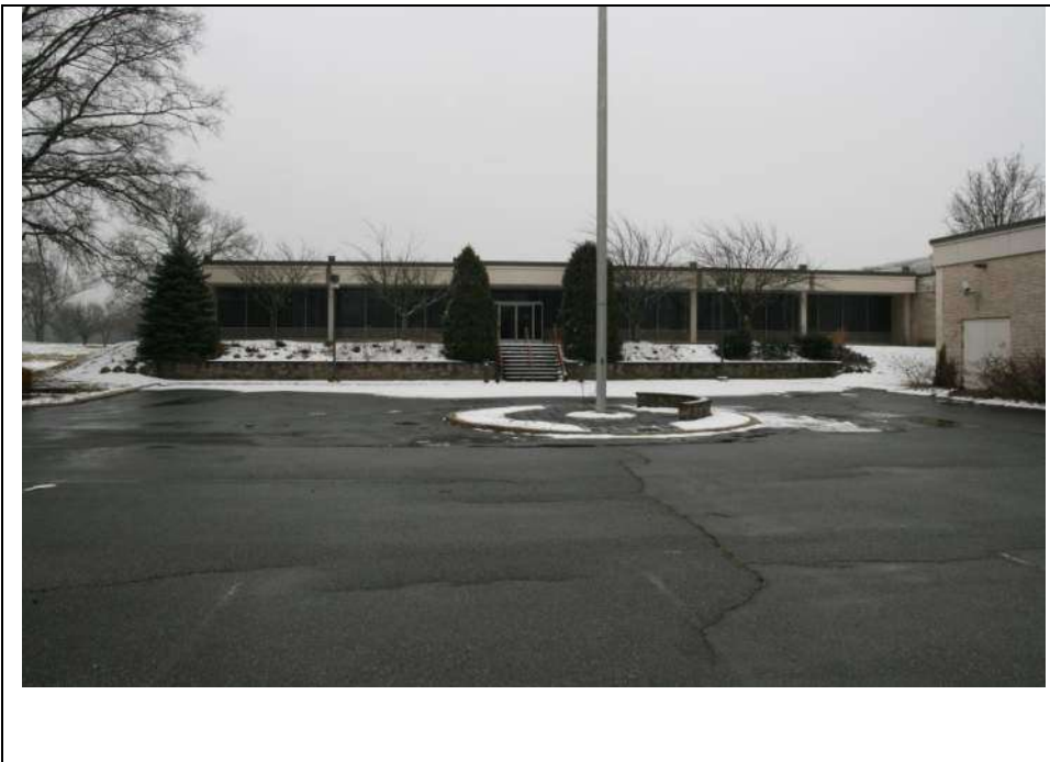
Photograph 7: Northwest elevation (façade) entrance of Block B. Note Block A is visible on the right. Looking southeast (January 2019).
