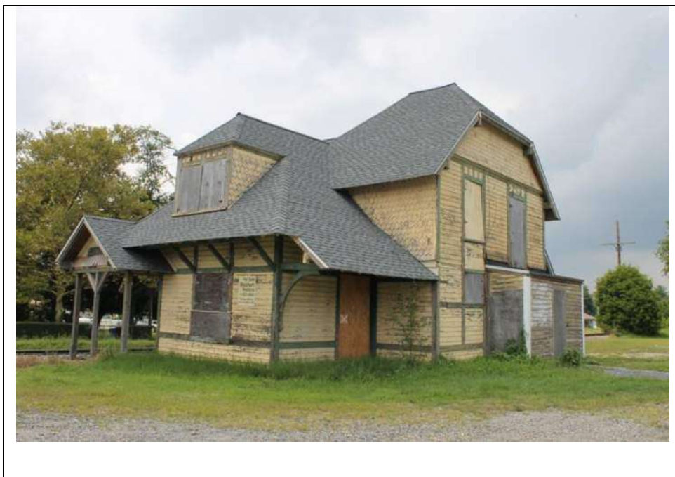
Photograph 5: Southeast (side) and northeast (rear) elevations of the Sewell Train Station, looking west (August 2013).
