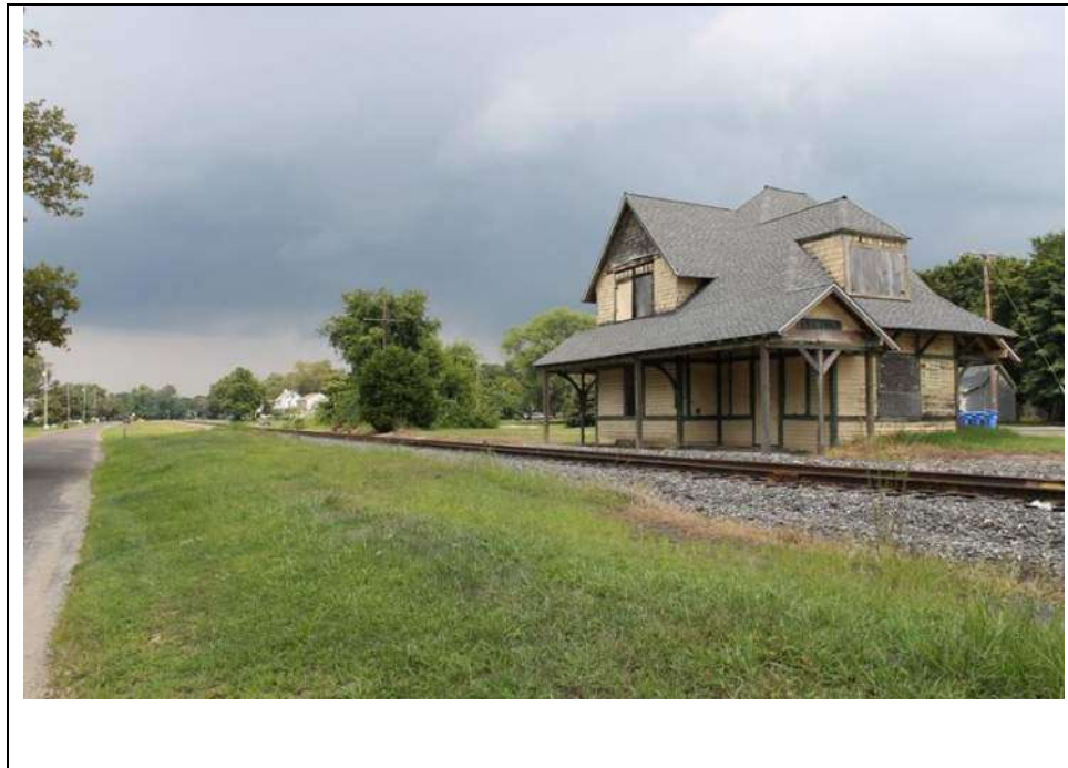
Photograph 2: Overview of the Sewell Train Station property, looking northwest from the intersection of W. Atlantic Avenue and Center Street. Note the proximity to the former West Jersey Railroad Main Line track (currently in operation as Conrail's Vineland Secondary Track; August 2013).
