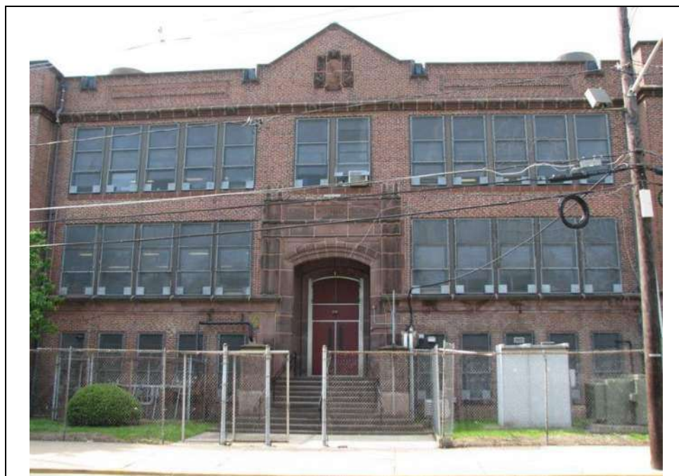
Photograph 3: Central bays of the north elevation (façade), looking south (May 2014).
