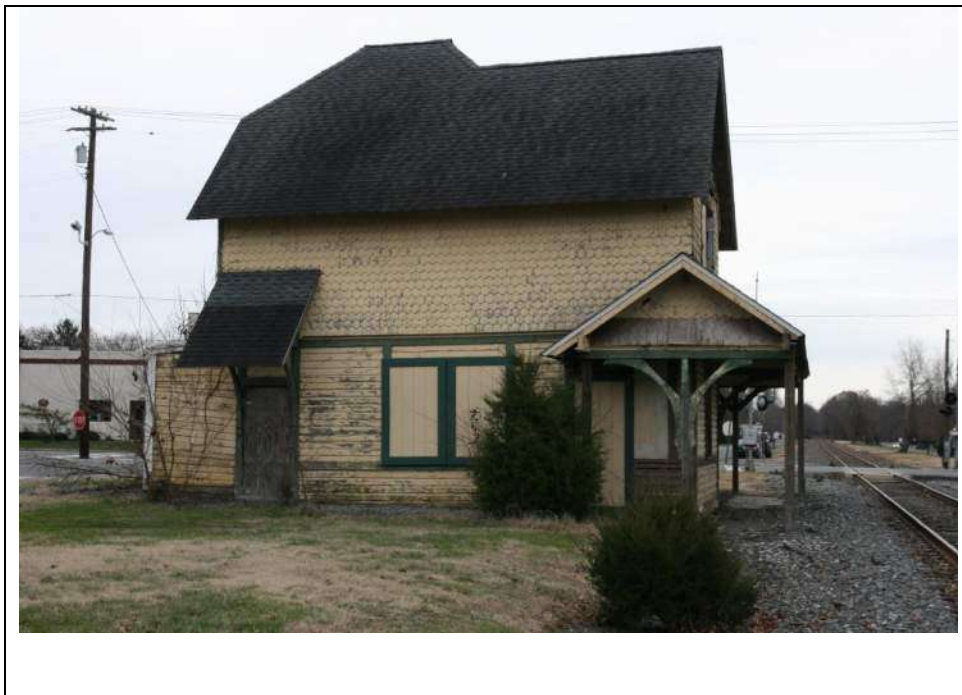
Photograph 4: Northwest (side) elevation of the Sewell Train Station, looking southeast (November 2018).
