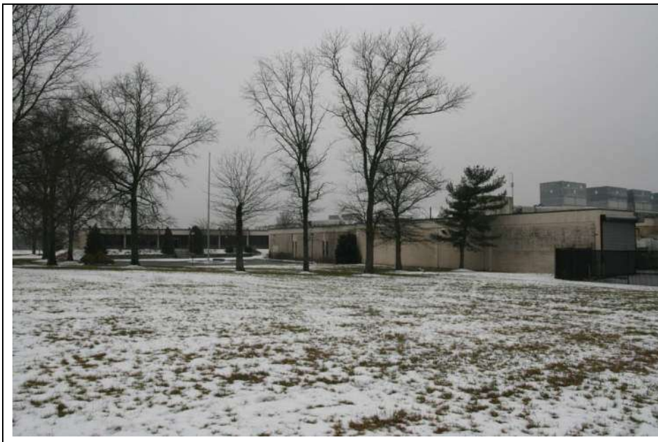
Photograph 10: Northwest (façade) elevation of Block B. Northeast elevation of Block A on the right. Note Block A's garage is also visible on the right, next to the north elevation of Block G. Looking southwest (January 2019).
