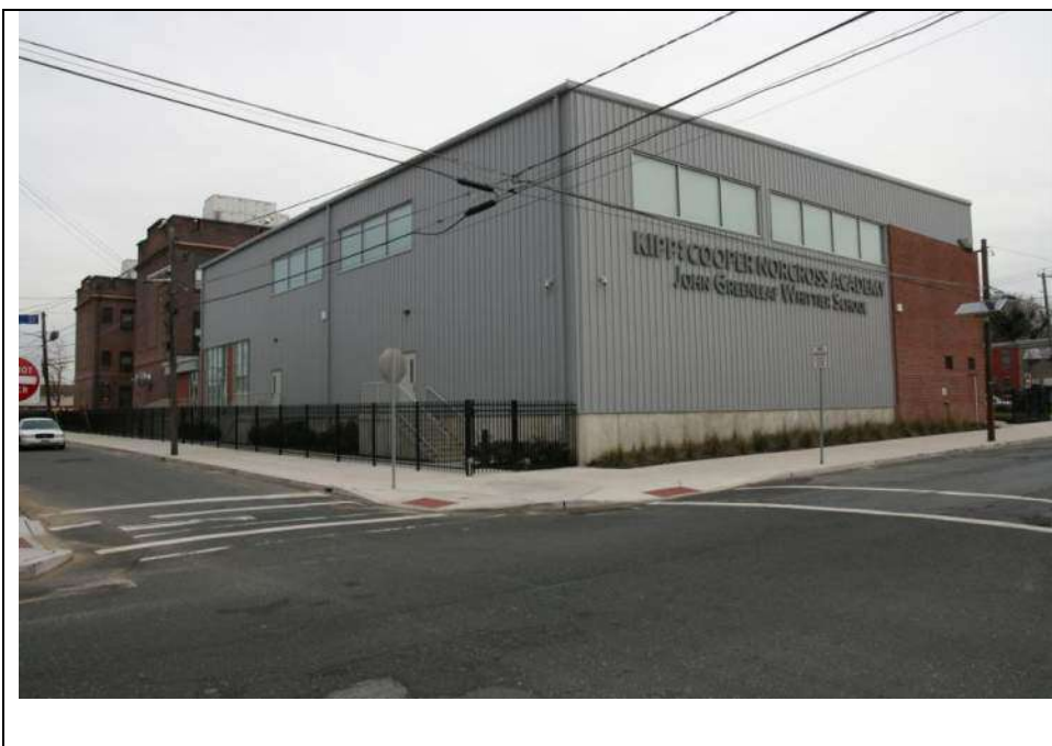
Photograph 13: South (rear) and east (side) elevations of the 2017 gymnasium, looking northwest (December 2018).
