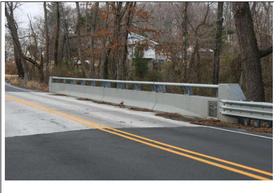
Photograph 3: North parapet. Looking northwest (December 2018).
