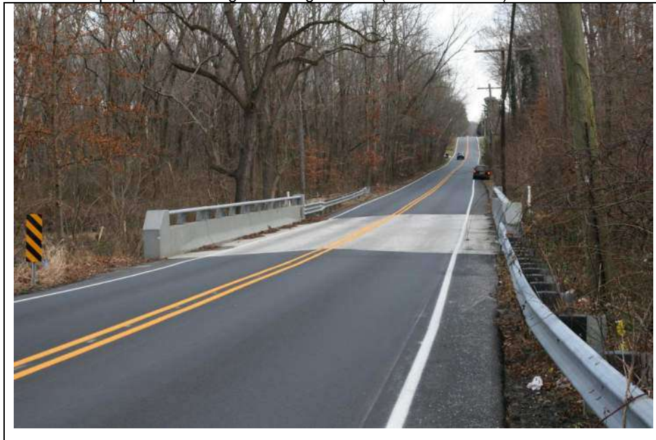
Photograph 1: Overview of the Tylers Mill Road Bridge over Chestnut Branch, looking southeast from the west end. Note the recently replaced concrete parapets with integral metal guiderails (December 2018).
