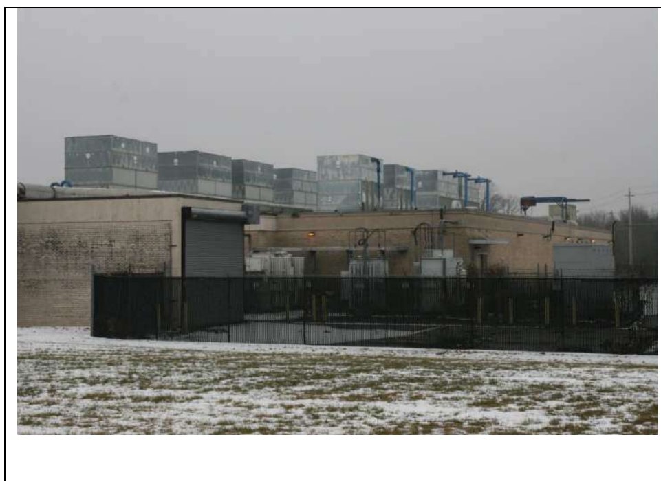
Photograph 11: Northwest elevation of Block G, note Block A's garage on the left. Looking southwest (January 2019).
