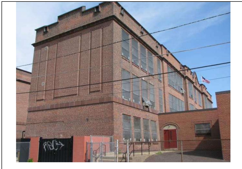
Photograph 7: East (side) elevation of the original 1910-11 building section (right-background), and south (rear) and east (side) elevations of a 1922 rear classroom wing (left-foreground; this is the eastern of the two rear wings). A portion of the 1922 gymnasium addition is visible at right-foreground. Looking northwest (May 2014).
