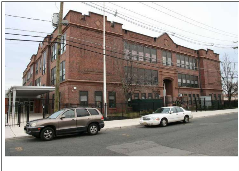
Photograph 2: East (side) and north (façade) elevations of the original 1910-11 section of the John G. Whittier School at 740 Chestnut Street, looking southwest (December 2018).
