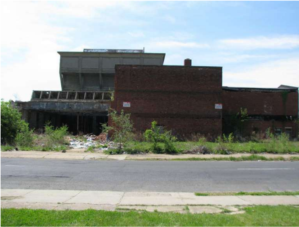
May 2014 photo of Farr & Bailey Manufacturing Company, looking south from Kaighn Avenue.
