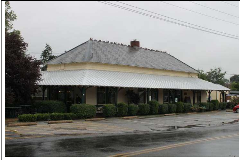
Photograph 8: Woodbury Train Station (1883), located at 101 Cooper Street, Woodbury City, Gloucester County. This former West Jersey Railroad train station exhibits Stick stylistic influences. The building has been converted to a café. Looking southeast (August 2013).
