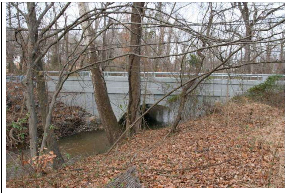
Photograph 7: South (upstream) elevation. Looking northwest (December 2018).
