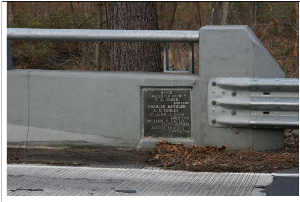
Photograph 8: Detail view of inscribed concrete bridge plaque located in the south face of the south parapet (moved from original location during rehabilitation). Looking northeast (December 2018).
