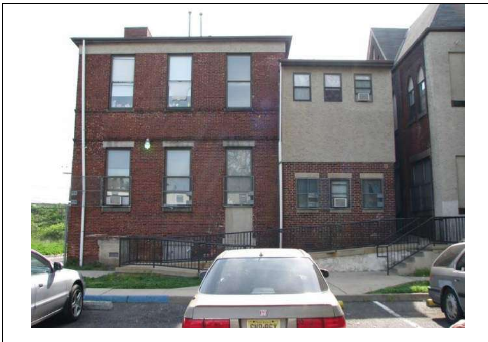
Photograph 3: West elevations of the circa -1900 rear addition (left) and one of the two circa -1994 additions (right). The north (rear) elevation of the original 1888-89 building is partially visible as well (far right). Looking east (May 2014).
