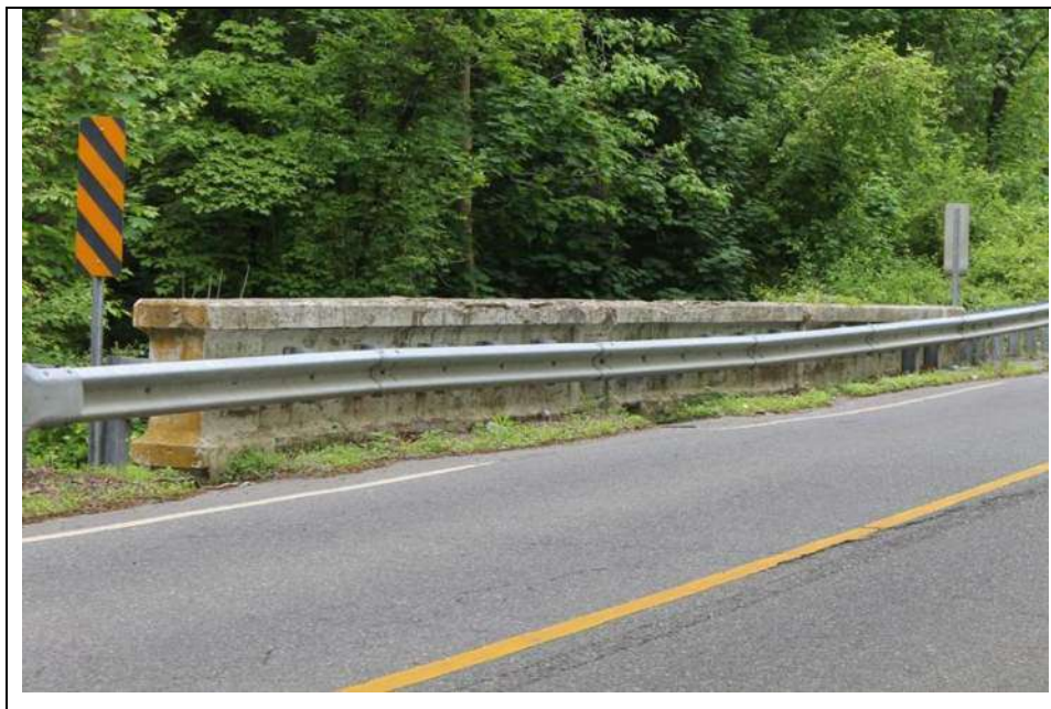
Photograph 4: South parapet and guiderail prior to the rehabilitation. Looking west (May 2014).
