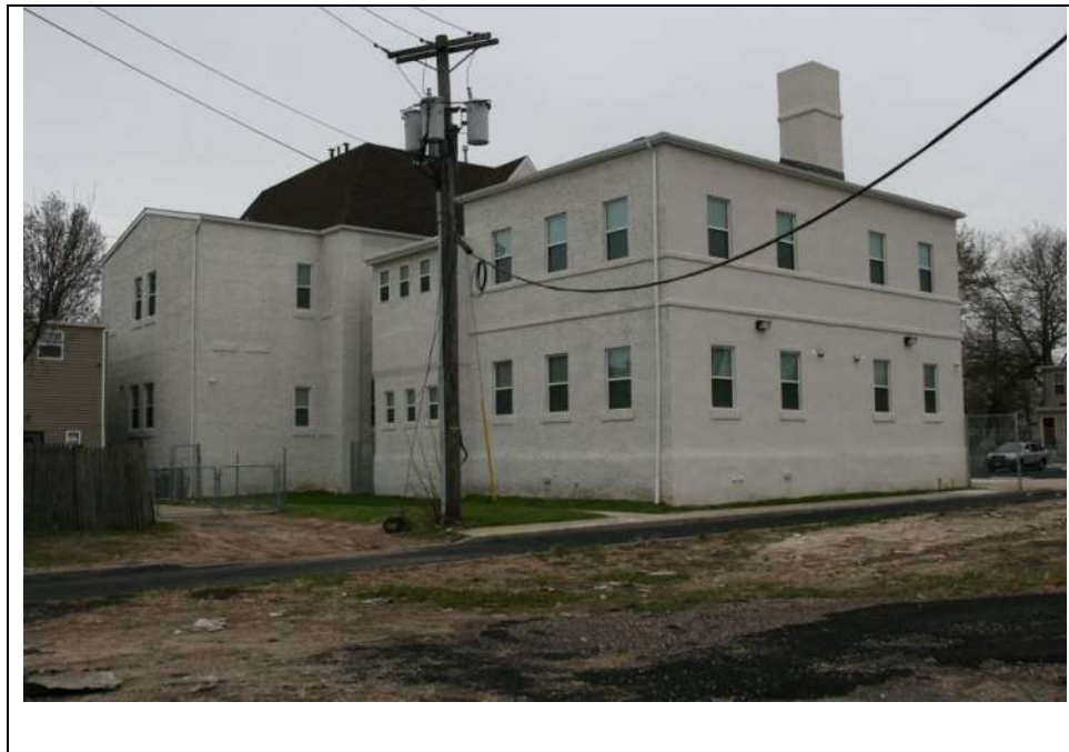
Photograph 4: East (side) and north (rear) elevations. The original (1888 to 1889) building is visible at left, the circa -1900 rear addition is shown at right, and one of the two circa -1994 additions is visible in the center. Looking southwest (December 2018).
