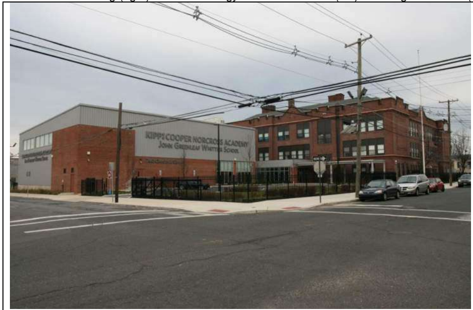
Photograph 1: Overview of the John G. Whittier School at 740 Chestnut Street, showing the east (side) and north (front) elevations of the 1910-11 main building (right) and the 2017 gymnasium addition (left). Looking southwest (December 2018).
