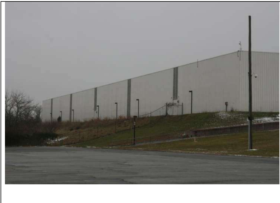
Photograph 20: Southeast (front) and northeast (side) elevation of Block E and lower parking lot. Looking northwest (January 2019).
