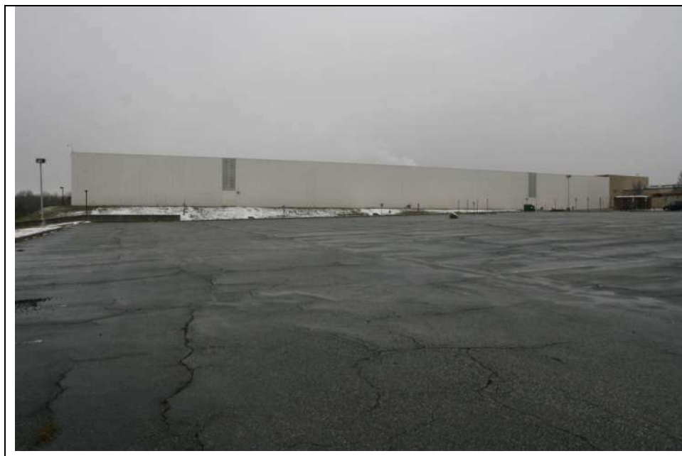
Photograph 21: Northeast elevation (side) of Block E and upper parking lot. Note the northeast elevation of block D is visible on the right. Looking southwest (January 2019).
