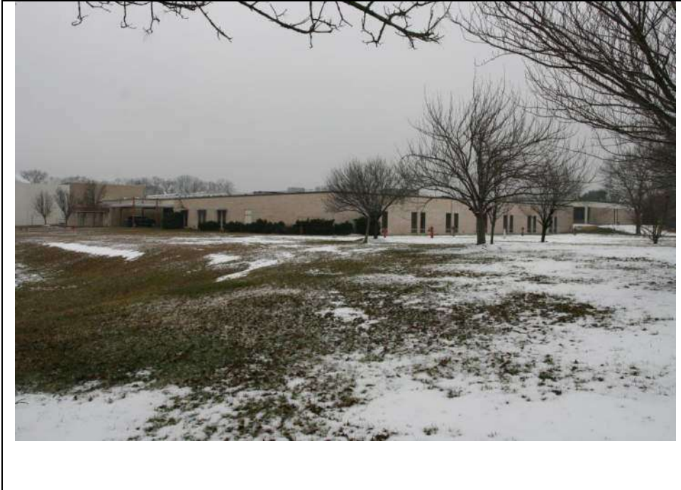
Photograph 2: Southeast (front) and northeast (side) elevations of the former Sony plant (Blocks A and F) at 400 N Woodbury Road. Looking northwest (January 2019).
