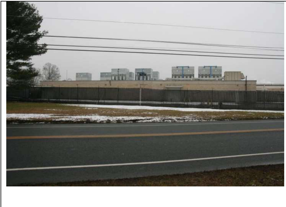
Photograph 12: Northwest elevation of Block G. Looking south (January 2019).
