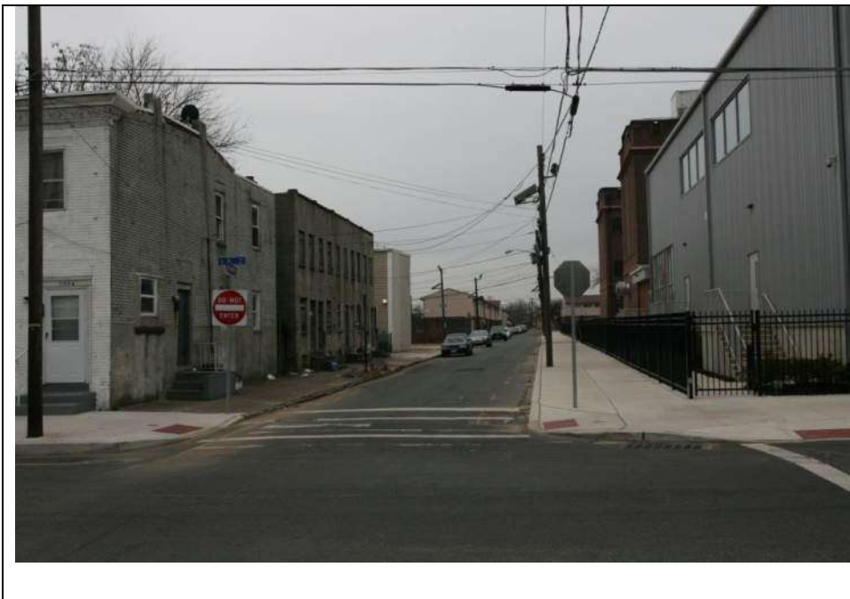
Photograph 15: Overview of the John G. Whittier School in context, looking west along Sycamore Street (December 2018).
