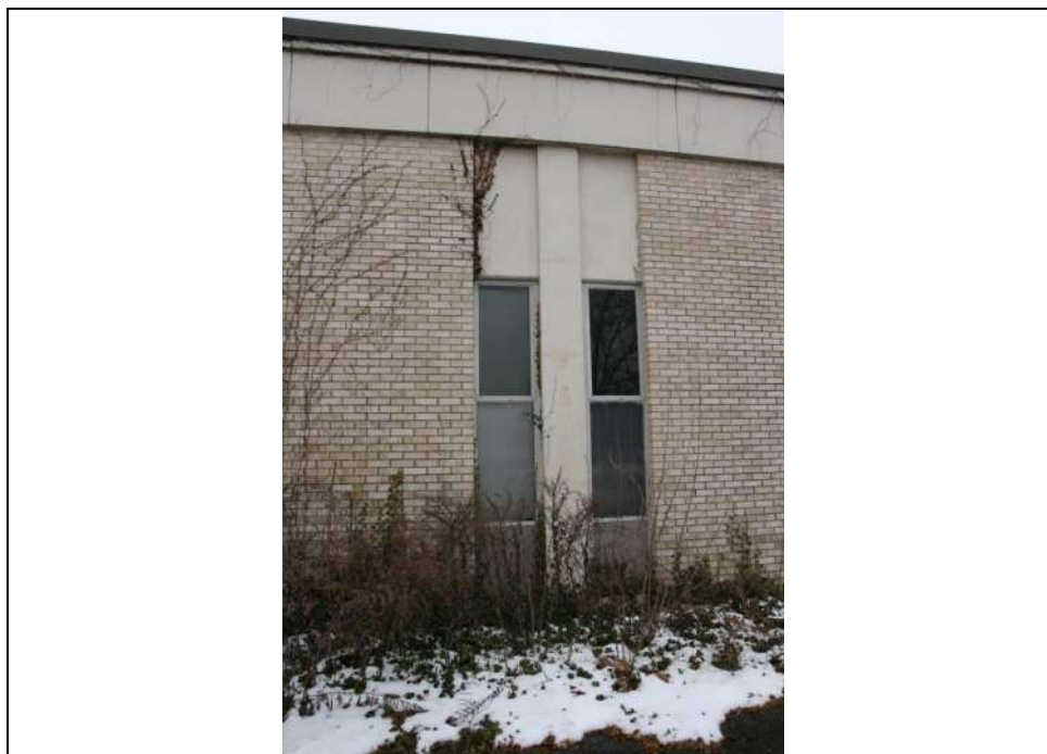
Photograph 9: Northeast elevation (side) window detail of Block A. Looking southwest (January 2019).
