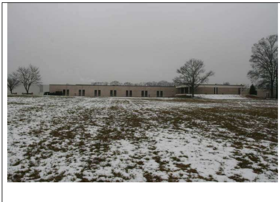
Photograph 5: Northeast elevation (side) of Blocks F on the left and Block B on the right. Note Block E is visible on the far left. Looking southwest (January 2019).
