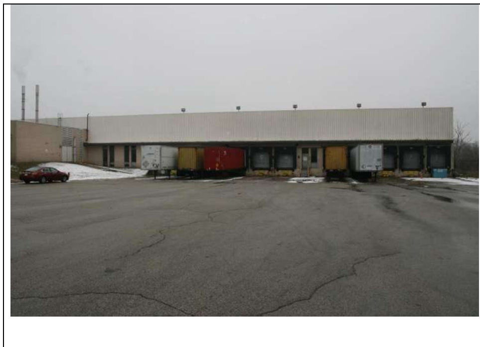
Photograph 18: Northwest elevation of Block E on the right and southwest elevation of Block D on the left. Looking southeast (January 2019).
