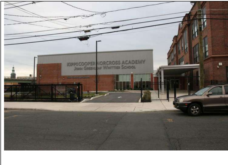
Photograph 12: North (front) elevation of the 2017 gymnasium, looking south (December 2018).
