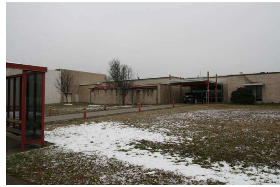
Photograph 3: Southeast elevation (façade) of Block A. Note that Block F's window is visible on the right. Looking northwest (January 2019).
