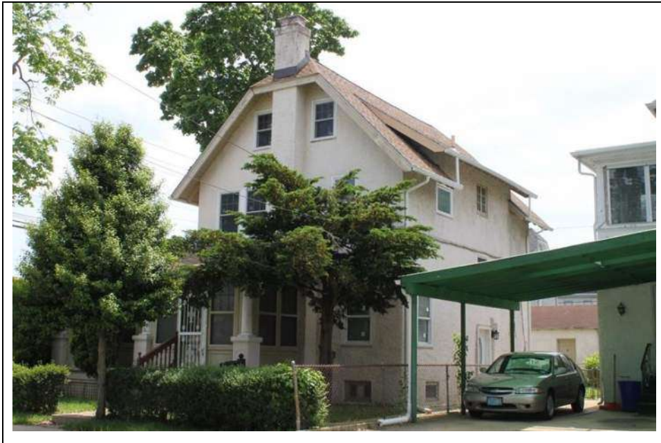
Photograph 4: Northeast (front) and northwest (side) elevations of dwelling at 85 Aberdeen Place. Looking south (May 2014).
