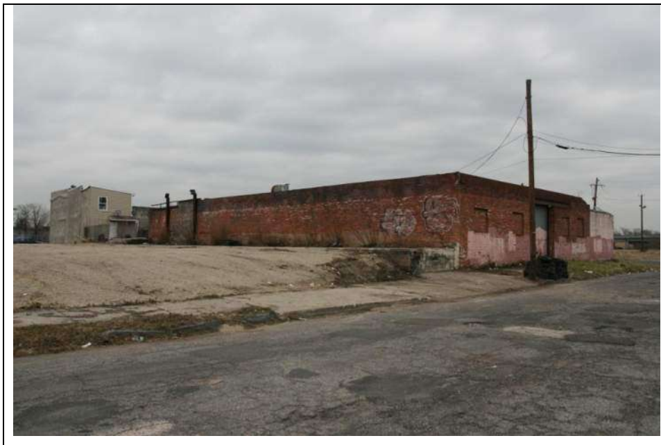
Photograph 8: West and south elevations of the brick wall enclosing the rear portion of the lot. Looking northeast (December 2018).
