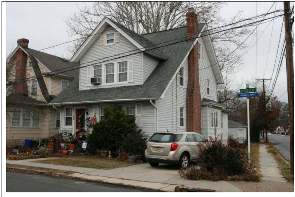
Photograph 1: Southwest (front) and southeast (side) elevations of dwelling at 86 Aberdeen Place. Looking north (November 2018).
