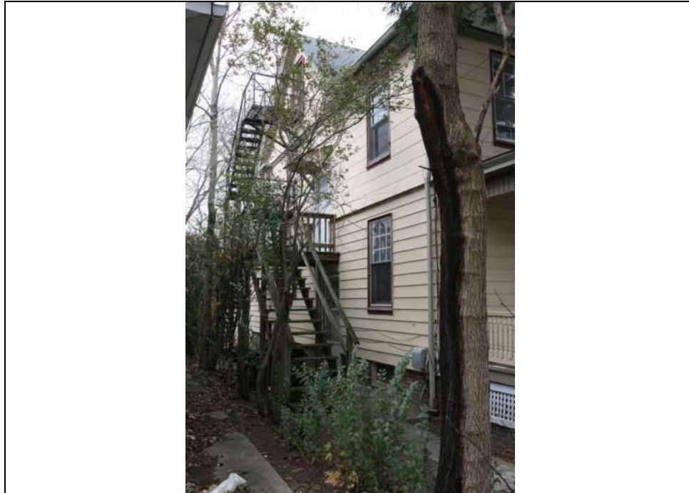
Photograph 2: Northwest (side) elevation of dwelling at 78 E. Centre Street. Looking northeast (November 2018).
