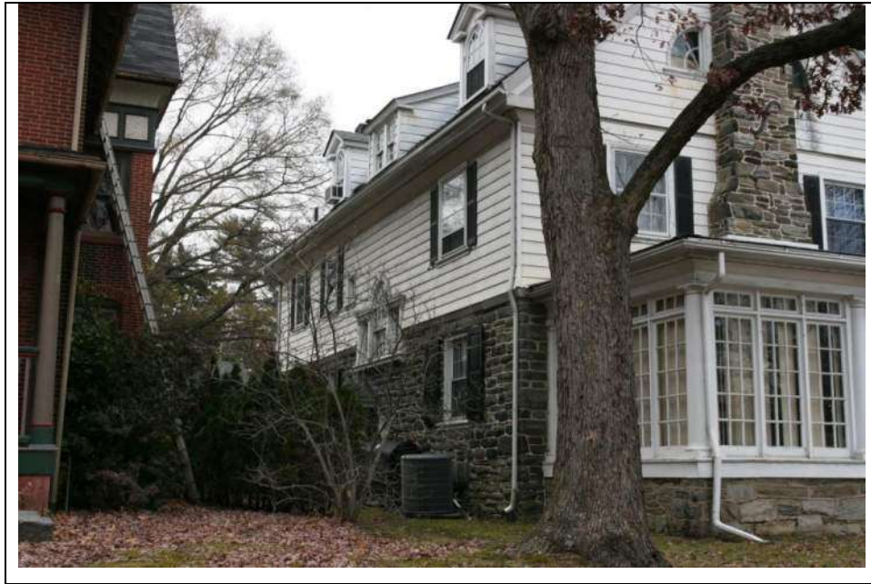
Photograph 4: South (side) and west (rear) elevations of dwelling at 7 N. Evergreen Avenue. Looking northeast (November 2018).
