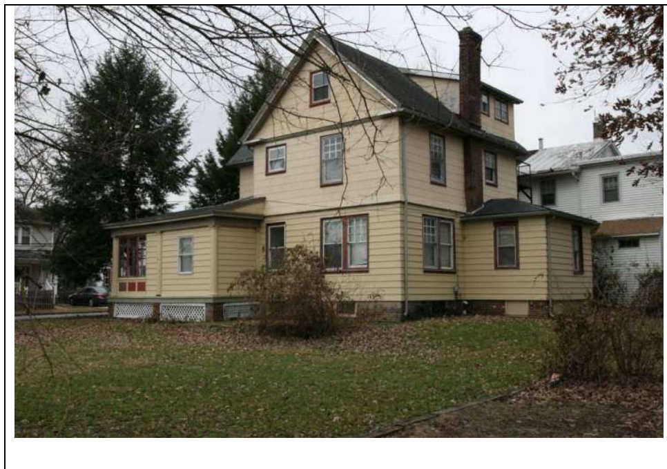
Photograph 3: Southeast (side) and northeast (rear) elevations of dwelling at 78 E. Centre Street. Looking west (November 2018).
