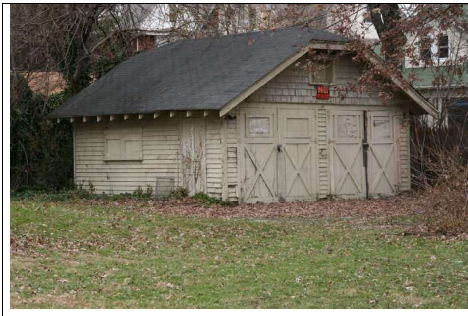
Photograph 4: Southwest (side) and southeast (front) elevations of the garage at 78 E. Centre Street. Looking north (November 2018).
