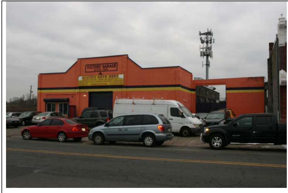
Photograph 4: View of the north (front) elevation showing the concrete wall projecting from the north end of the west (side) elevation of Victory Garage toward a neighboring residential property (just visible at right). A modern metal gate occupies the large opening in the wall. Looking southeast (December 2018).
