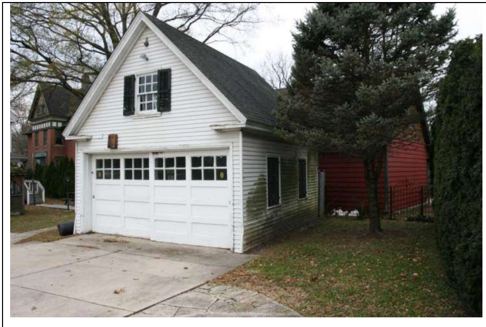
Photograph 7: East (front) and north (side) elevations of garage at 7 N. Evergreen Avenue. Looking west (November 2018).
