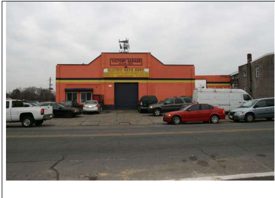
Photograph 2: North elevation (façade) of Victory Garage at 634 Kaighn Avenue. Looking south (December 2018).
