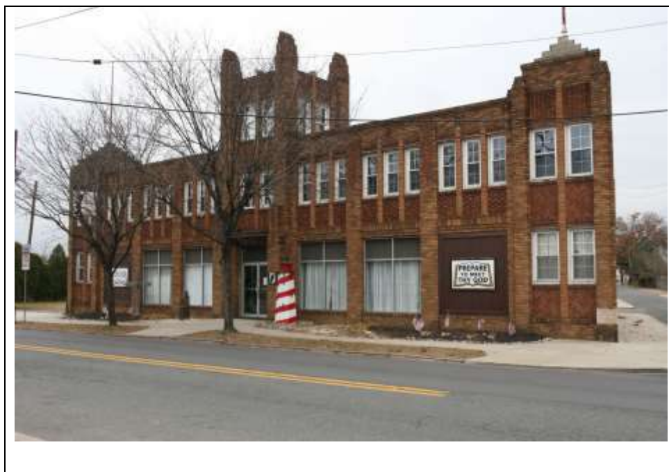
Photograph 3: South elevation (façade). Looking northwest (November 2018).
