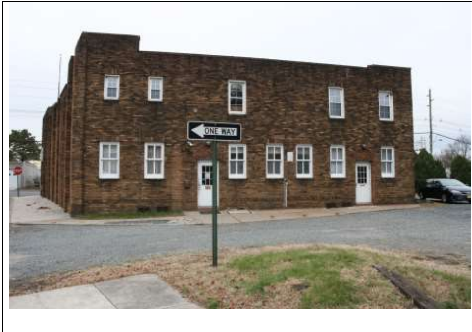
Photograph 8: North (rear) elevation. Looking southwest (November 2018).
