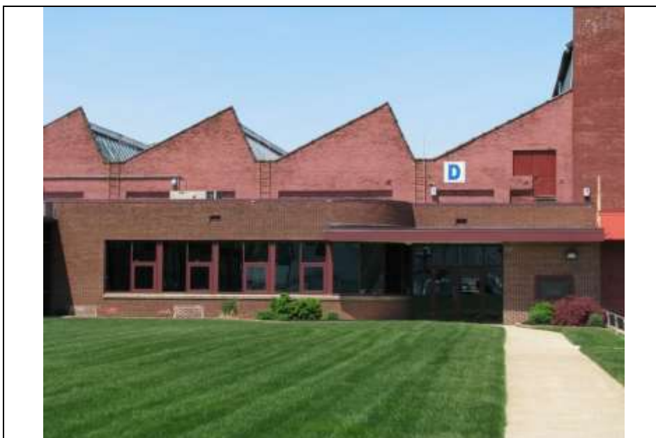
Photograph 25: Detail of southeast elevation of the circa -1967 office (Unit C). Looking northwest (May 2014).
