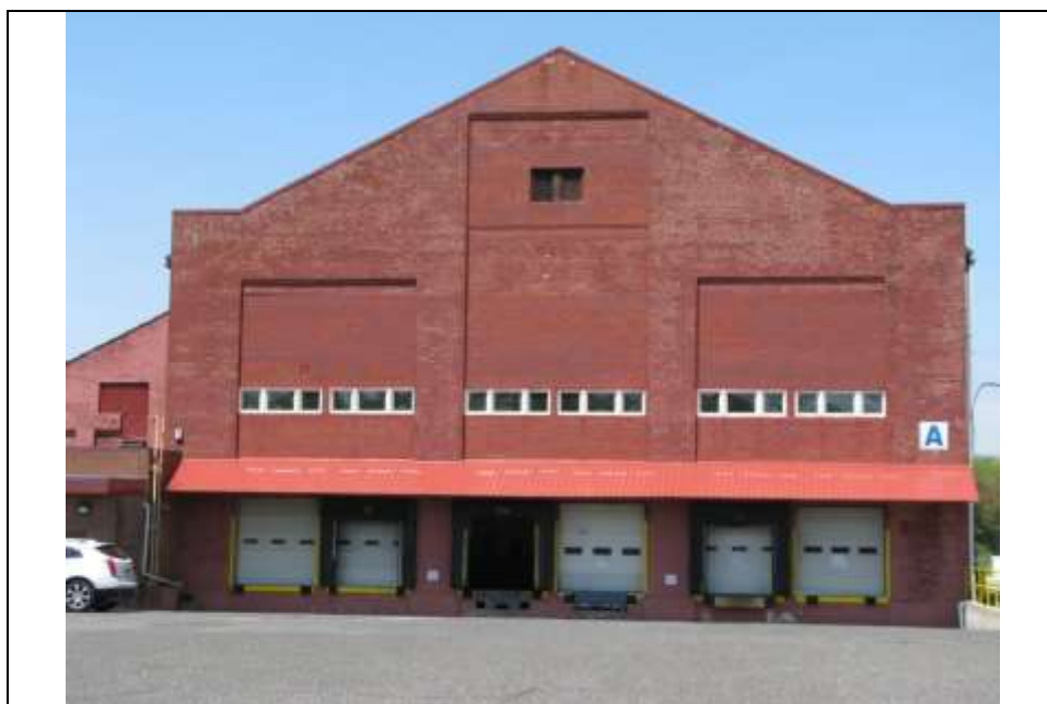
Photograph 4: Southeast elevation (façade) of the 1918 furnace room (Unit A). Looking northwest (May 2014).
