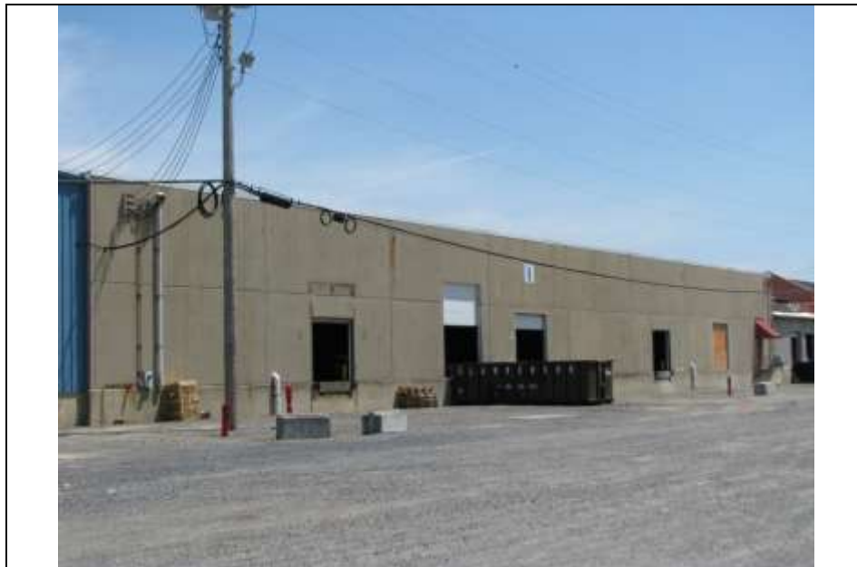
Photograph 23: Southwest elevation of the circa -1960 Unit I. Looking east (May 2014).
