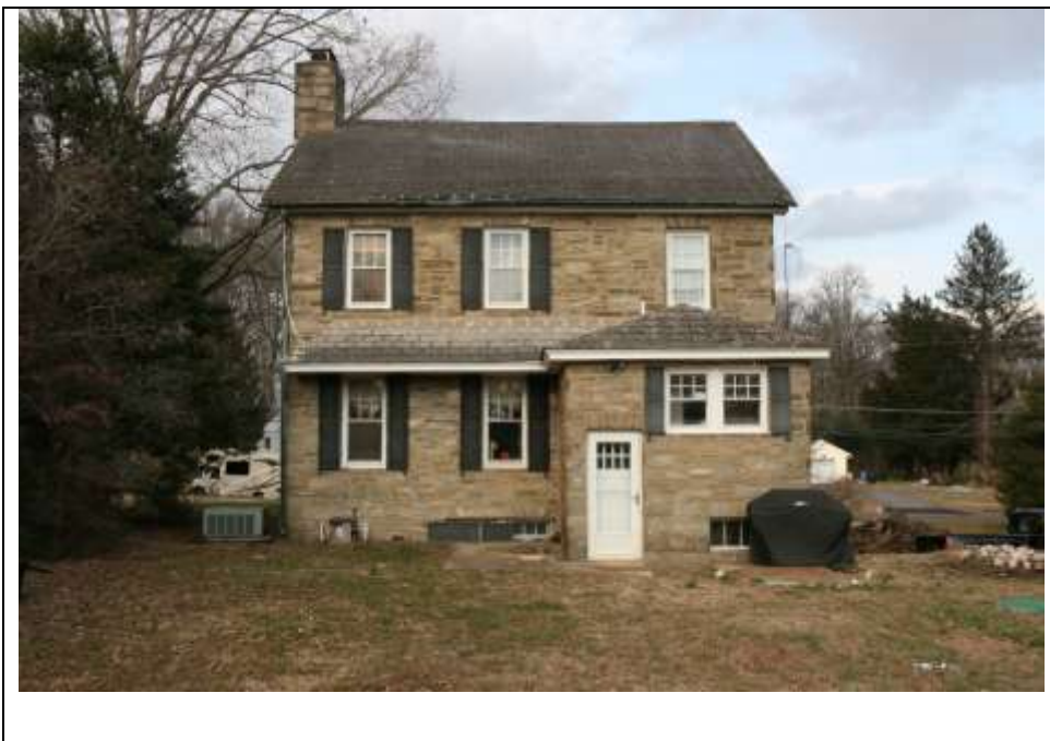
Photograph 3: Southwest (rear) elevation of dwelling at 856 Main Street. Looking northeast (December 2018).
