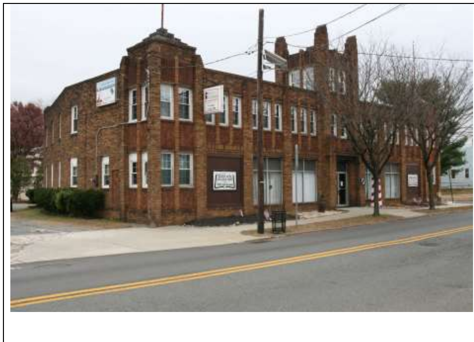
Photograph 2: West (side) and south (front) elevations of the former J.R. Quigley Company office and store at 811 Market Street. Looking east (November 2018).
