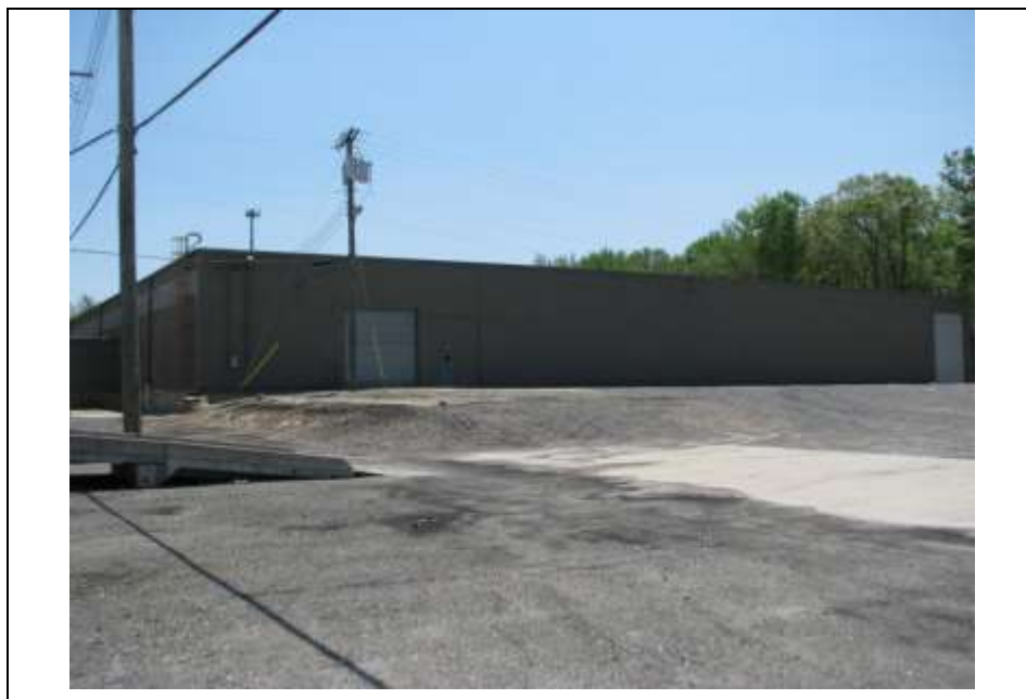
Photograph 22: Northwest elevation of the circa -1953 Unit K. Looking southeast (May 2014).
