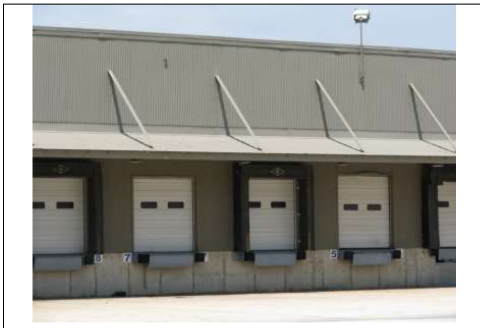
Photograph 20: Detail of southeast elevation of the circa -1953 Unit K, showing the shipping bays with modern garage doors. Looking northwest (May 2014).
