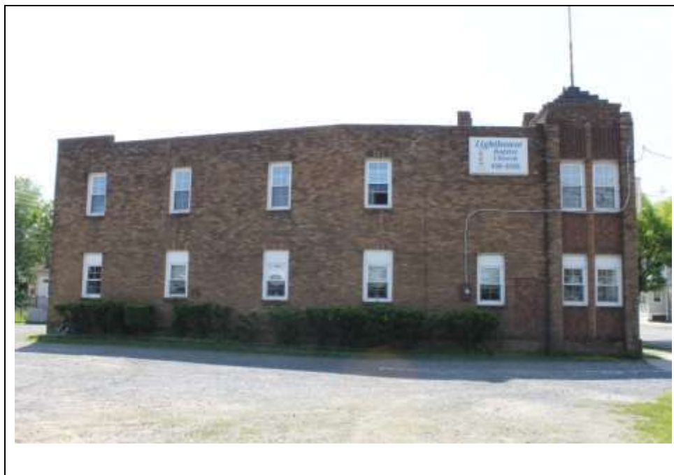
Photograph 6: West (side) elevation. Looking southeast (May 2014).
