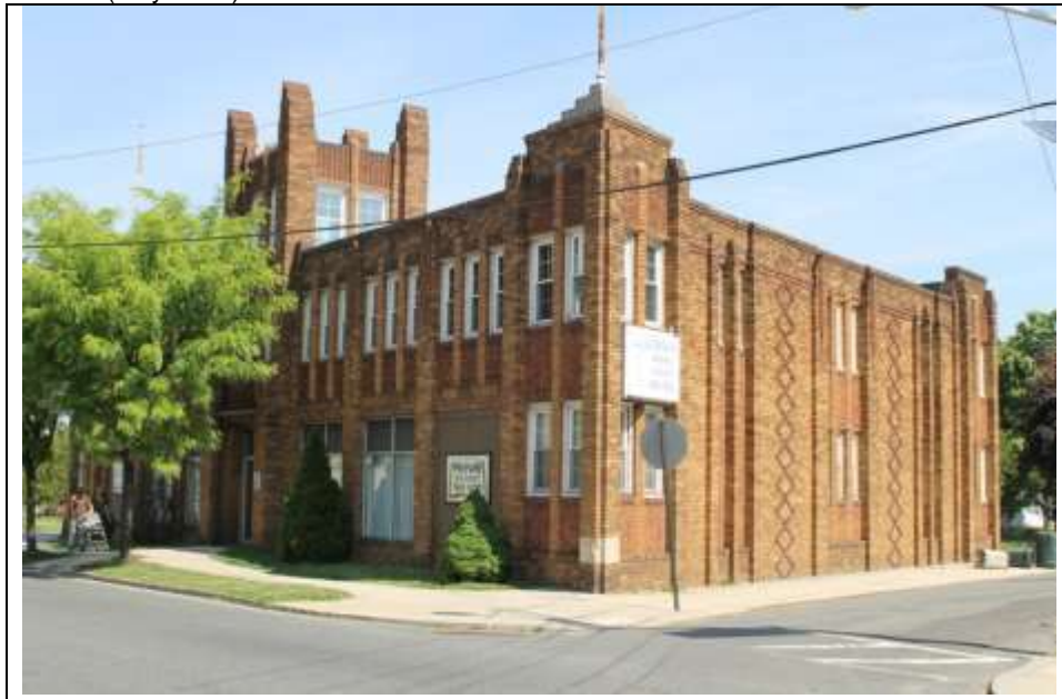
Photograph 1: South (front) and east (side) elevations of the former J.R. Quigley Company office and store at 811 Market Street. Looking northwest (May 2014).
