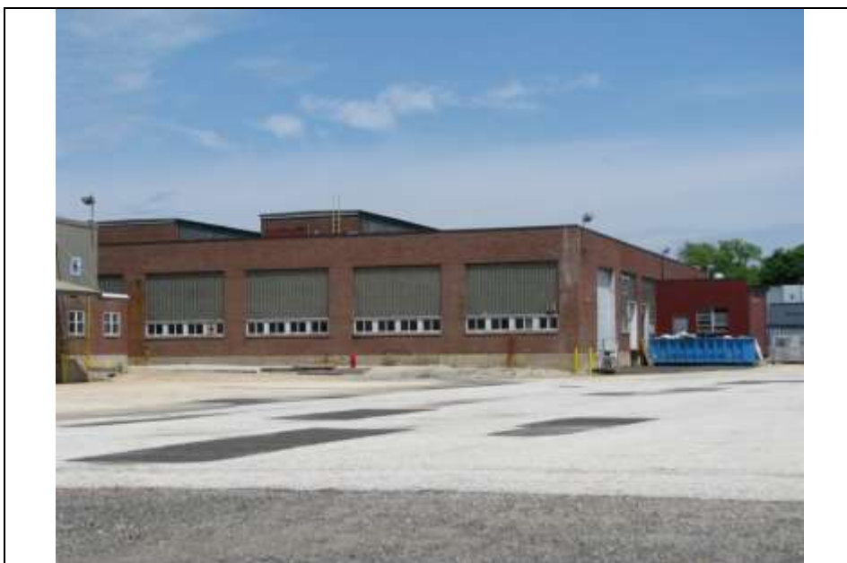
Photograph 15: Southwest and southeast elevations of the 1948 Unit F. Looking north (May 2014).
