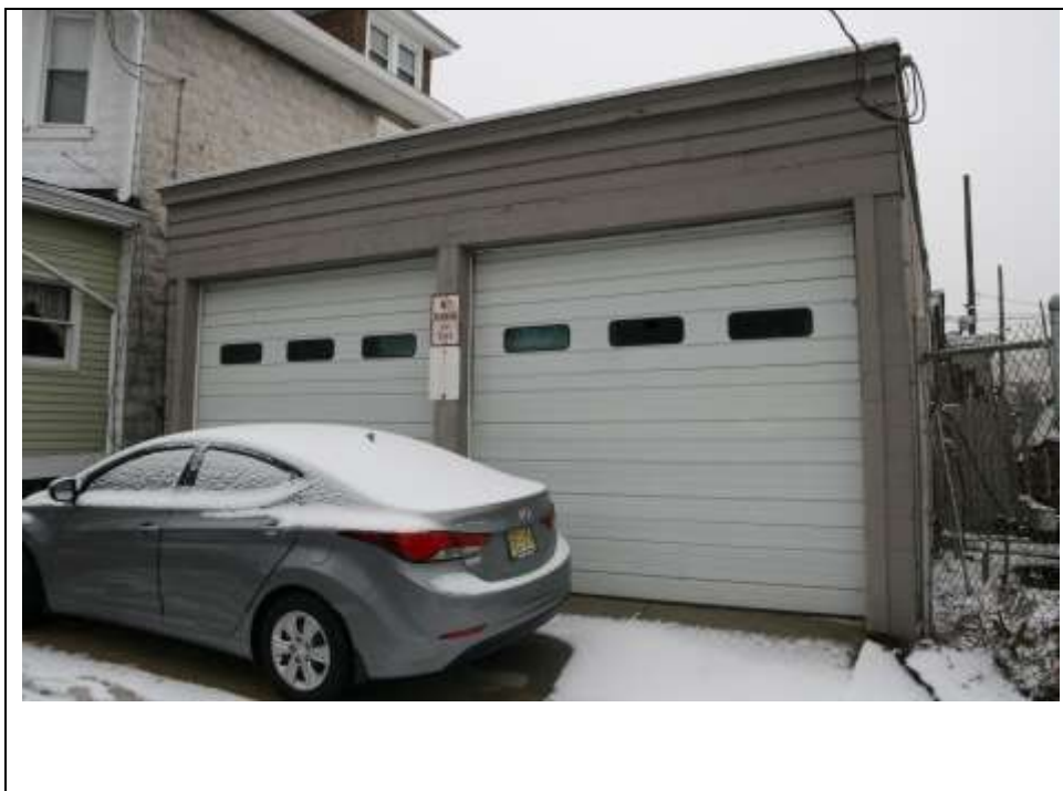
Photograph 9: Northeast (front) elevation of the Garage/Workshop. Looking southwest (January 2019).
