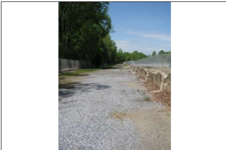
Photograph 31: Partially buried circa -1953 railroad siding located just inside the southwest property line (the rails are visible in the background). It appears that this line, which extended from the West Jersey Railroad's Bridgeton Branch, was installed to serve Unit K (ca. 1953), as it is aligned with an opening in the building's northwest elevation. Looking northwest (May 2014).
