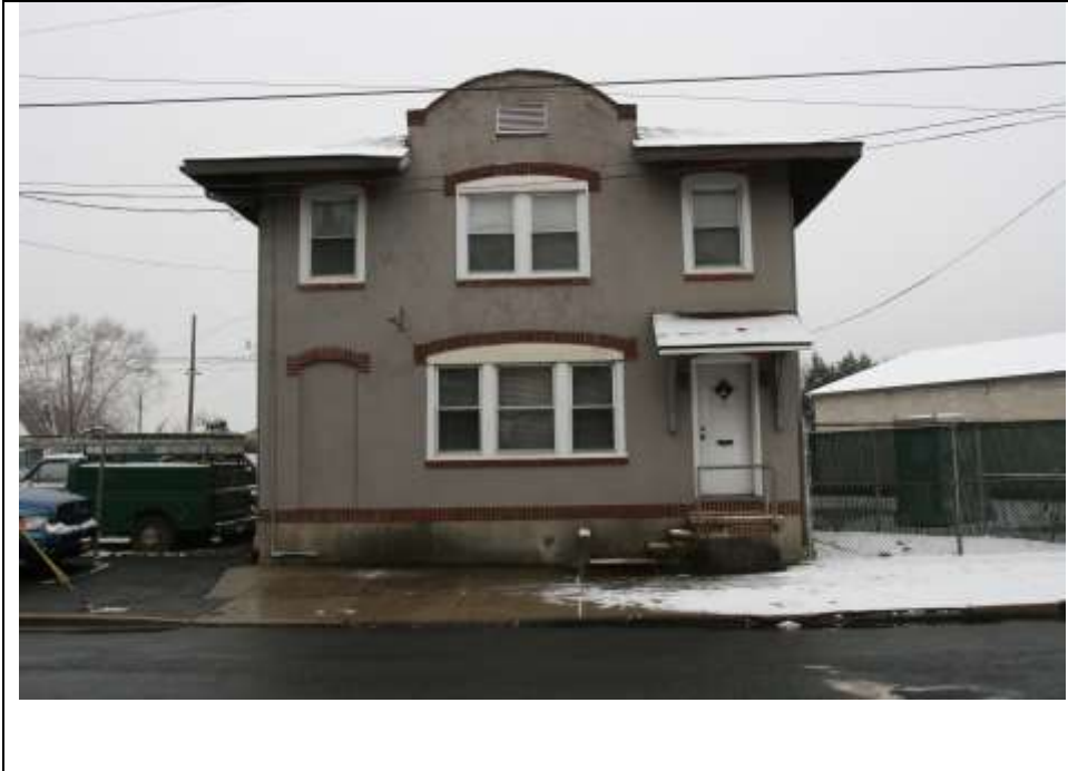
Photograph 2: Northeast elevation (façade) of the former Gallagher Brothers Inc. office at 806 Market Street.. Note the infilled entrance at the left. Looking southwest (January 2019).
