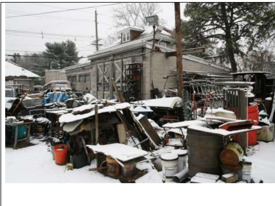
Photograph 10: Northwest (side) and southwest (rear) elevations of the Garage/Workshop. Looking northeast (January 2019).
