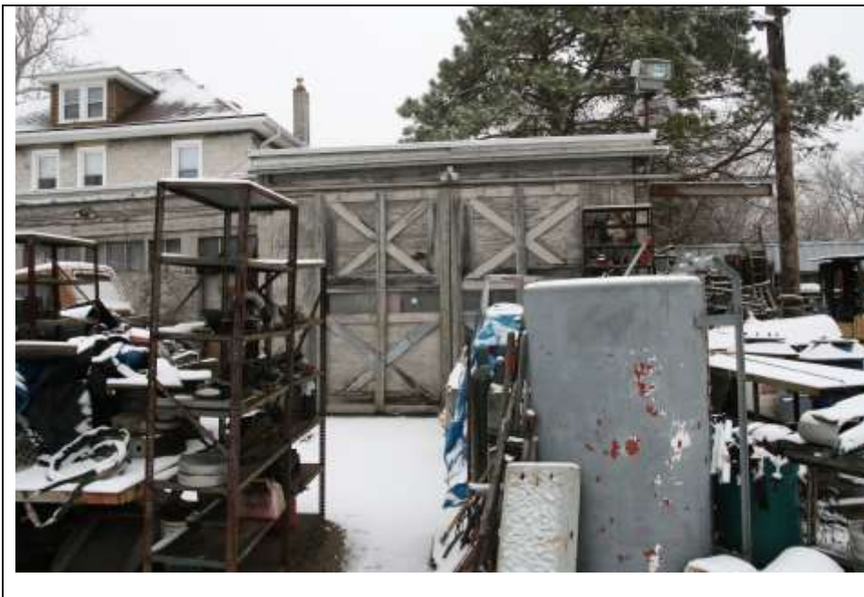
Photograph 13: Southern portion of northwest (side) elevation of the Garage/Workshop. Note the plywood construction. Looking east (January 2019).
