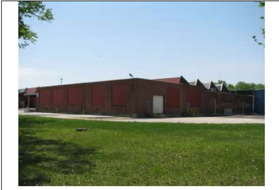
Photograph 14: Northeast and northwest elevations of the 1948 Unit B. The facility with the sawtooth roof (background) is the 1918 machine shop (Unit E). The northwest elevation of Unit E is also visible. Looking south (May 2014).
