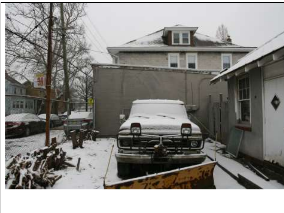
Photograph 11: North portion of northwest (side) elevation of the Garage/Workshop; note the concrete block construction. The façade of the gas station is visible on the right. Looking east (January 2019).
