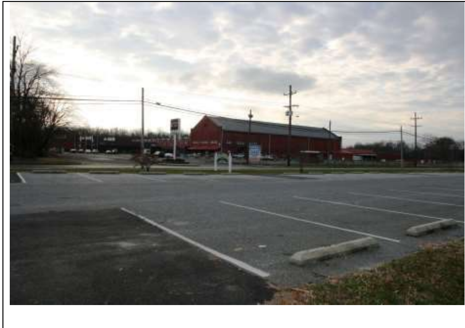
Photograph 1: Overview of the plant from the primary Sewell Street entrance. Looking southwest (December 2018).
