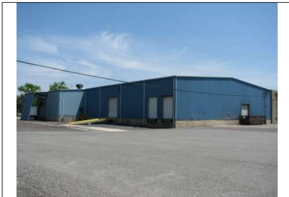
Photograph 26: Northwest and southwest elevations of the circa -1980 Unit J. Looking east (May 2014).
