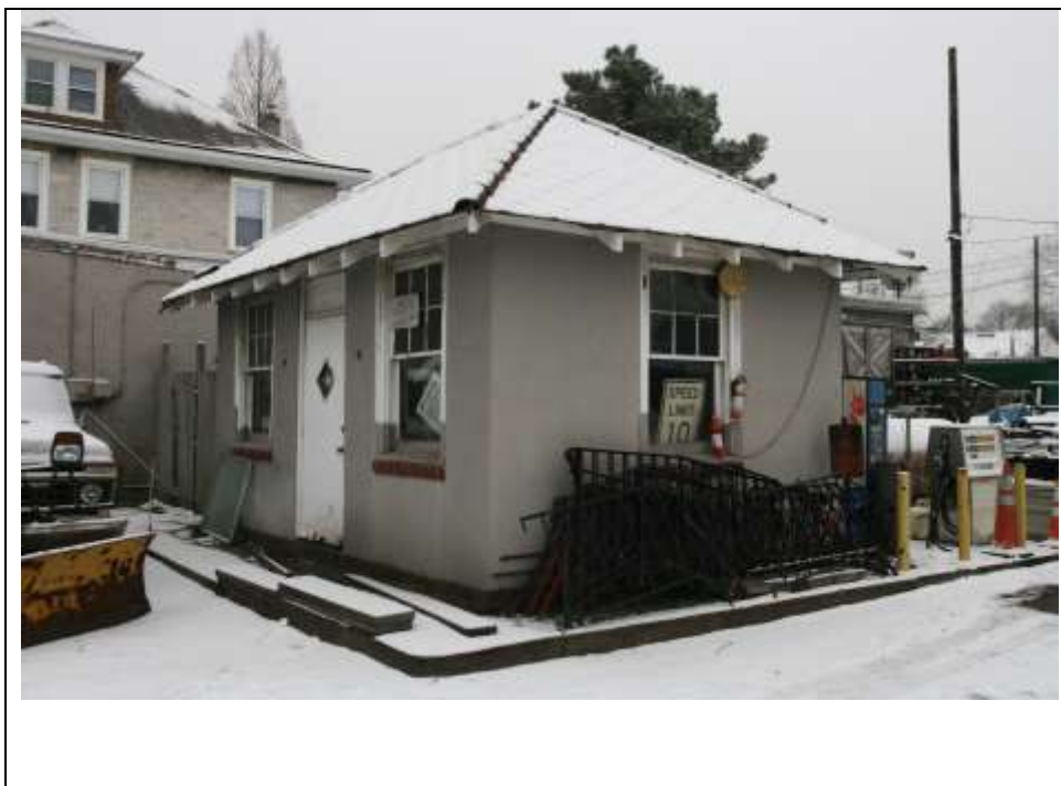
Photograph 6: Northeast (façade) and northwest (side) elevations of the Gas Station. Looking southeast (January 2019).
