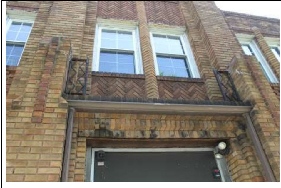
Photograph 4: Detail of brickwork and ironwork in the second story of the façade's central tower. Looking northeast (May 2014).
