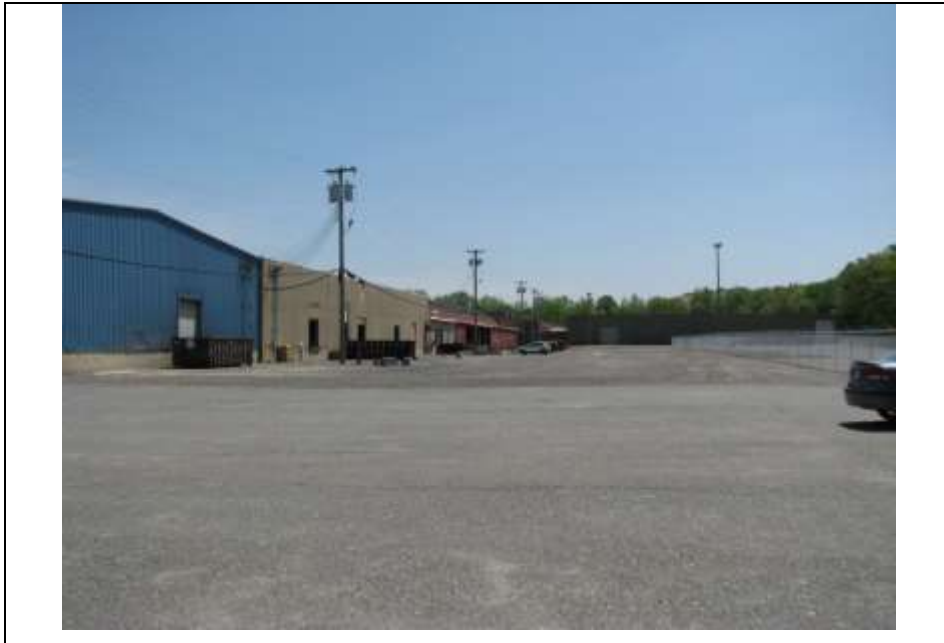
Photograph 10: Overview of the southwest elevation of the plant, showing (at left, from foreground to background) Unit J, Unit I, the wooden box shop (Unit H), and the storehouse (Unit G). Unit K is at right background. Looking southeast (May 2014).
