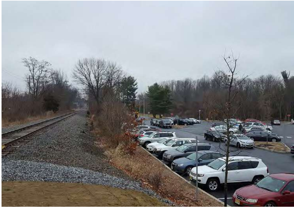
Photograph 43: View of the proposed Rowan University West Station showing the prepared railroad berm and parking lot on the east side, facing north (February 2018).
