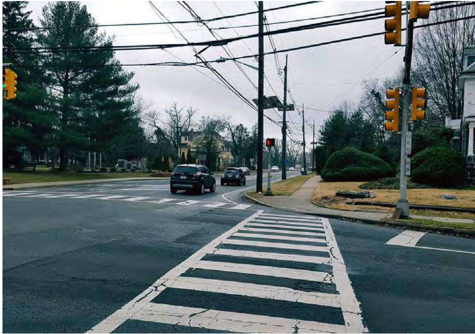
Photograph 54: View of the northwest quadrant of the Cooper Street intersection improvement area showing the road, sidewalk, and landscaped yard, facing northwest (February 2018).
