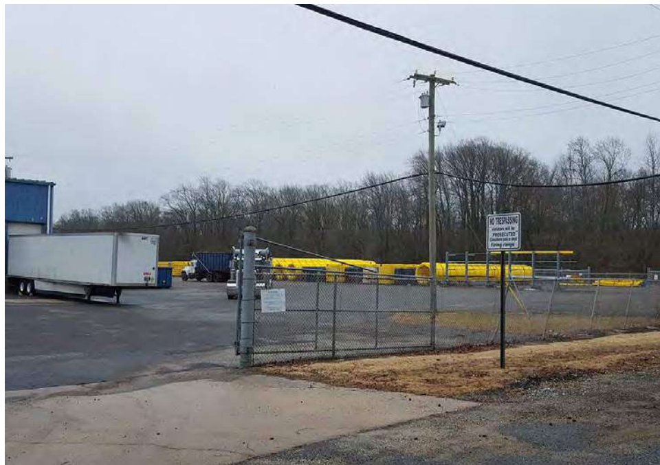
Photograph 48: View of a paved area in the northwest corner of the New Glassboro Yard Site, facing southwest (February 2018).
