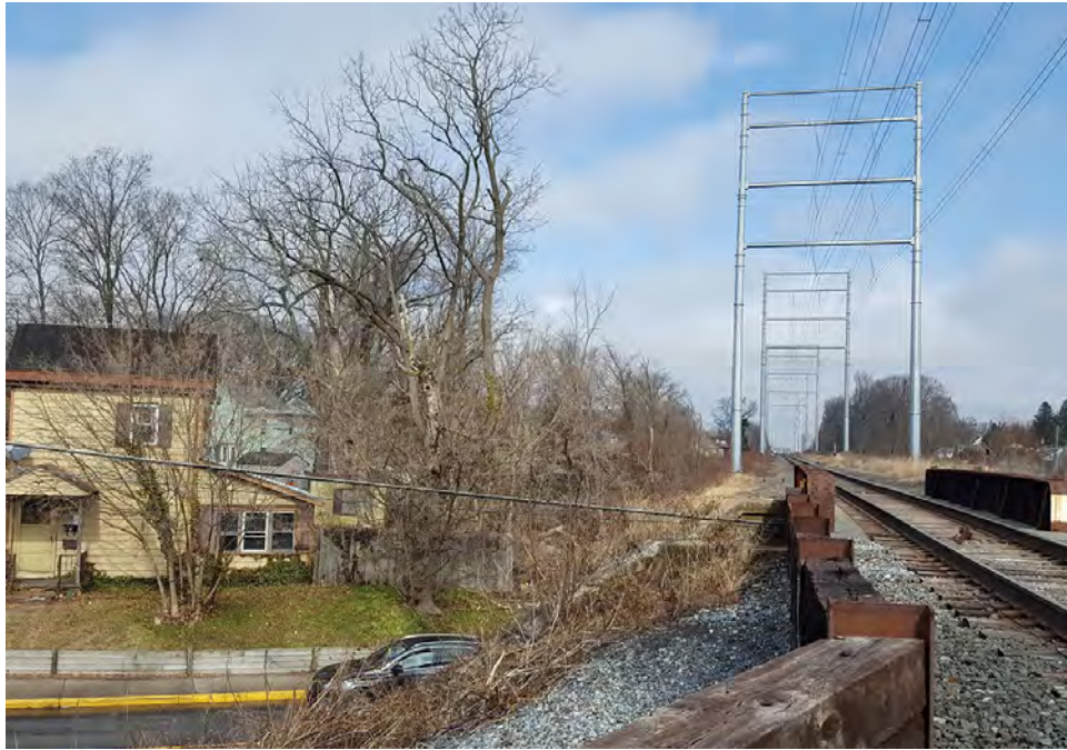
Photograph 39: View of the steep berm on the west side of the Conrail Line at the proposed Red Bank Avenue Station, facing northeast (February 2018).
