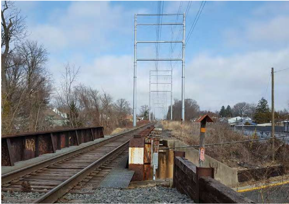
Photograph 37: View of the proposed Red Bank Avenue Station on the raised Conrail Line, facing northeast (February 2018).
