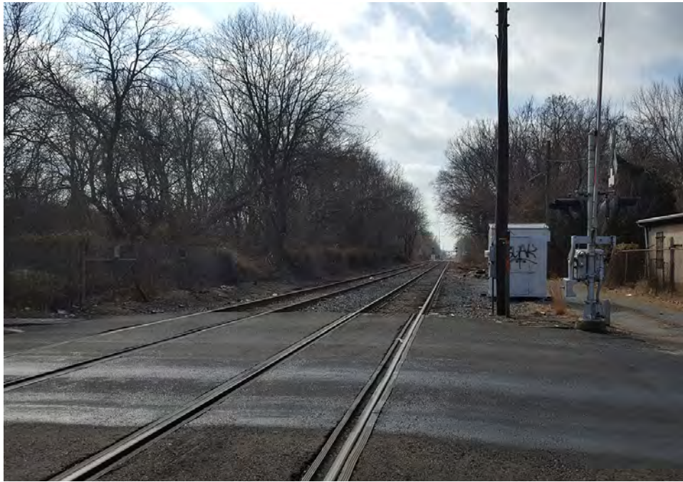
Photograph 61: View of the proposed GCL corridor along Railroad Avenue in Camden, facing south (February 2018).
