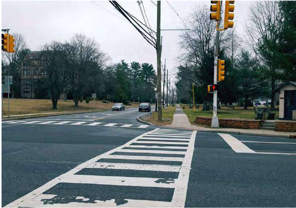
Photograph 52: View of the southwest quadrant of the Cooper Street intersection improvement area showing the road and sidewalk within the APE, facing southwest (February 2018).
