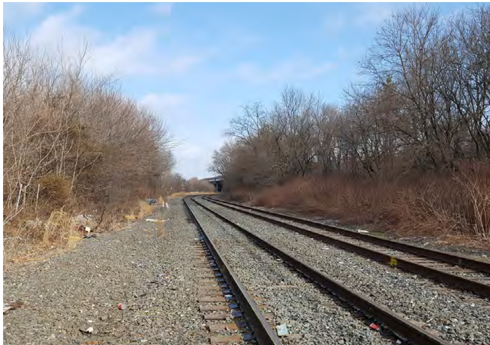
Photograph 62: View of the proposed GCL corridor along Railroad Avenue in Camden, facing north (February 2018).
