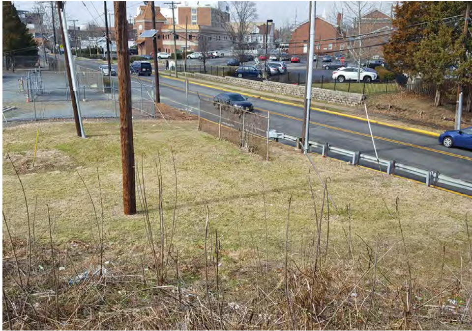
Photograph 41: View of the grassy lawn at the intersection of East Red Bank Avenue and the bridge that carries the Conrail Line, showing the location of underground utility lines (water main), facing northwest (February 2018).
