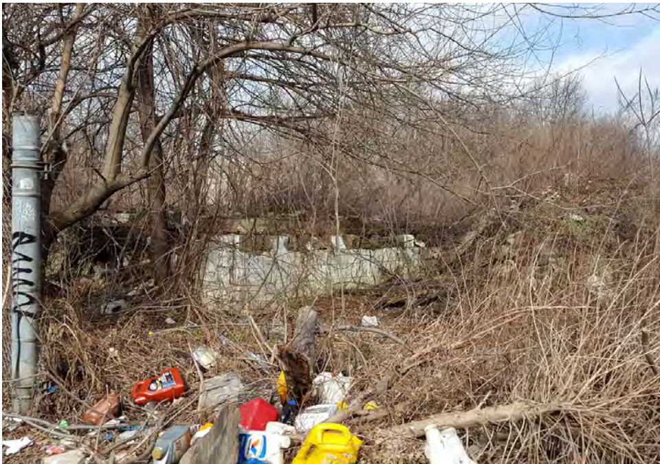
Photograph 11: View of the southern edge of Test Area 3 showing partially demolished buildings, spoil piles, and recent garbage piles, facing north (February 2018).
