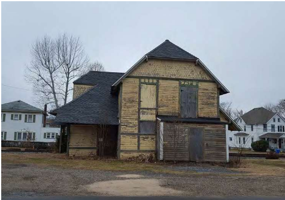
Photograph 18: View of the abandoned Sewell Station south of Test Area 9, facing southwest (February 2018).
