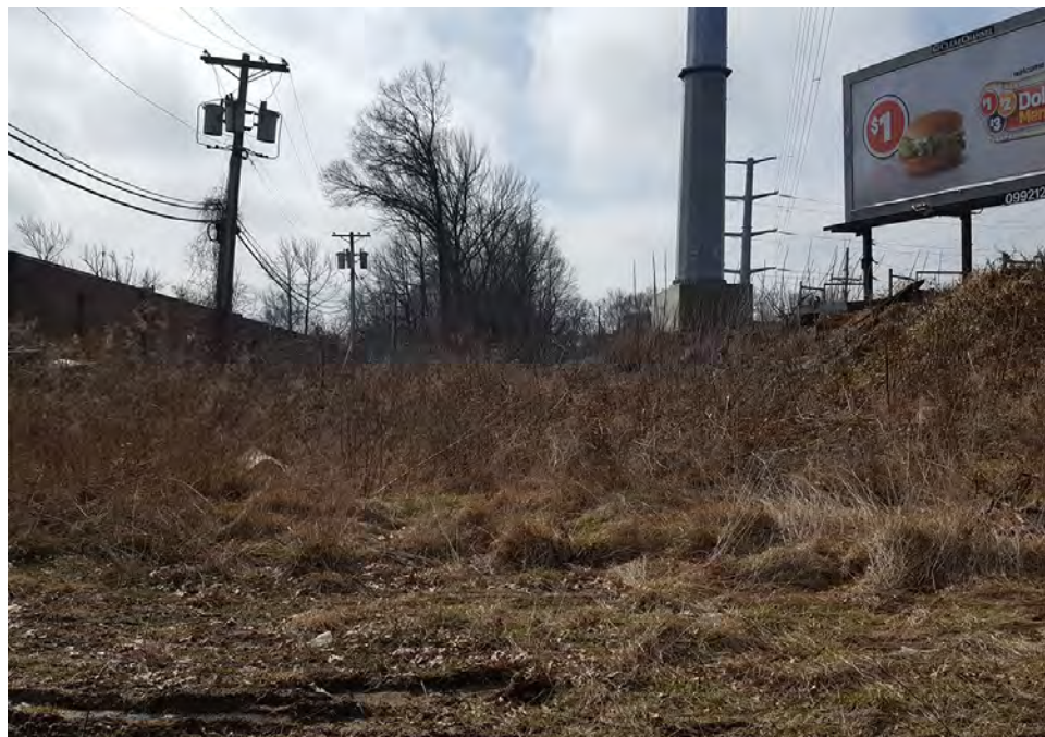
Photograph 40: View of the steep berm on the east side of the Conrail Line at the proposed Red Bank Avenue Station, facing southwest (February 2018).
