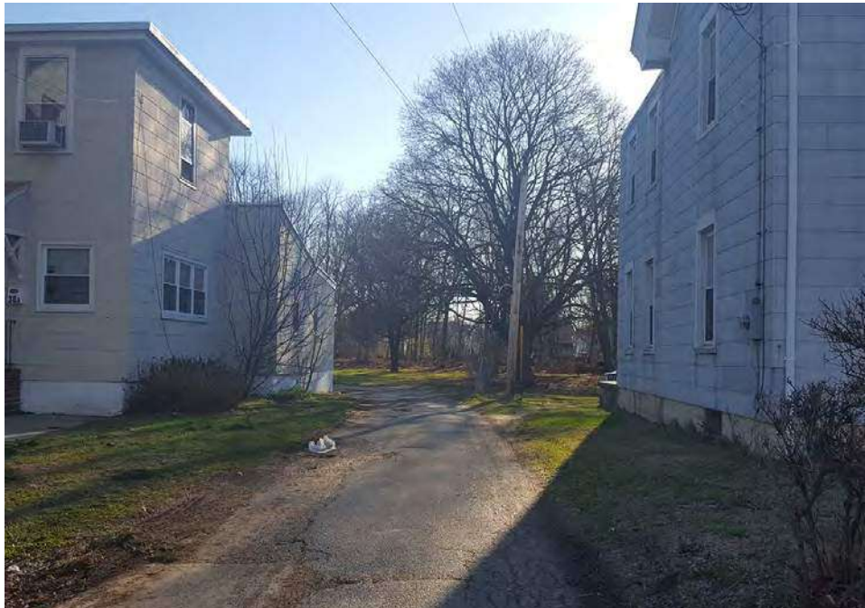
Photograph 28: View of the western end of Test Area 13 showing some of the nineteenth-century buildings at this location, facing east (February 2018).
