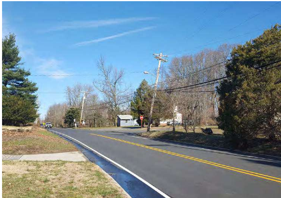
Photograph 55: View of the intersection at Tylers Mill Road and Main Street in Mantua Township showing the road, road berms, and underground utility corridors, facing northwest (February 2018).
