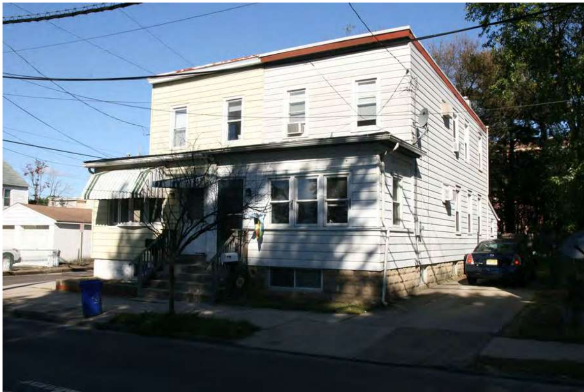
Photograph 25: 13-15 Koehler Street, Gloucester City (October 2018).
