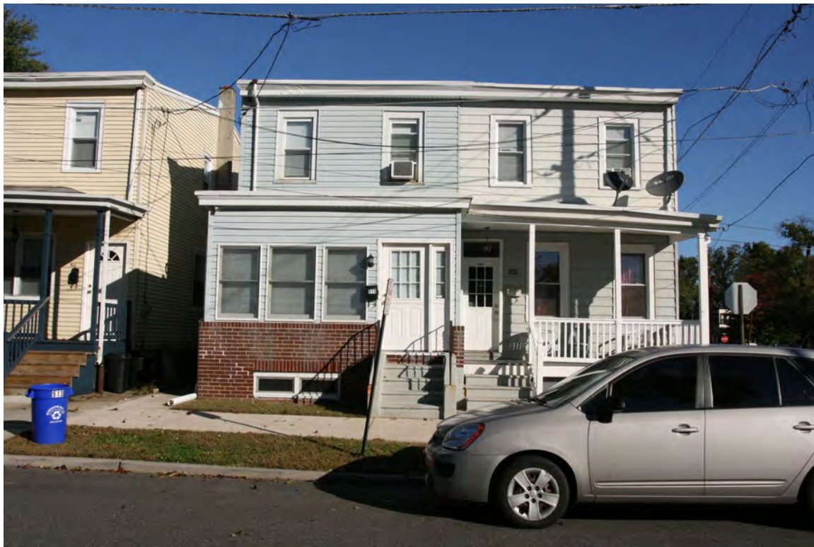
Photograph 7: 513-515 Mercer Street, Gloucester City (October 2018).
