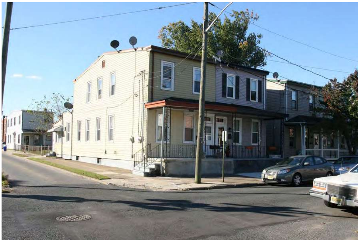
Photograph 12: 512-514 Middlesex Street, Gloucester City (October 2018).
