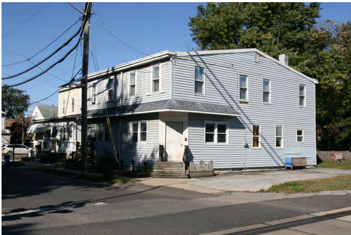
Photograph 26: 17-19 Koehler Street, Gloucester City (October 2018).
