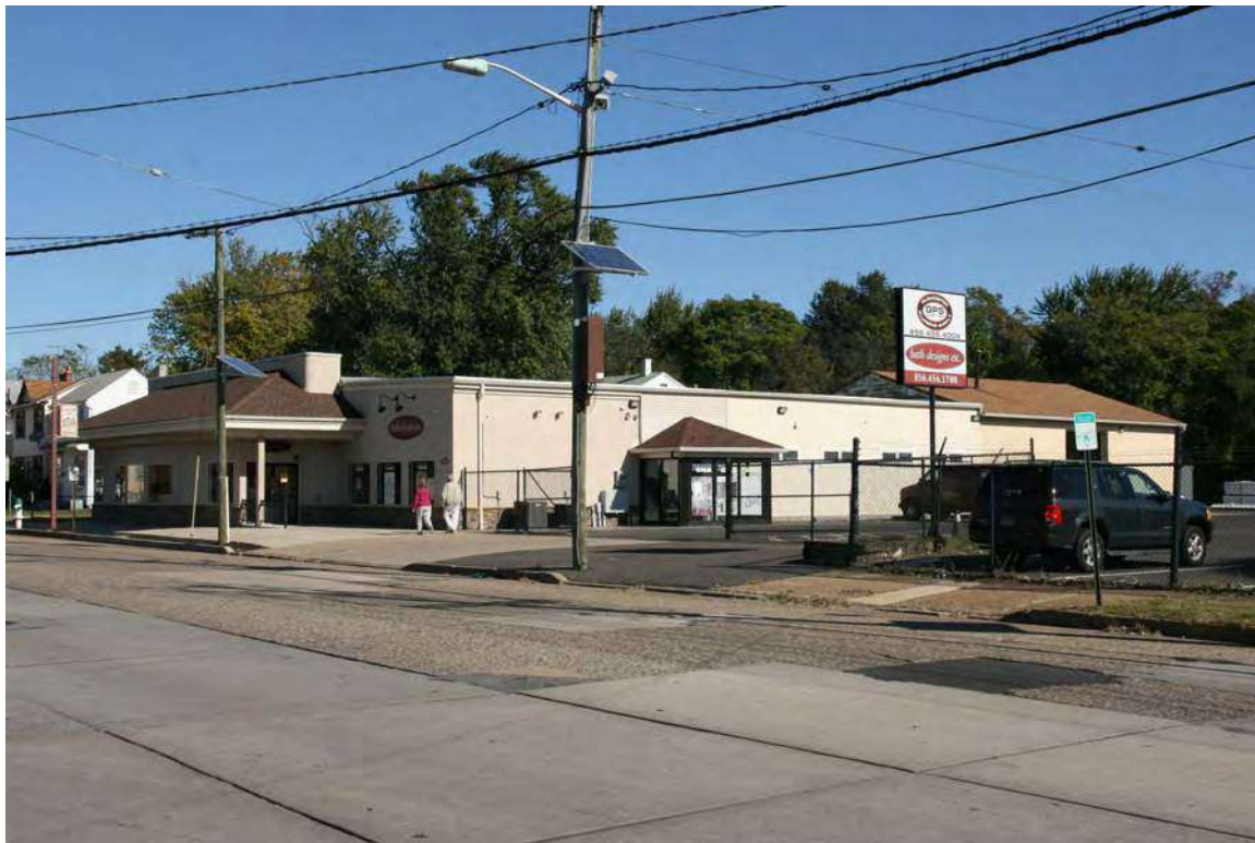
Photograph 31: 520 South Broadway, Gloucester City (October 2018).
