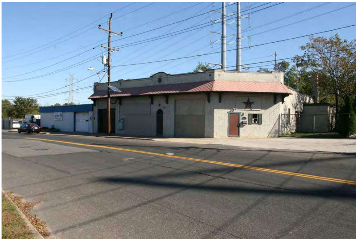
Photograph 32: 500-510 New Broadway, Brooklawn Borough (October 2018).
