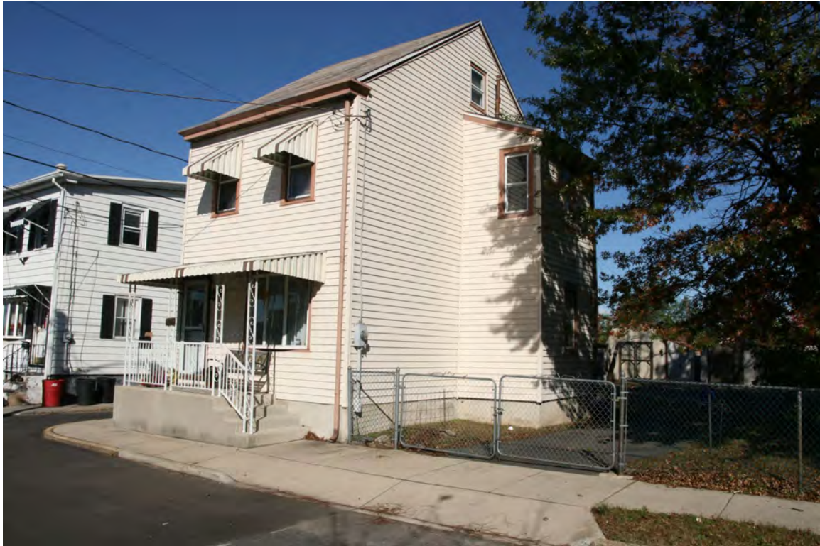
Photograph 19: 921 George Street, Gloucester City (October 2018).
