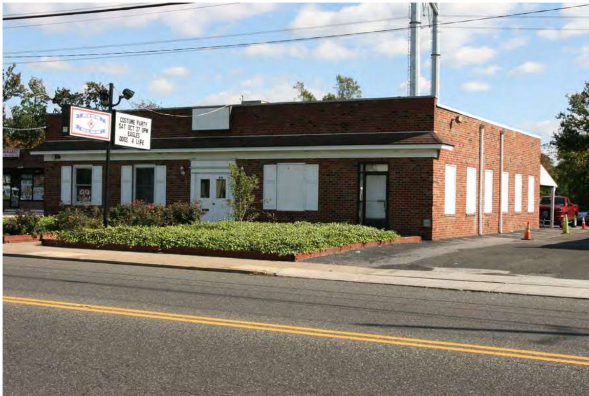
Photograph 35: 818 N. Broad Street, Woodbury City (October 2018).
