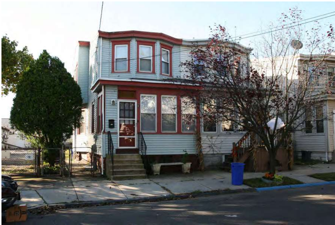
Photograph 9: 508-510 Mercer Street, Gloucester City (October 2018).
