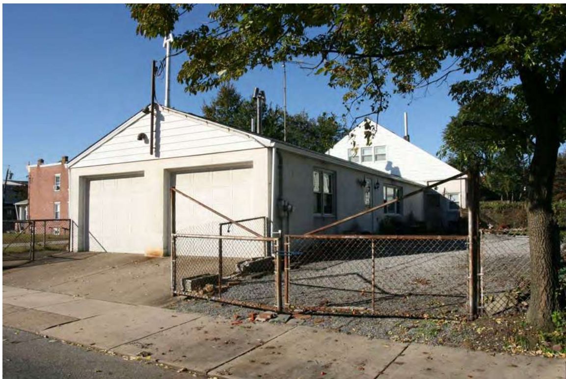
Photograph 10: 512 Mercer Street, Gloucester City (October 2018).
