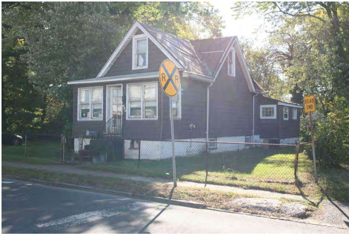
Photograph 27: 128 Koehler Street, Gloucester City (October 2018).
