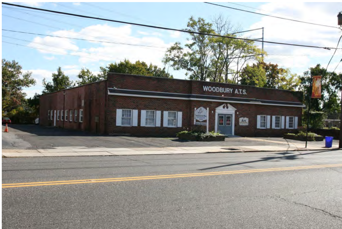
Photograph 36: 814 N. Broad Street, Woodbury City (October 2018).
