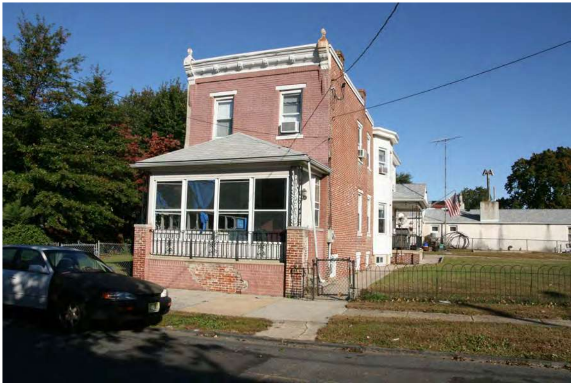
Photograph 11: 509 Middlesex Street, Gloucester City (October 2018).
