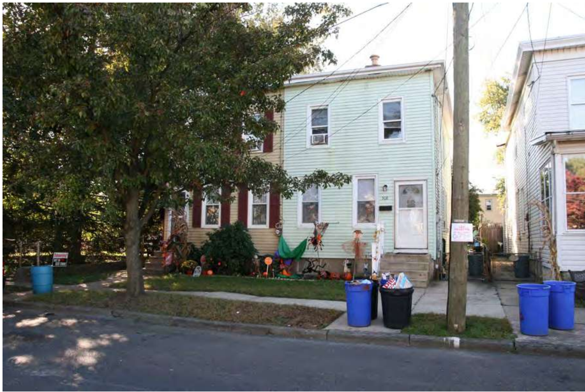
Photograph 5: 508-510 Morris Street, Gloucester City (October 2018).
