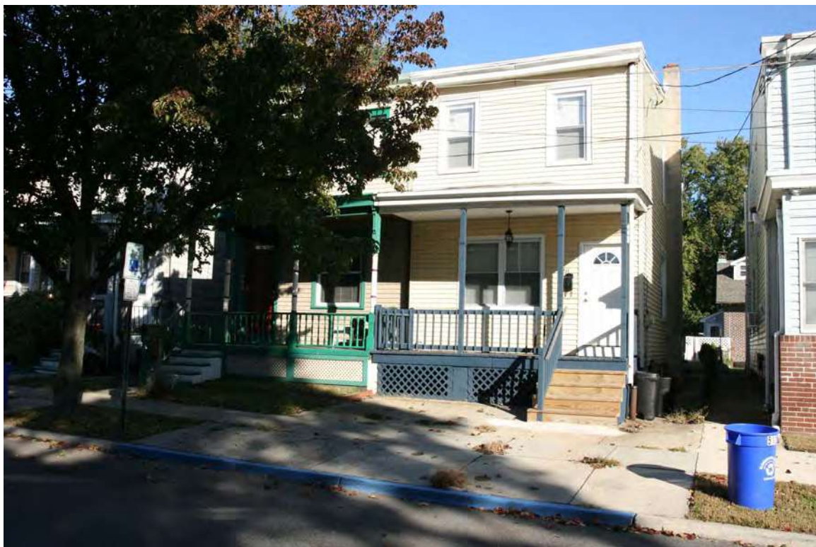
Photograph 8: 509-511 Mercer Street, Gloucester City (October 2018).
