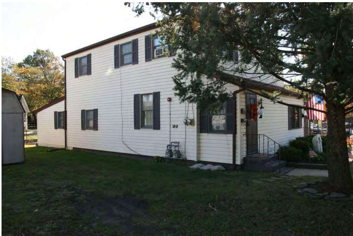
Photograph 24: 420-422 South Broadway, Gloucester City (October 2018).
