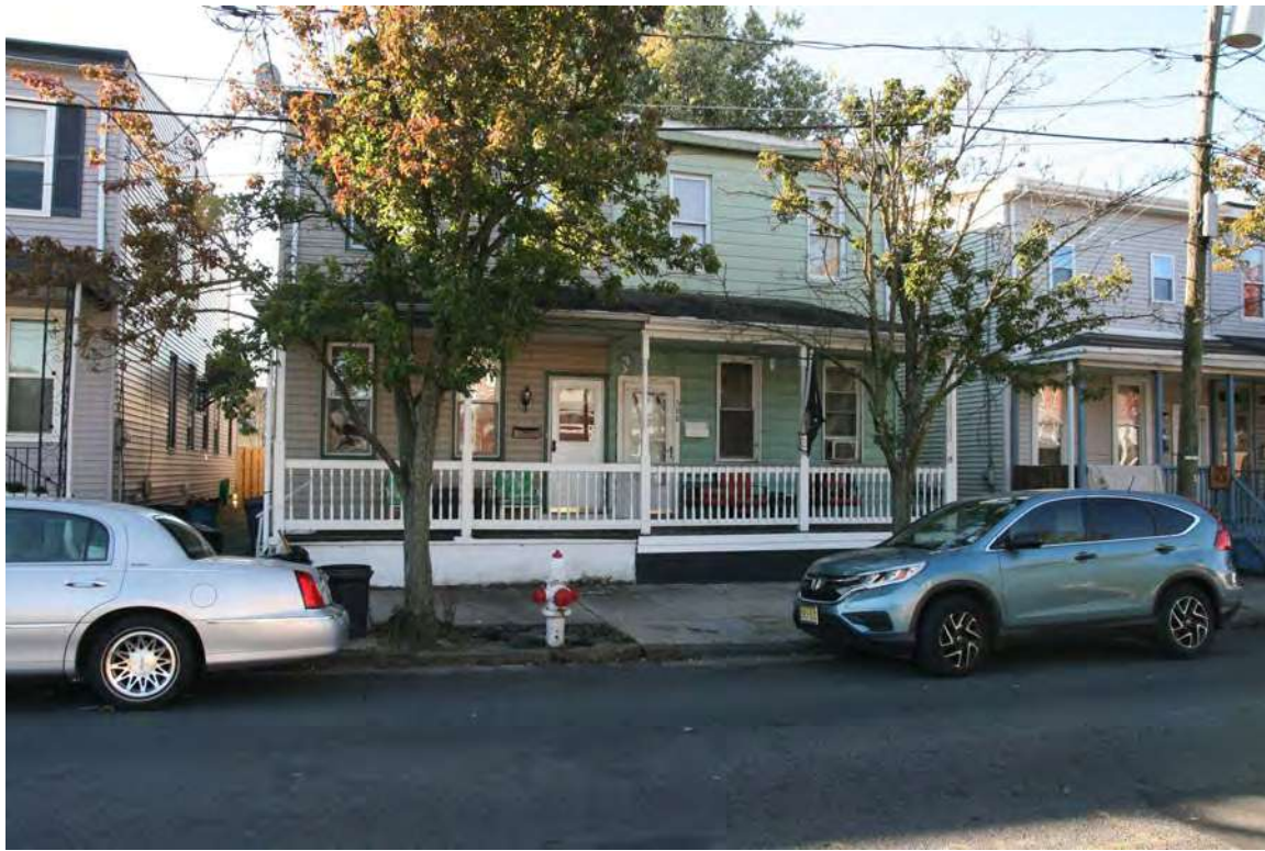
Photograph 13: 508-510 Middlesex Street, Gloucester City (October 2018).
