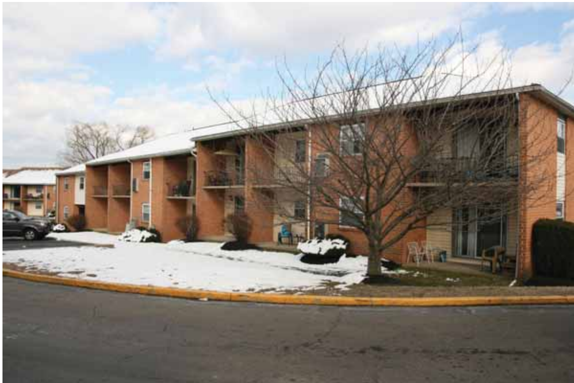
Photograph 26: Crossing at Glassboro, 515 Mullica Hill Road, Glassboro Borough (March 2018).
