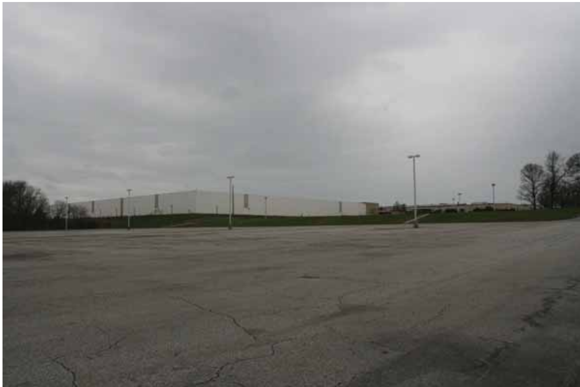
Photograph 22: Sony CD Plant, 400 N. Woodbury Road, Mantua Township (Pitman; April 2018).
