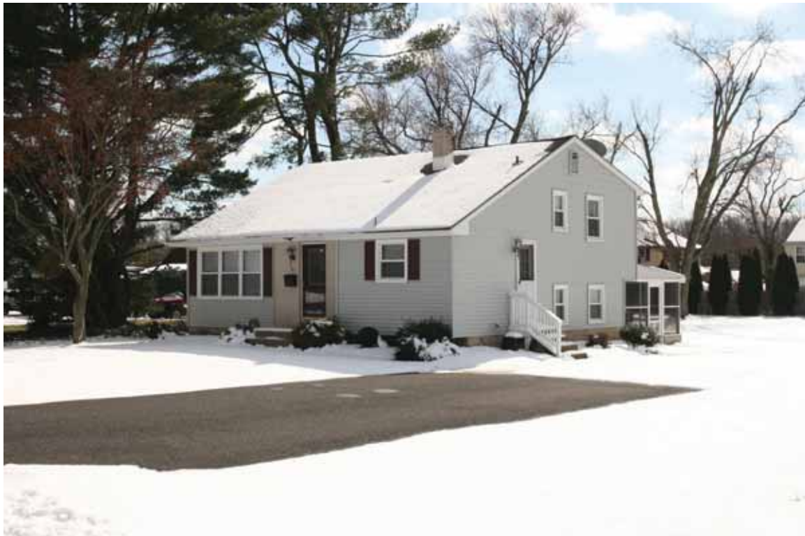
Photograph 20: 765 W. Atlantic Avenue, Mantua Township (Sewell; March 2018).
