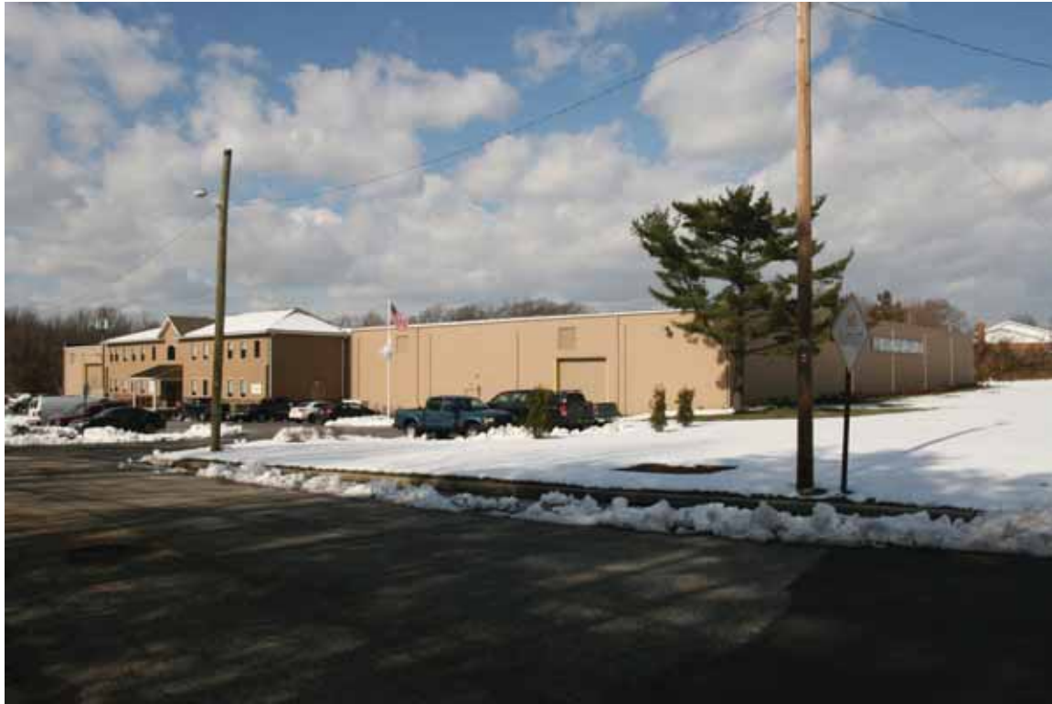
Photograph 21: 360 Columbia Drive, Mantua Township (Pitman; March 2018).
