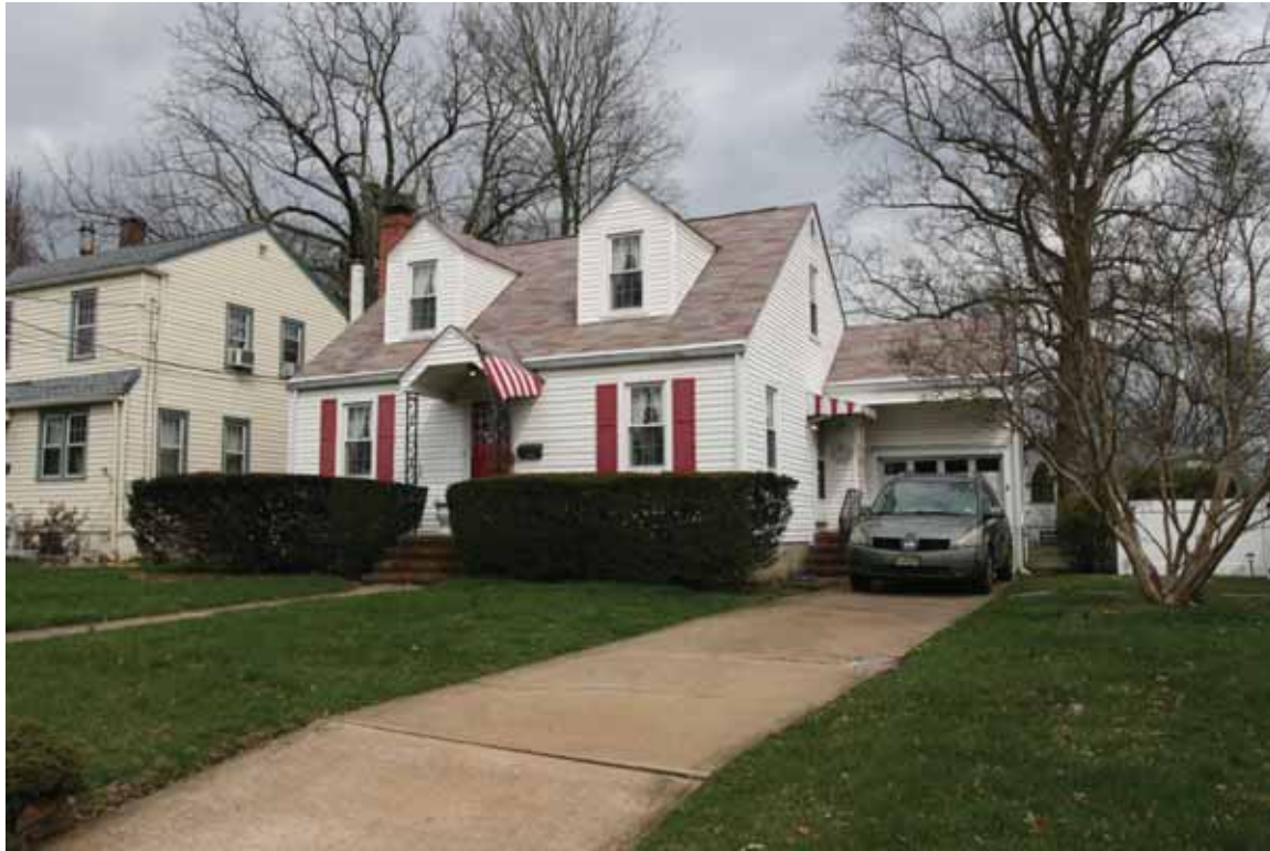
Photograph 17: 459 Oak Avenue, Woodbury Heights Borough (April 2018).
