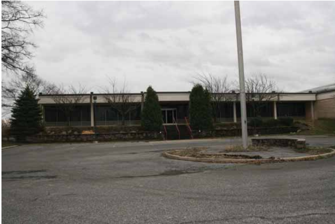
Photograph 23: Sony CD Plant, 400 N. Woodbury Road, Mantua Township (Pitman; April 2018).
