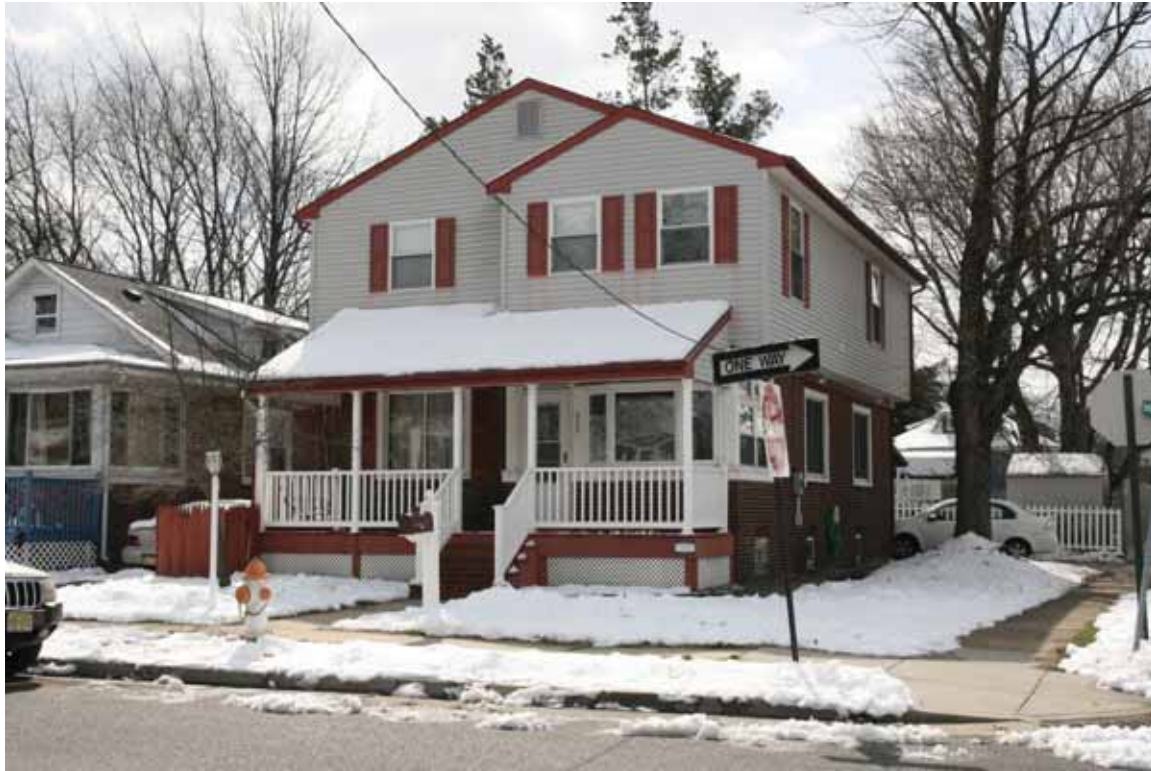
Photograph 3: 800 Mercer Street, Gloucester City (March 2018).
