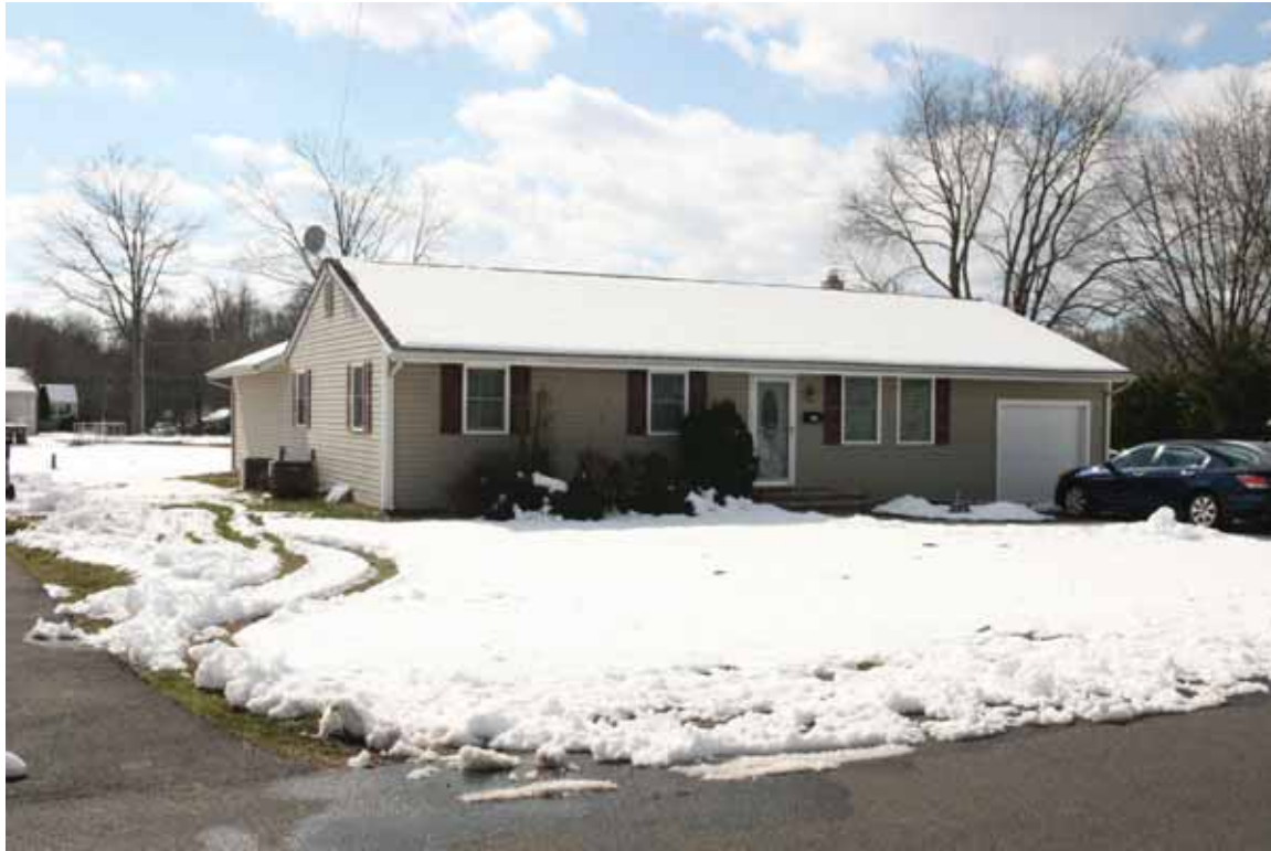
Photograph 19: 761 W. Atlantic Avenue, Mantua Township (Sewell; March 2018).
