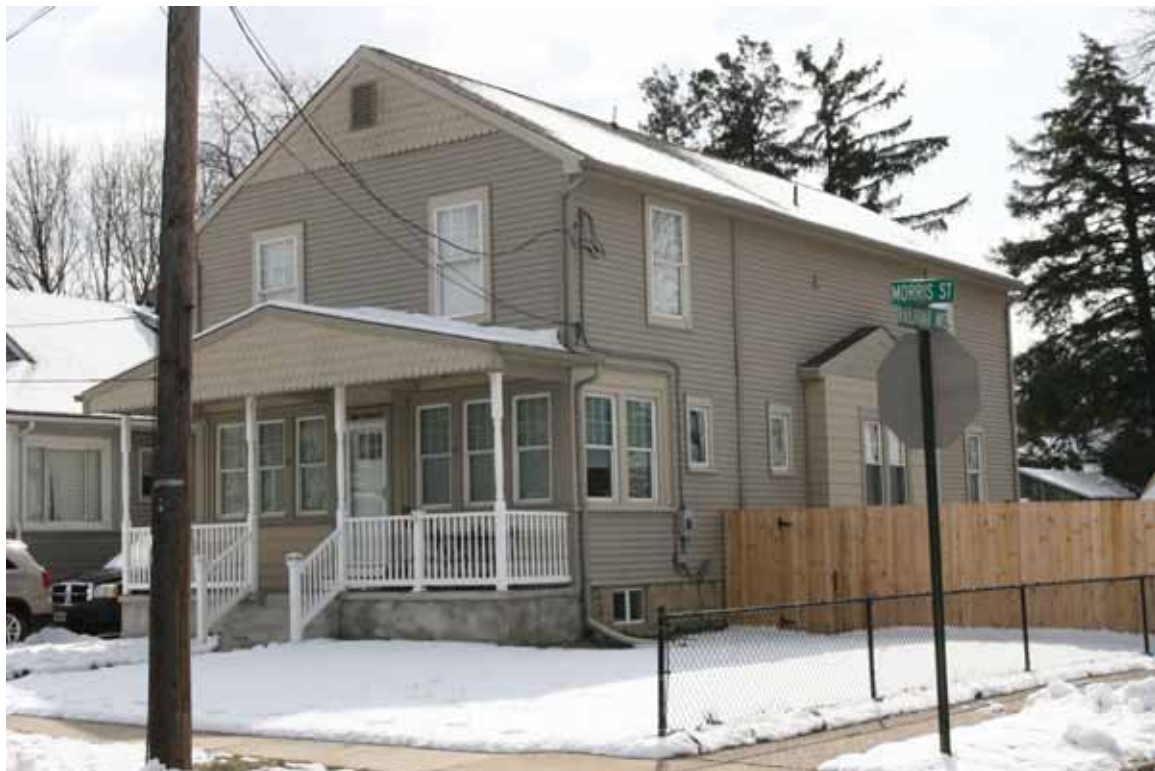
Photograph 2: 800 Morris Street, Gloucester City (March 2018).
