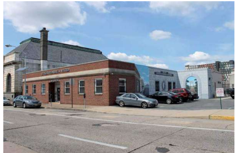
Photograph 4: 415 Federal Street, Camden City.
