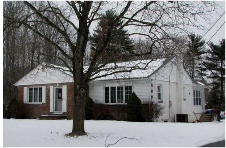
Photograph 50: 825 Main Street, Mantua Township.
