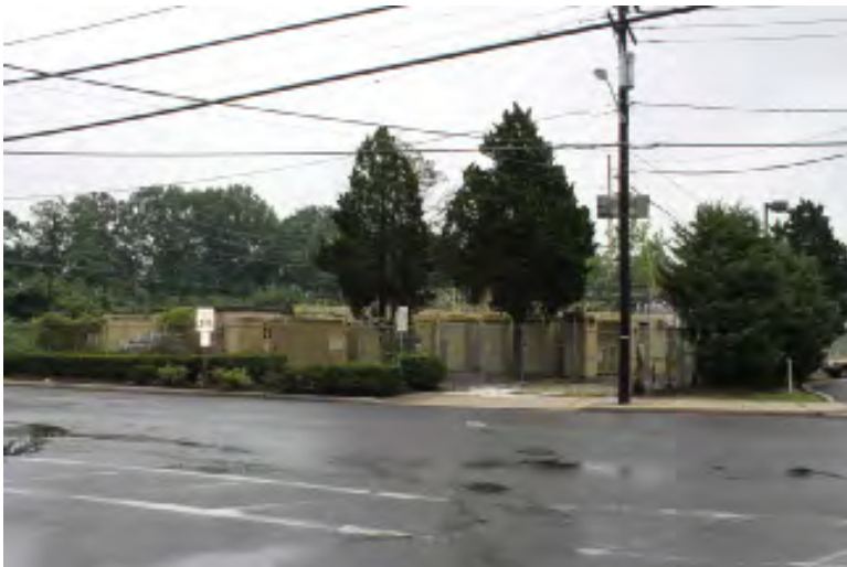
Photograph 263: E. Red Bank Avenue Electrical Substation, Woodbury City.
