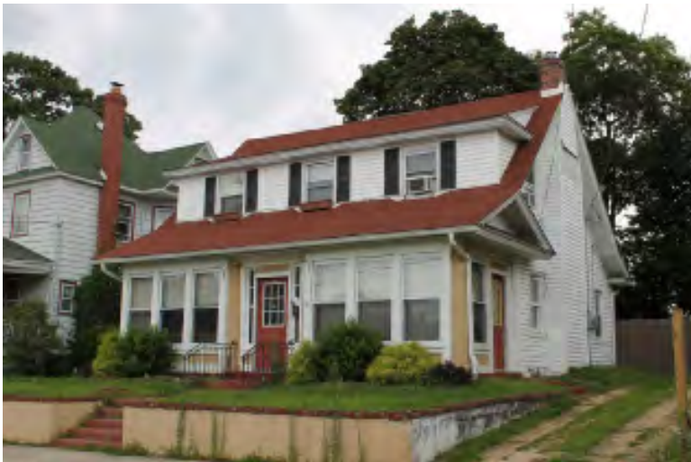
Photograph 199: Simpson Avenue Residential Streetscape, Pitman Borough. View looking northeast to 51 Simpson Avenue.
