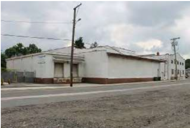
Photograph 179: 55 Commerce Avenue (Riley/Fay Sales Company Milk, Ice, and Cold Storage), Pitman Borough. View of west (front) and north (side) elevations.
