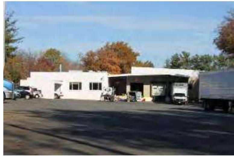
Photograph 254: 535 Glassboro Road, Woodbury City.
