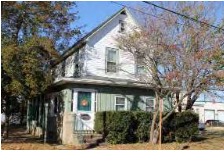
Photograph 243: 136 Crown Point Road, Westville Borough.
