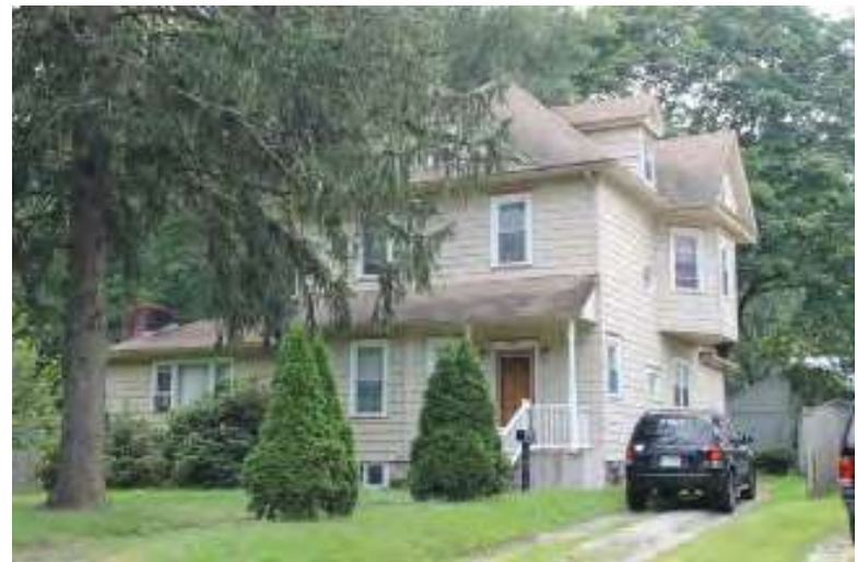
Photograph 280: 883 W. Jersey Avenue, Woodbury Heights Borough.
