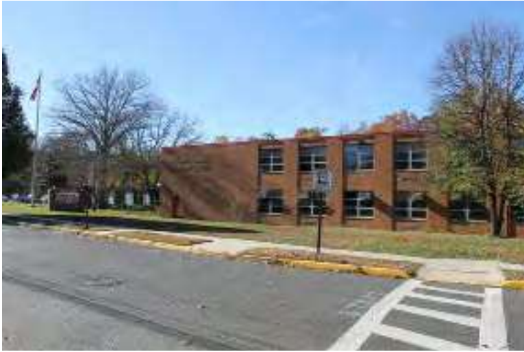
Photograph 269: 100 Academy Avenue (Woodbury Heights Elementary School), Woodbury Heights Borough.
