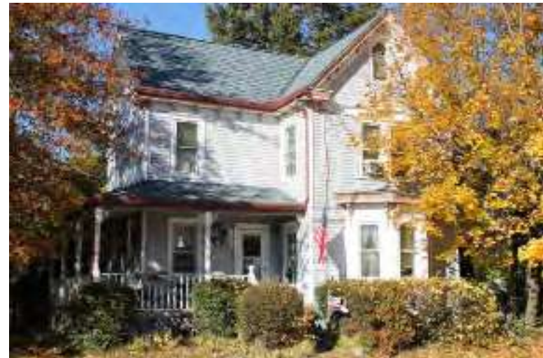
Photograph 244: 148 Crown Point Road, Westville Borough.
