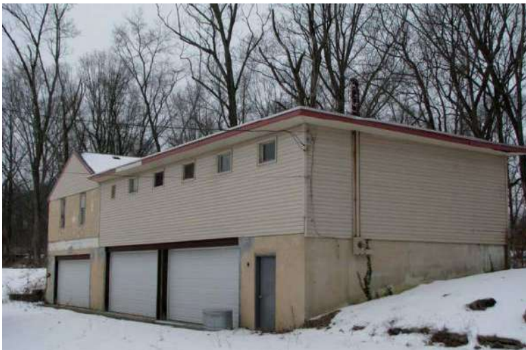
Photograph 7: 204 Bark Bridge Road, Deptford Township. View showing a garage/workshop.
