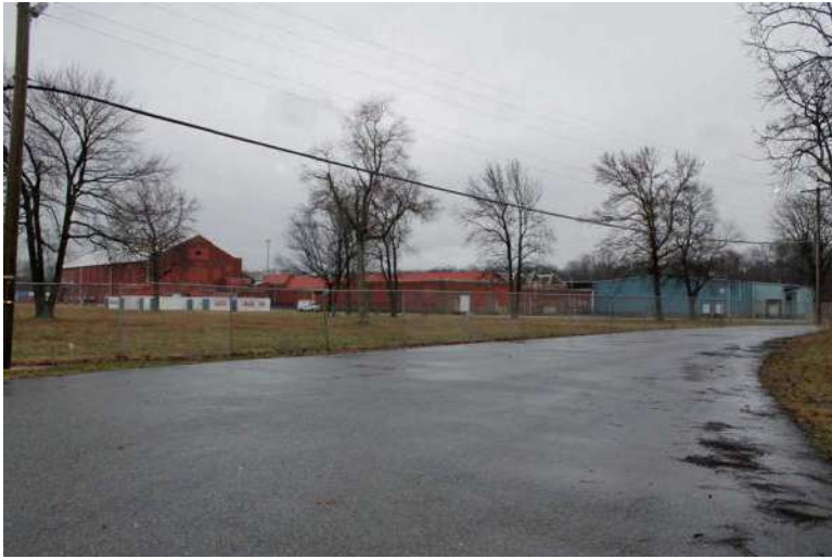
Photograph 33: 70 Sewell Street (Owens Illinois Glass Company/ former Owens Bottle Company) Plant No. 8, Glassboro Borough. View looking southeast from Sewell Street.
