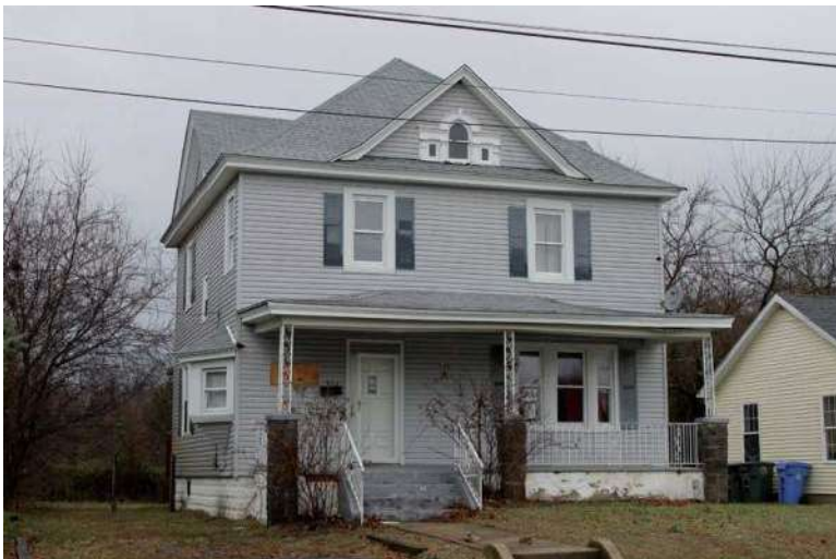
Photograph 35: 213 Wilmer Street, Glassboro Borough.
