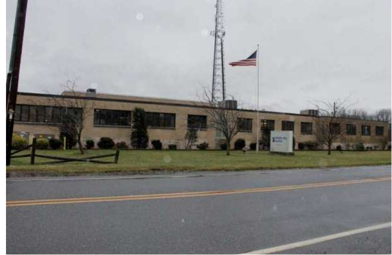
Photograph 18: 428 Ellis Street (Atlantic City Electric), Glassboro Borough.
