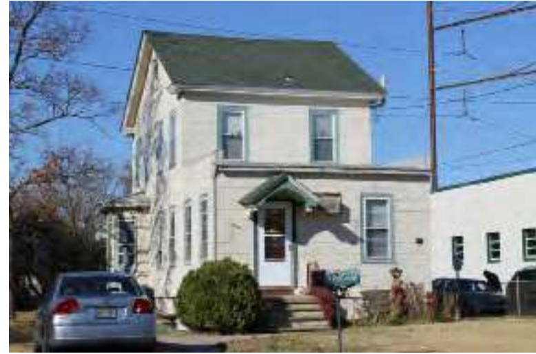
Photograph 242: 128 Crown Point Road, Westville Borough.
