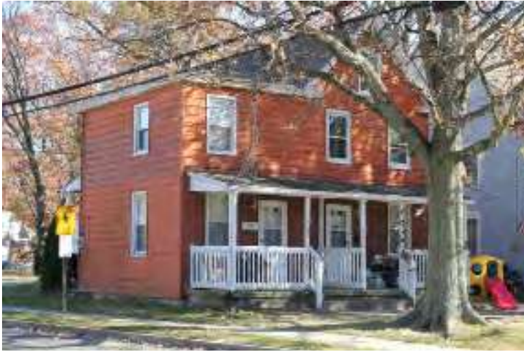
Photograph 189: 201-203 W. Jersey Avenue, Pitman Borough.
