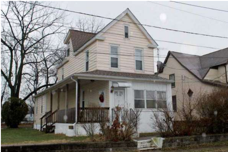
Photograph 83: 1036 Washington Avenue, Woodbury City.
