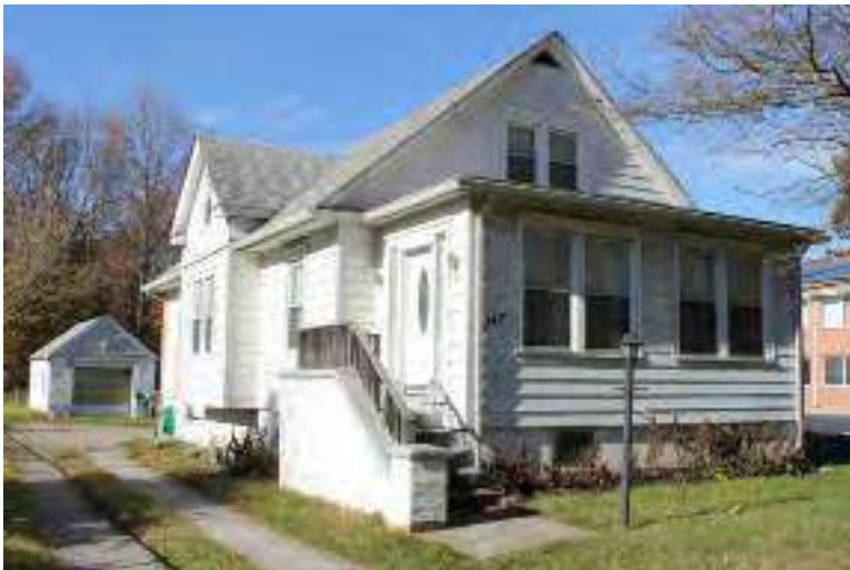
Photograph 275: 347 Glassboro Road, Woodbury Heights Borough.
