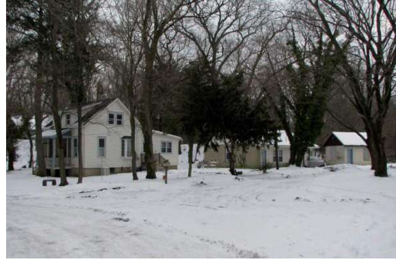
Photograph 10: 205 Bark Bridge Road, Deptford Township. Overview showing the primary dwelling (at left), secondary dwelling (center), and shed (at right).
