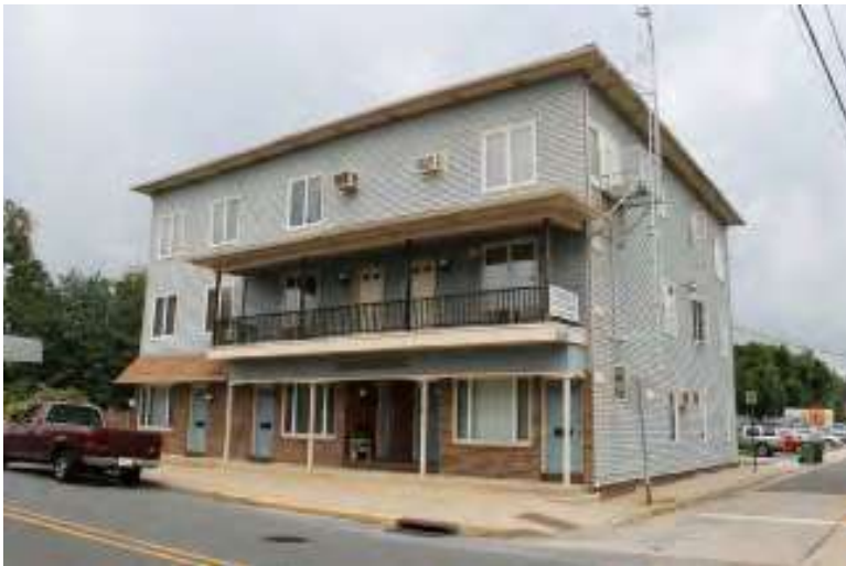
Photograph 195: 42-46 Pitman Avenue, Pitman Borough.
