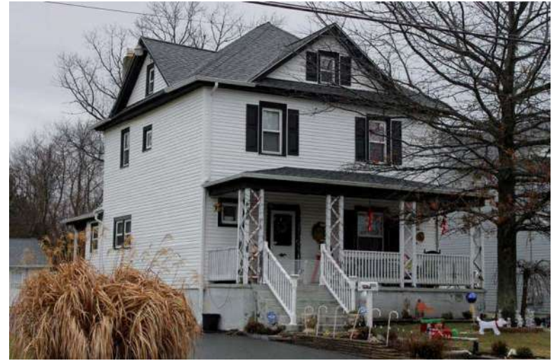
Photograph 38: 221 Wilmer Street, Glassboro Borough.
