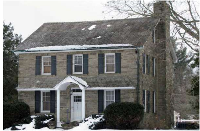
Photograph 54: 856 Main Street, Mantua Township.
