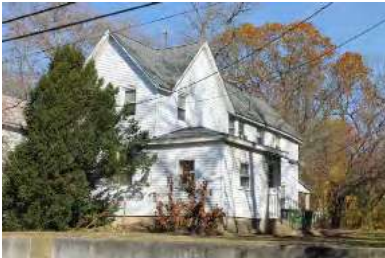
Photograph 183: 135 W. Jersey Avenue, Pitman Borough.
