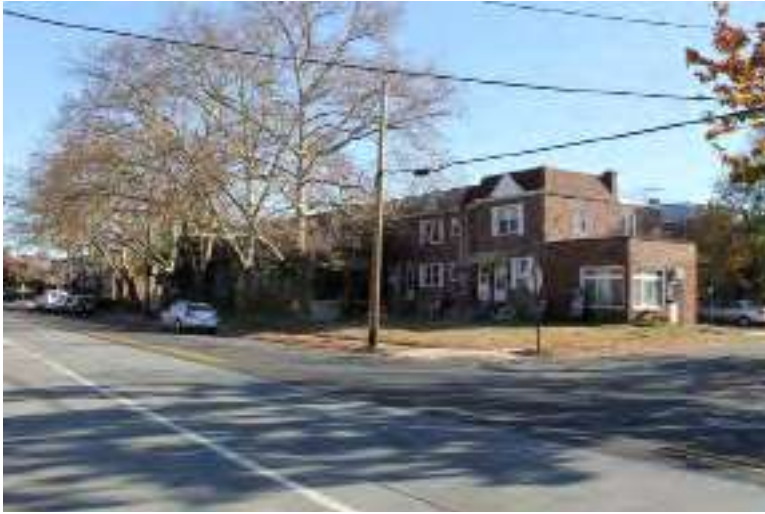
Photograph 241: Broadway Rowhouses (Oak Avenue to Cedar Avenue), Westville Borough.
