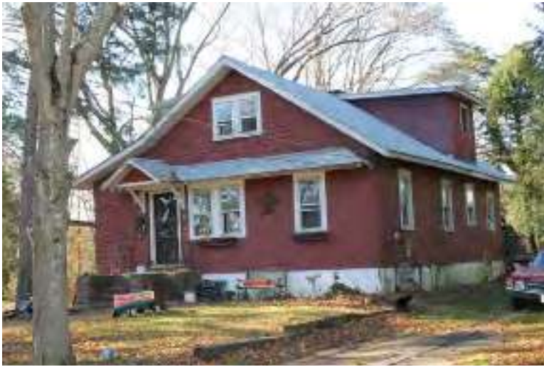
Photograph 165: Hunterdon Avenue (southwest end), Sewell, Mantua Township.
