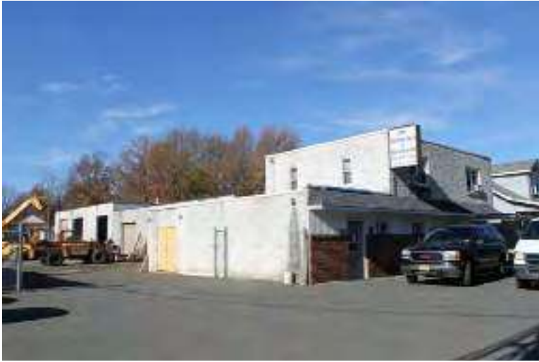
Photograph 277: 363 Glassboro Road, Woodbury Heights Borough.
