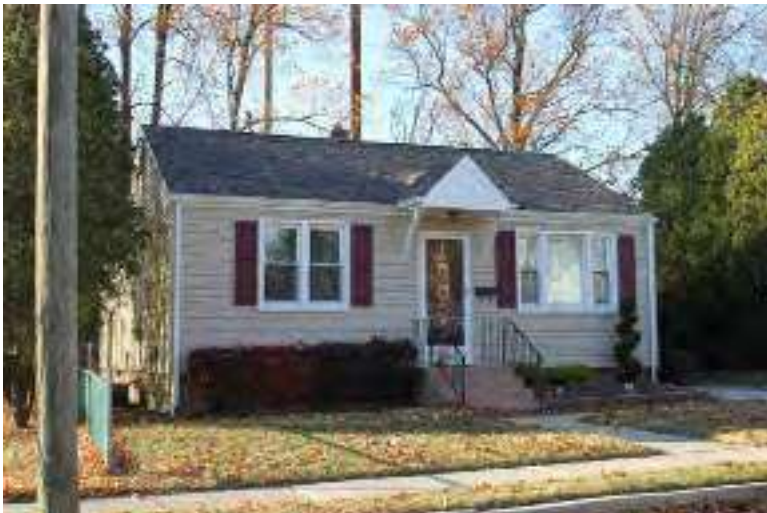
Photograph 267: Washington and Evergreen Avenues Grouping, Woodbury City. View looking northwest toward a representative dwelling at the south end of Washington Avenue within the grouping.
