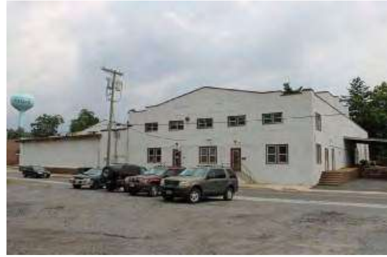
Photograph 178: 55 Commerce Avenue (Riley/Fay Sales Company Milk, Ice, and Cold Storage), Pitman Borough. View of west (front) and south (side) elevations.
