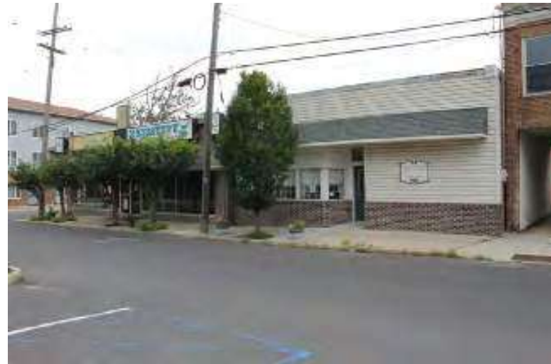
Photograph 192: W. Jersey Avenue Commercial Streetscape, Pitman Borough. View looking northeast toward 107 W. Jersey Avenue.
