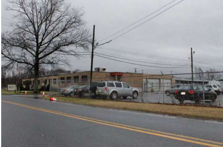
Photograph 19: 428 Ellis Street (Atlantic City Electric), Glassboro Borough.
