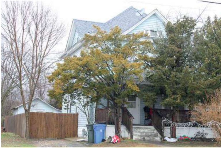
Photograph 37: 217 Wilmer Street, Glassboro Borough.
