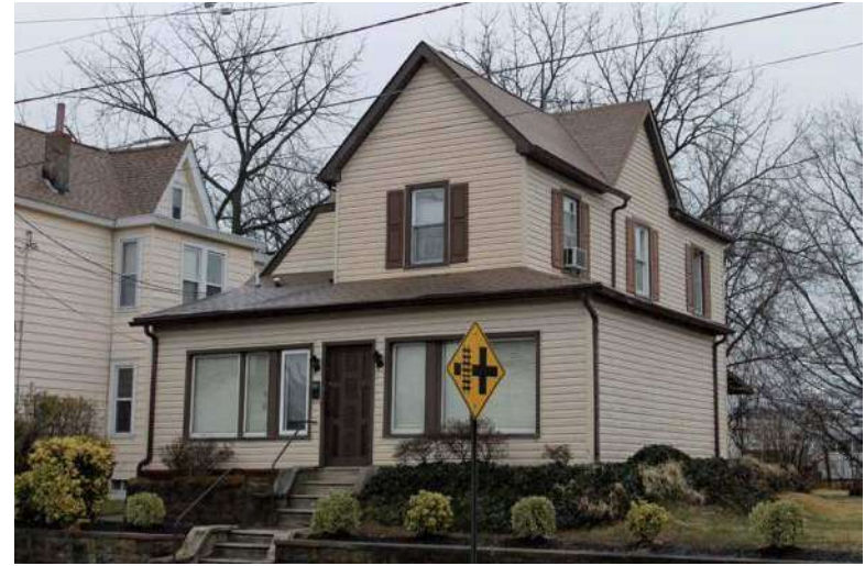
Photograph 82: 1032 Washington Avenue, Woodbury City.
