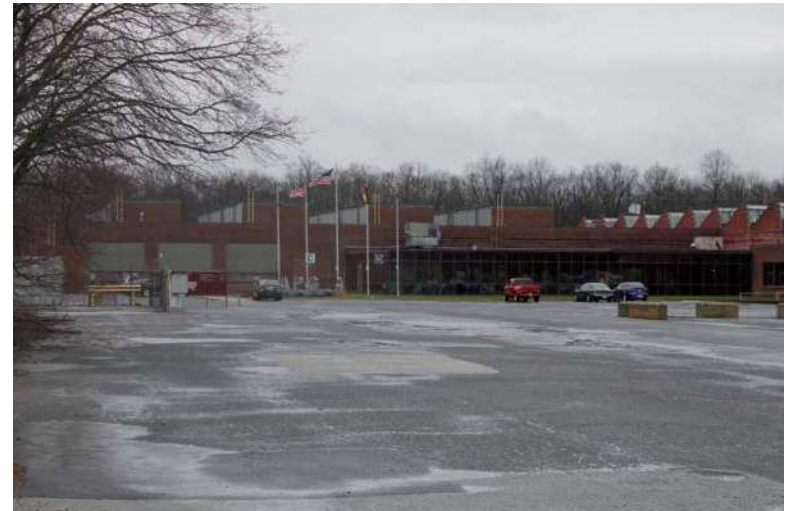
Photograph 32: 70 Sewell Street (Owens Illinois Glass Company/ former Owens Bottle Company) Plant No. 8, Glassboro Borough. View looking south from Sewell Street.
