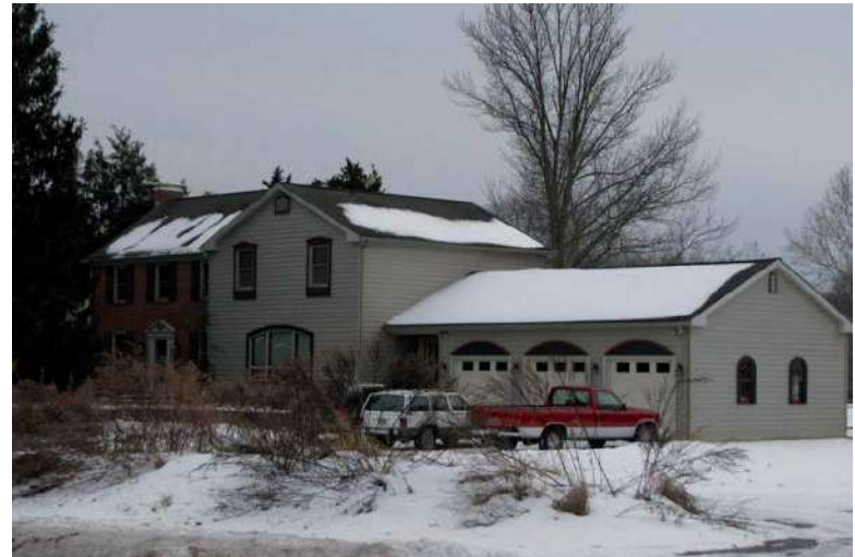
Photograph 52: 844 Main Street, Mantua Township. Overview showing extensive circa -2000 additions.
