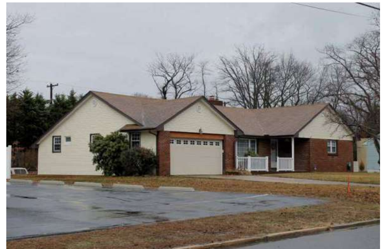
Photograph 40: 305 Wilmer Street, Glassboro Borough.
