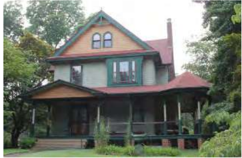
Photograph 278: 791 W. Jersey Avenue, Woodbury Heights Borough.
