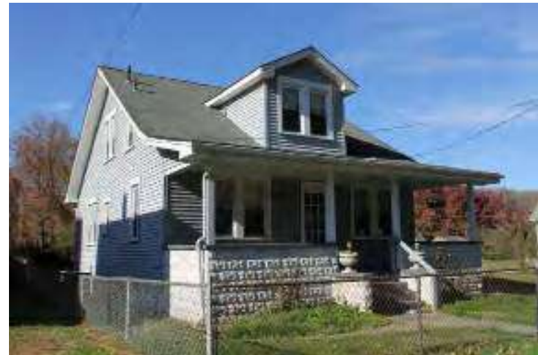
Photograph 276: 355 Glassboro Road, Woodbury Heights Borough.
