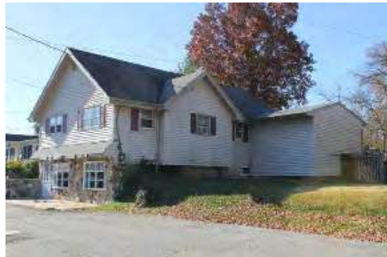
Photograph 256: 609 Glassboro Road, Woodbury City.
