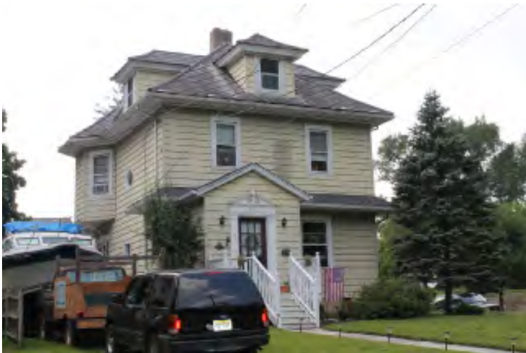
Photograph 279: 871 W. Jersey Avenue, Woodbury Heights Borough.
