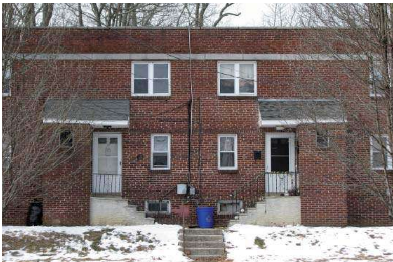
Photograph 75: S. Evergreen Avenue and S. Woodland Avenue Rowhouses, Woodbury City. Representative view of 67 S. Evergreen Avenue.
