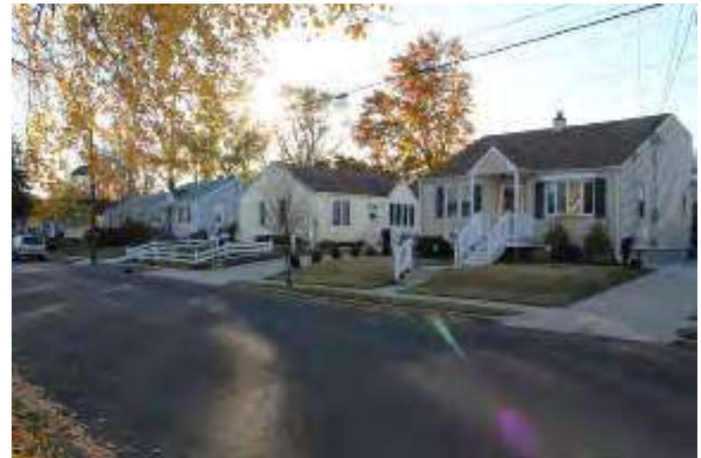
Photograph 268: Washington and Evergreen Avenues Grouping, Woodbury City. View looking southwest along Washington Avenue within the grouping.
