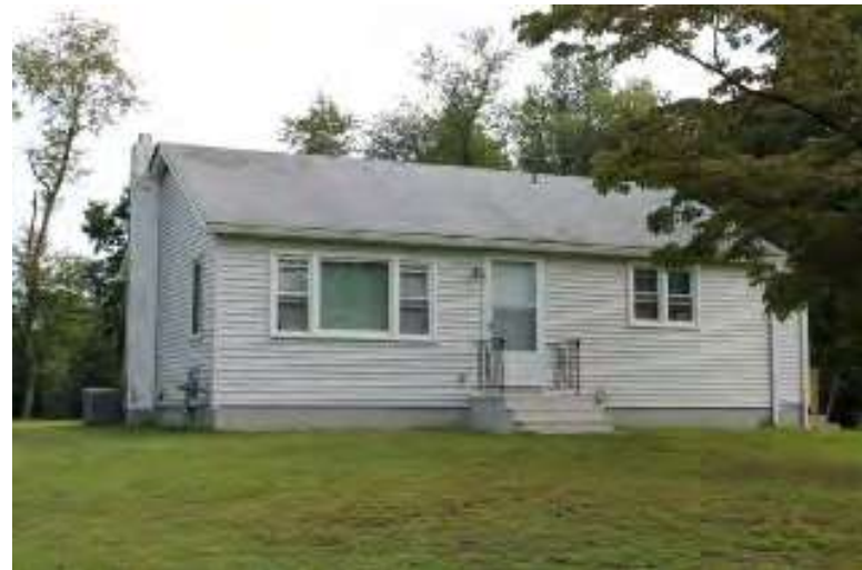
Photograph 172: Tylers Mill Road (north-side, west of railroad), Mantua Township.
