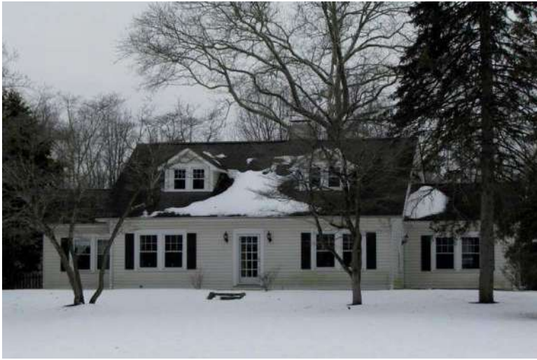
Photograph 49: 816 Main Street, Mantua Township.
