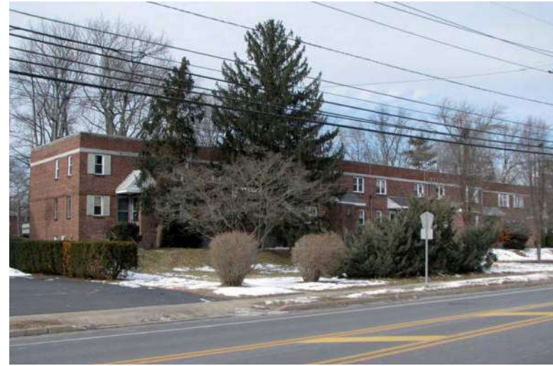
Photograph 74: S. Evergreen Avenue and S. Woodland Avenue Rowhouses, Woodbury City. Representative view of 57-73 S. Evergreen Avenue.
