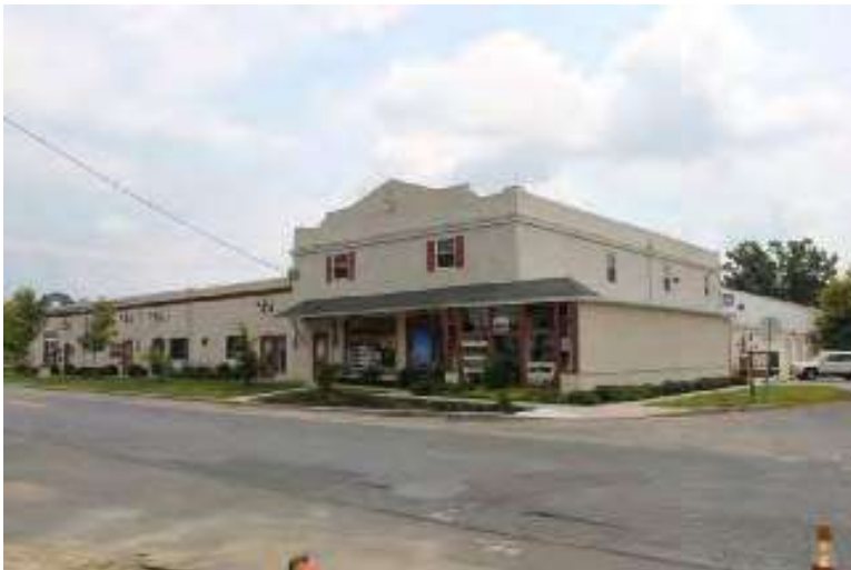
Photograph 163: 195 Center Street, Sewell, Mantua Township.
