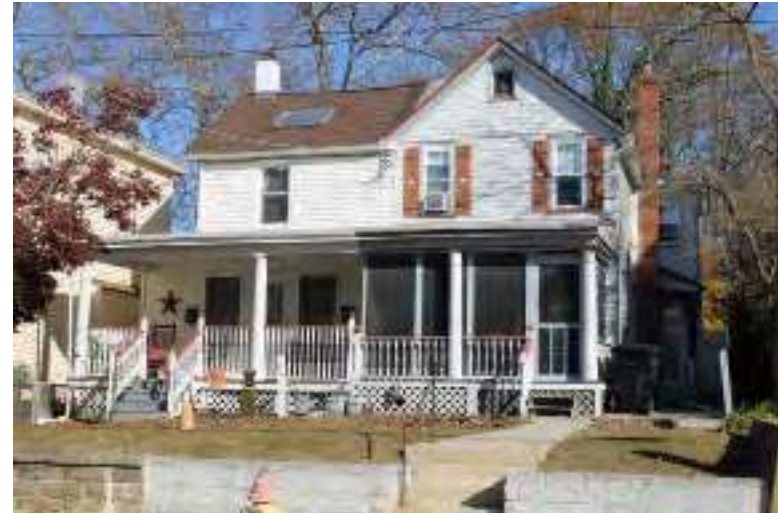
Photograph 182: 129-131 W. Jersey Avenue, Pitman Borough.
