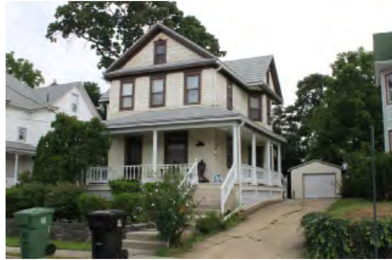
Photograph 198: Simpson Avenue Residential Streetscape, Pitman Borough. View looking northeast to 41 Simpson Avenue.
