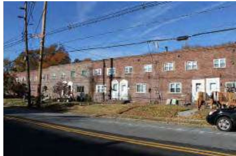
Photograph 240: Broadway Rowhouses (Oak Avenue to Cedar Avenue), Westville Borough.
