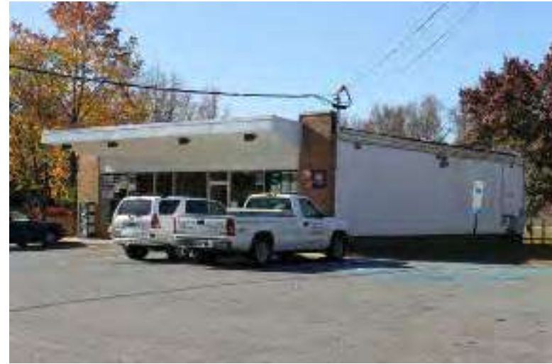
Photograph 274: 319 Glassboro Road, Woodbury Heights Borough.
