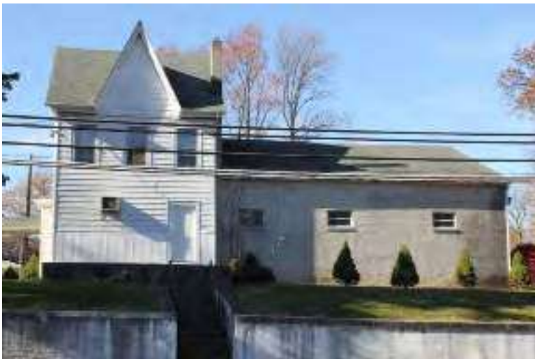
Photograph 255: 569 Glassboro Road, Woodbury City.
