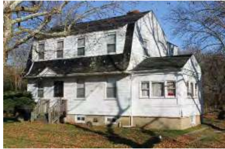
Photograph 94: 129 Buck Road, Elk Township.
