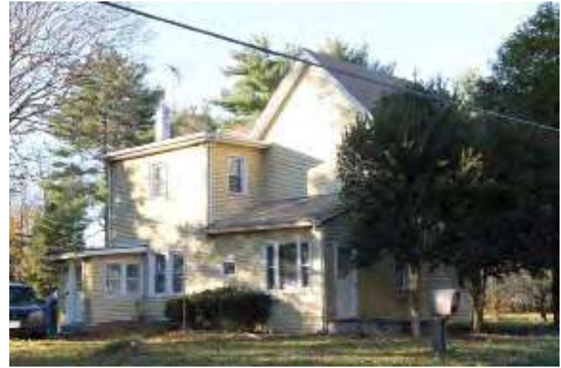
Photograph 90: 116 Buck Road, Elk Township.
