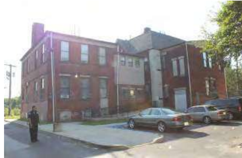
Photograph 6: Jesse Starr School (NR eligible), 823 Pine Street, Camden City. View of north (rear) and west (side) elevations, showing alterations.
