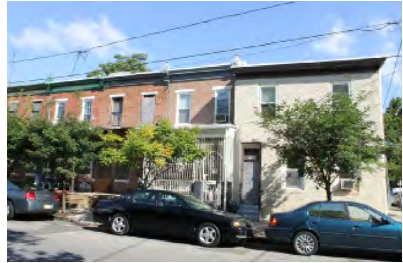
Photograph 78: Walnut Street Rowhouses (north-side, west of S. 9th Street), Camden City.
