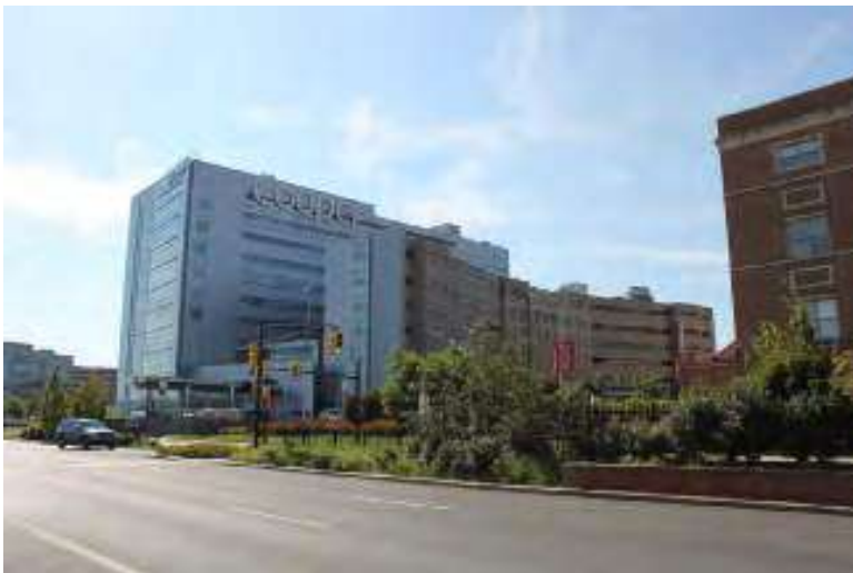
Photograph 47: 1 Cooper Plaza (Cooper University Hospital), Camden City. Extensive additions have compromised the resource's integrity.
