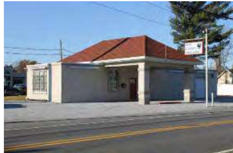
Photograph 84: 1250 Broadway, Deptford Township.
