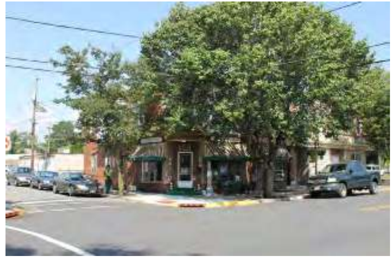
Photograph 138: Monmouth Street Commercial Row, Gloucester City.
