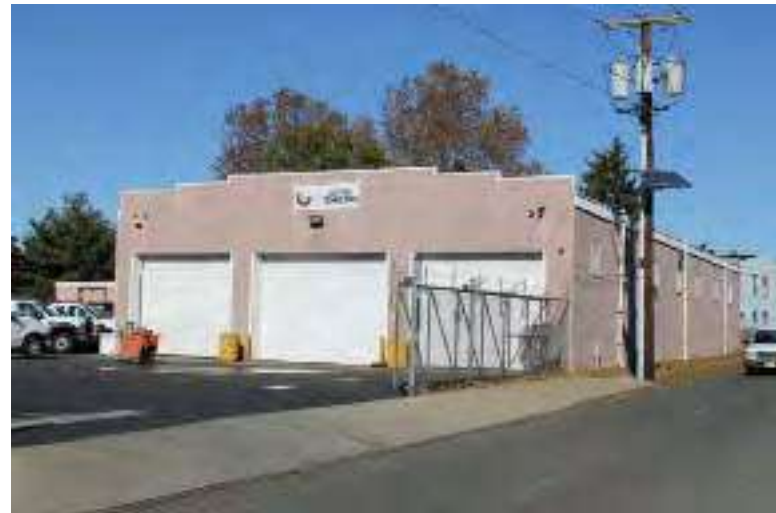
Photograph 152: 101 Washington Avenue, Gloucester City.
