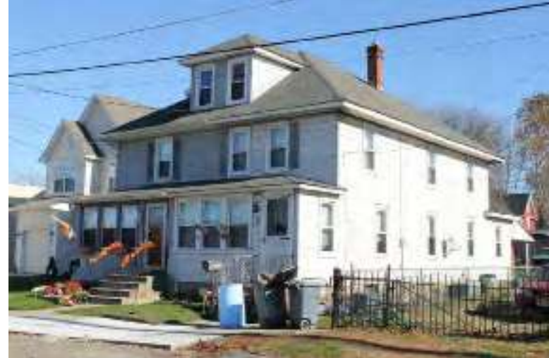
Photograph 28: 3-5 Railroad Lane, Brooklawn Borough.
