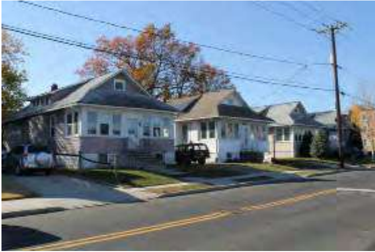
Photograph 125: Essex Street Streetscape (south-side, east of Railroad Avenue), Gloucester City.
