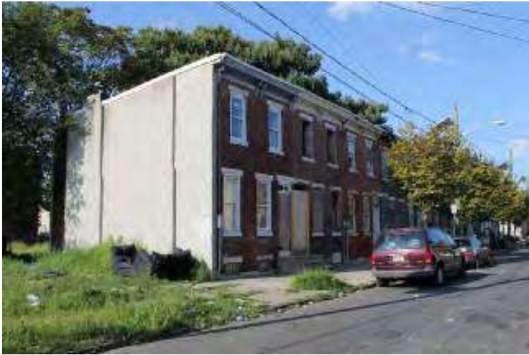
Photograph 61: Line Street Rowhouses (south-side, west of S. 9th Street), Camden City.
