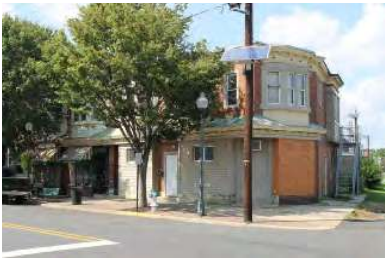
Photograph 139: Monmouth Street Commercial Row, Gloucester City.
