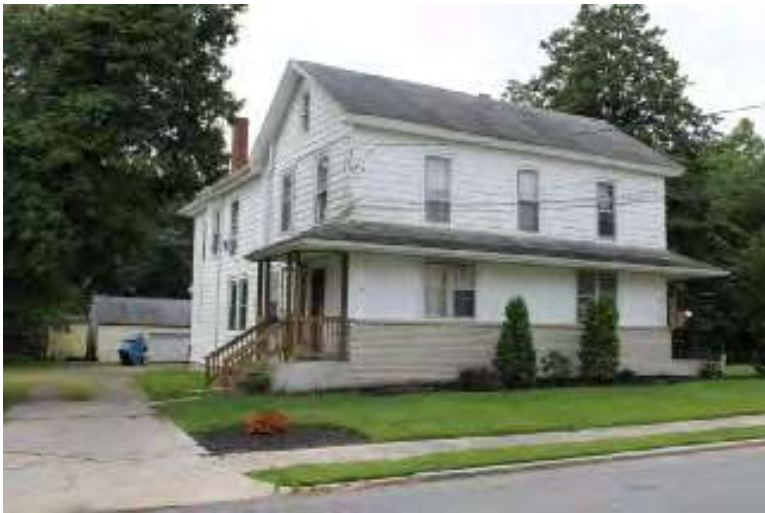
Photograph 115: 34 Zane Street, Glassboro Borough.
