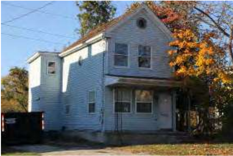
Photograph 81: 1190 Broadway, Deptford Township.
