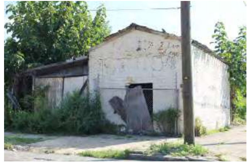
Photograph 74: 801 Sycamore Street, Camden City.
