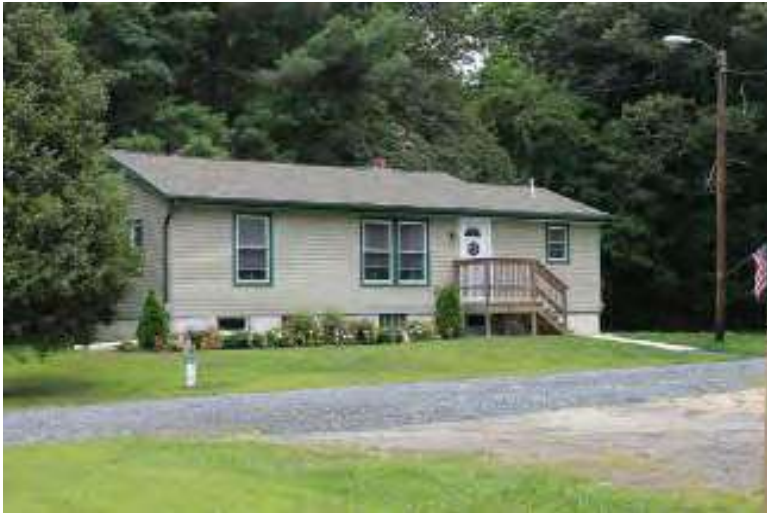
Photograph 93: 121 Buck Road, Elk Township.
