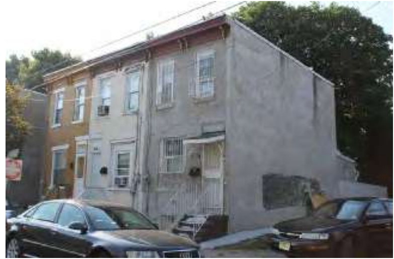
Photograph 62: Line Street Rowhouses (south-side, west of S. 9th Street), Camden City.
