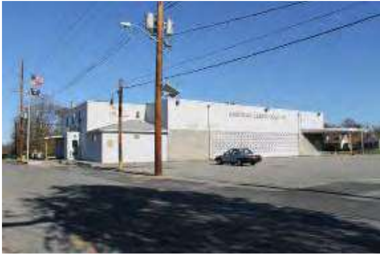
Photograph 29: 11 Railroad Lane (American Legion Post 72), Brooklawn Borough.
