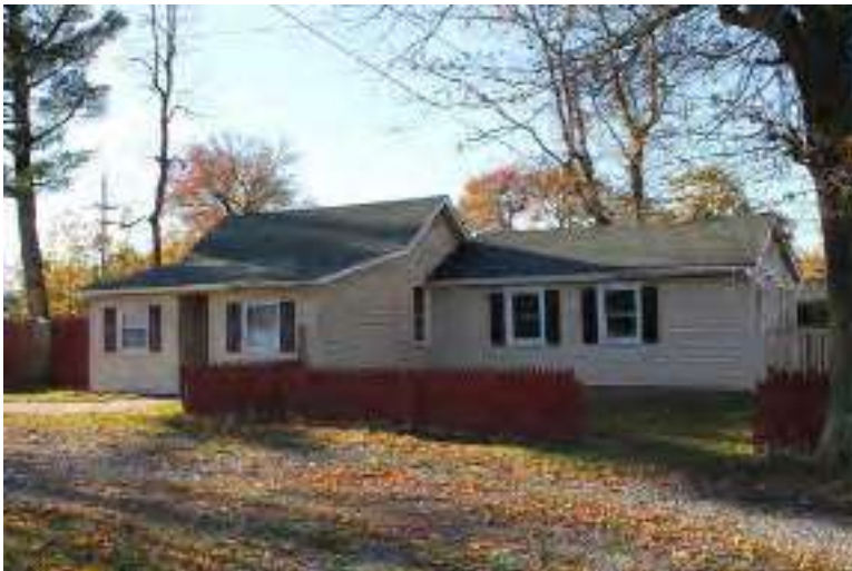
Photograph 83: 1240 Broadway, Deptford Township.
