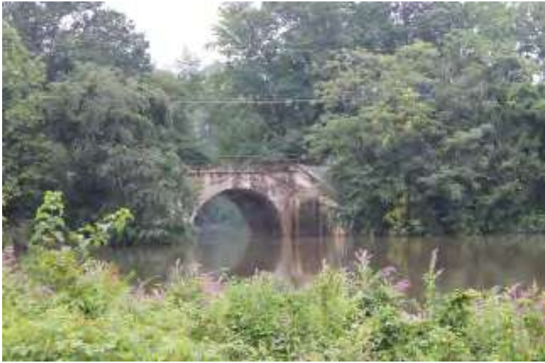
Photograph 25: West Jersey & Seashore Railroad/Pennsylvania Reading Seashore Lines, bridge over Woodbury Creek, Woodbury Township.
