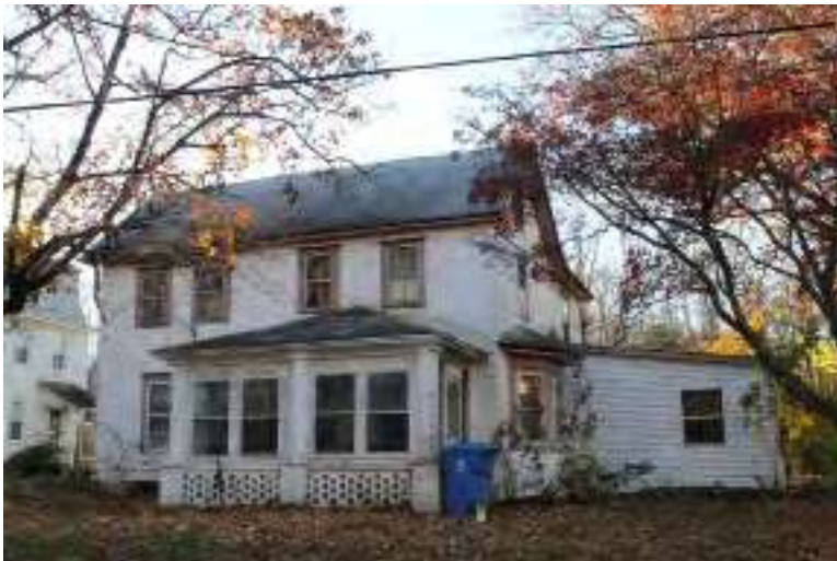
Photograph 91: 118 Buck Road, Elk Township.
