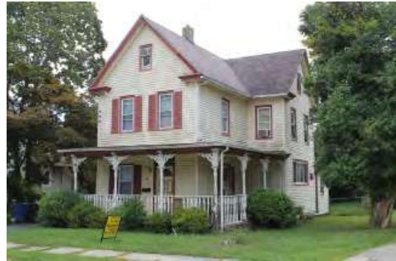
Photograph 114: 32 Zane Street, Glassboro Borough.
