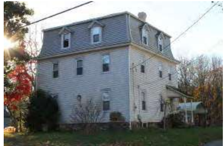
Photograph 92: 120 Buck Road, Elk Township.
