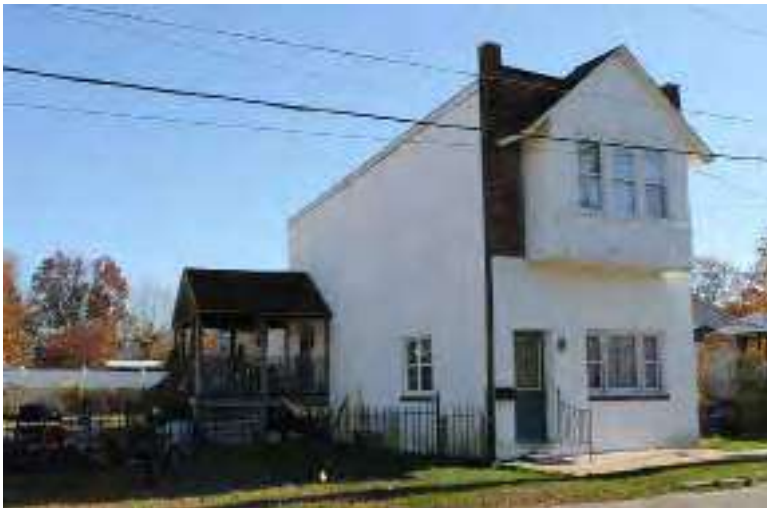
Photograph 27: 1 Railroad Lane, Brooklawn Borough.
