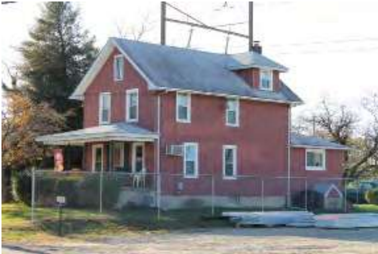
Photograph 79: 1180 Broadway, Deptford Township.
