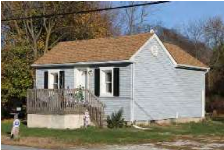
Photograph 95: 151 Buck Road, Elk Township.
