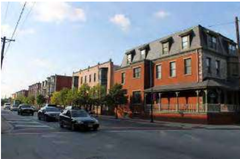
Photograph 3: Cooper Plaza Historic District (NR eligible; local certified district), Camden City. View looking northeast along Haddon Avenue.
