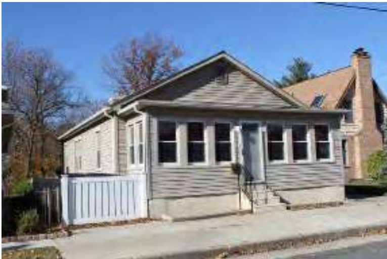
Photograph 151: 7 S. Stites Avenue, Gloucester City.
