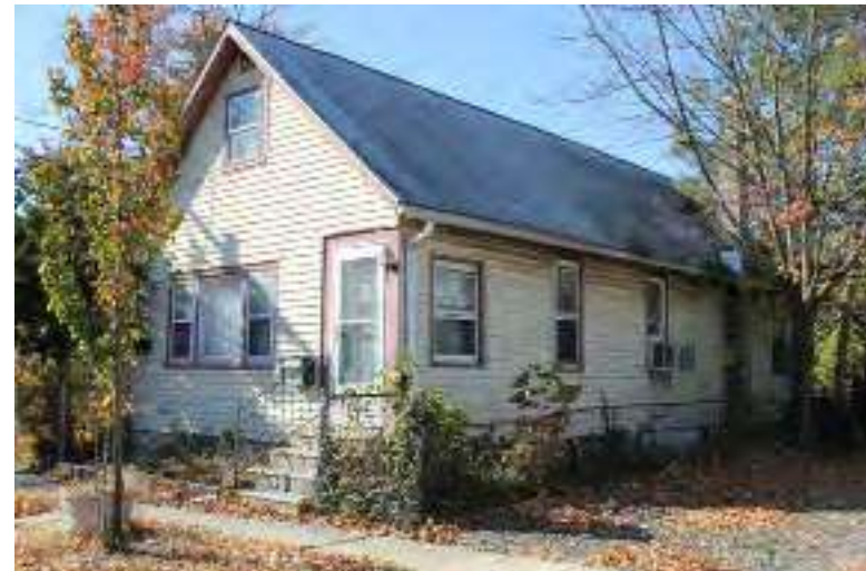
Photograph 148: 1 S. Stites Avenue, Gloucester City.
