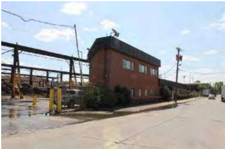
Photograph 31: 1500 S. 6th Street (Camden Iron and Metal), Camden City. View looking south. All that remains from the pre-1965 era are two small brick office buildings.
