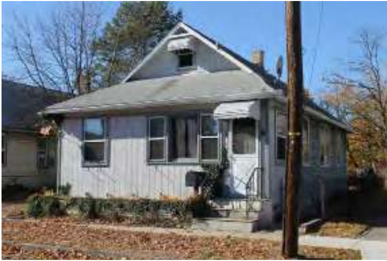
Photograph 149: 3 S. Stites Avenue, Gloucester City.
