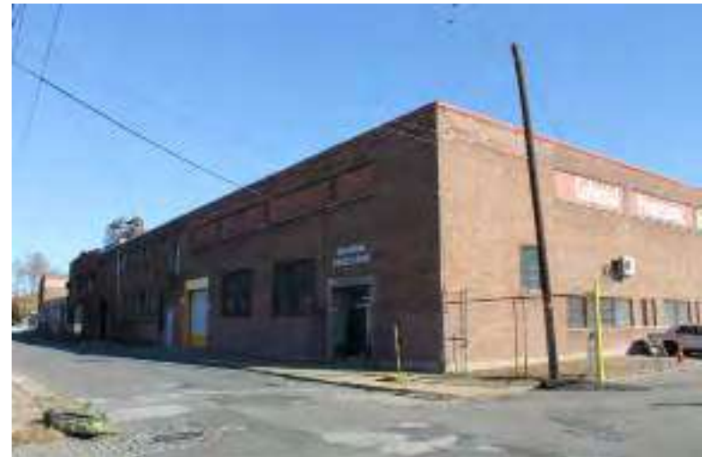
Photograph 32: 6th Street Streetscape (east side, Viola Street to Jefferson Street), Camden City.
