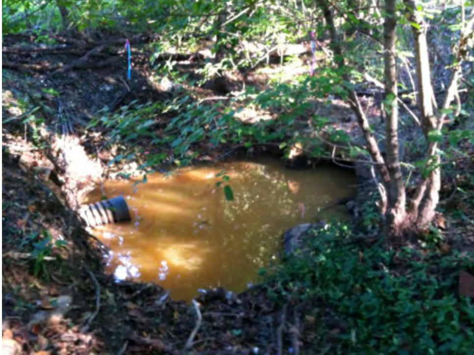
Photo 15: Drainage ditch WWH-B looking west (September 2013).
