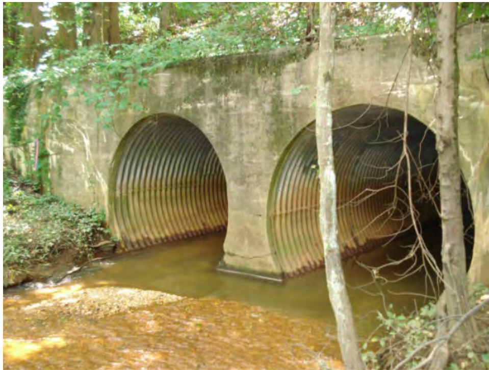
Photo 28: Wetland WWN-B looking west at culvert crossing carrying Monongahela Brook (August 2013).
