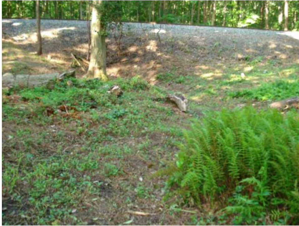
Photo 29: Drainage ditch WMT-E at Surrey Road, looking southwest (August 2013).
